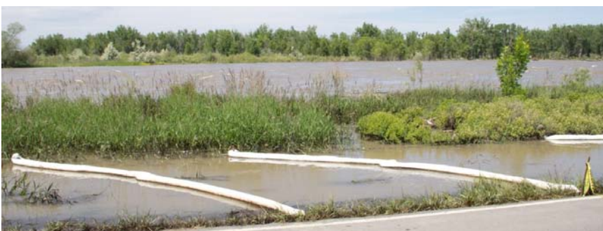
Booms along the Yellowstone River to capture spilled oil
