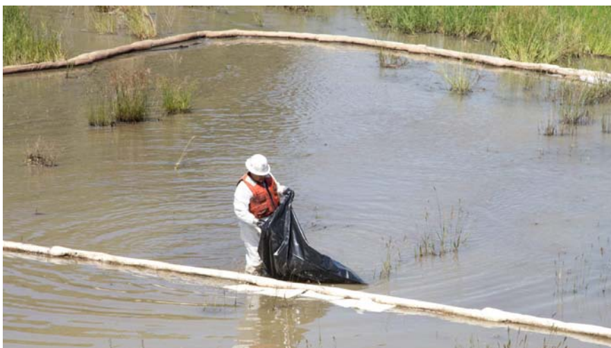
Collecting oil soiled pads along a boom in the Yellowstone River
