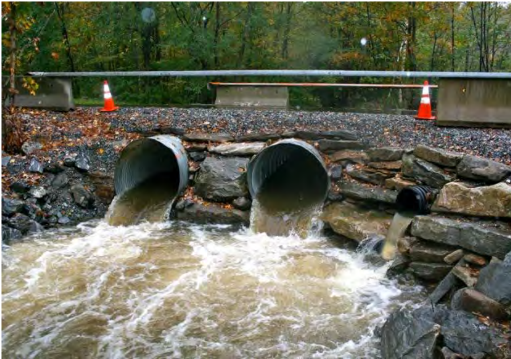
Walker Brook project, Becket, MA
