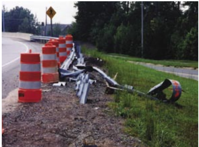
Figure 2. Photograph. Information on the cost of maintaining guardrails mangled by crashes can be identified through highway management systems.
