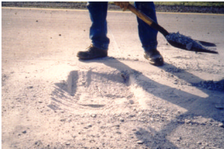
Figure 7b. Milled patch with rounded edges.
