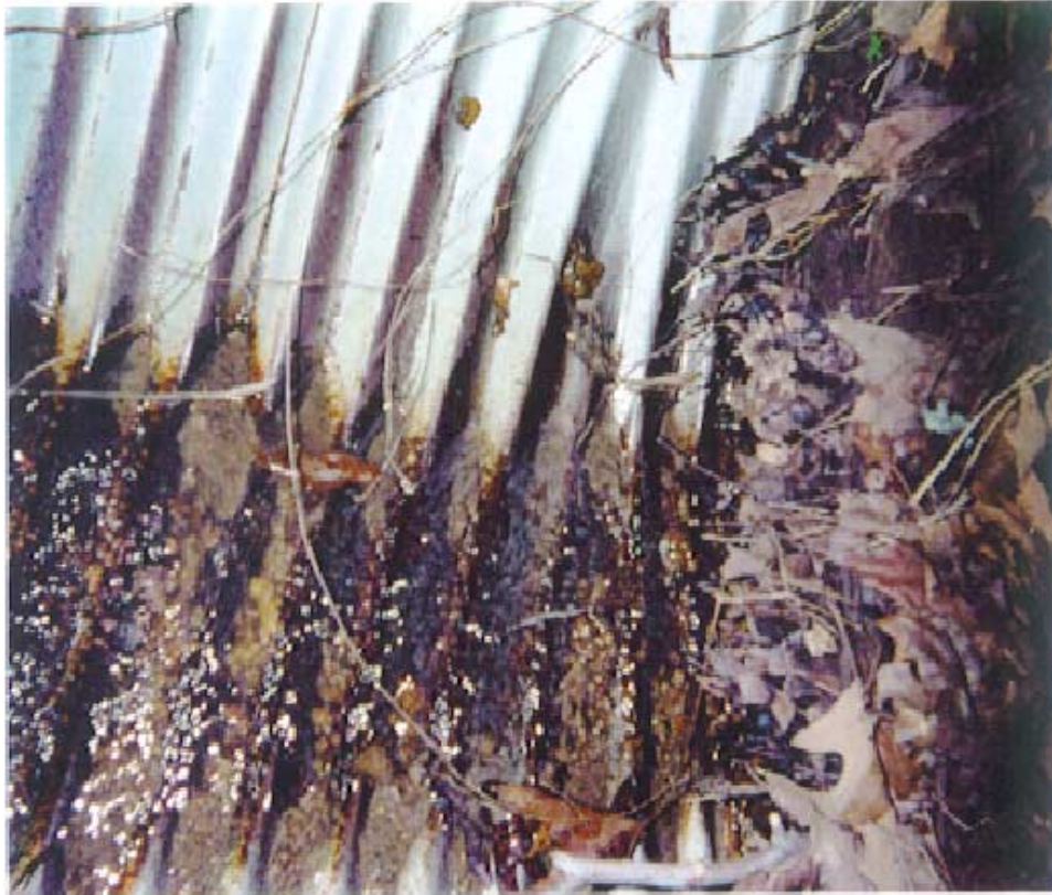
Figure 17. Inlet of the pipe at 309.4.
