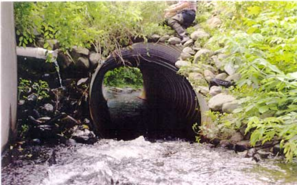
Figure 7. Culvert at Dexter, Maine, experiencing high-velocity flow.
