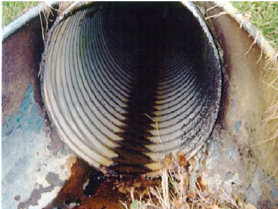
Figure 16. Inlet of the pipe at 309.5.
