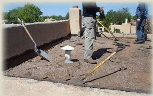
Roof: Before (After, shown above)
