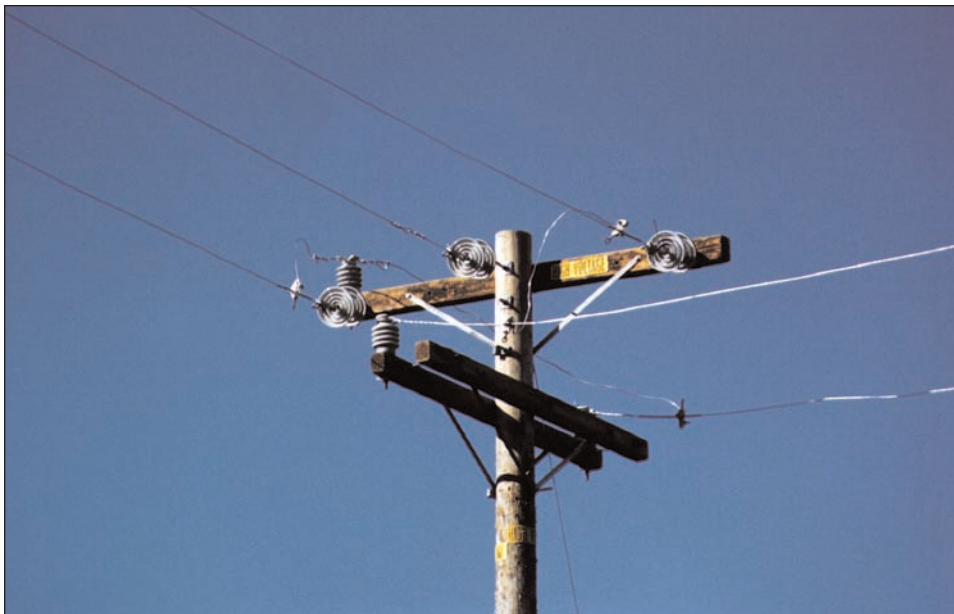
Figure 4-6 Crossarm Deadend Corner (Line and Buck)
