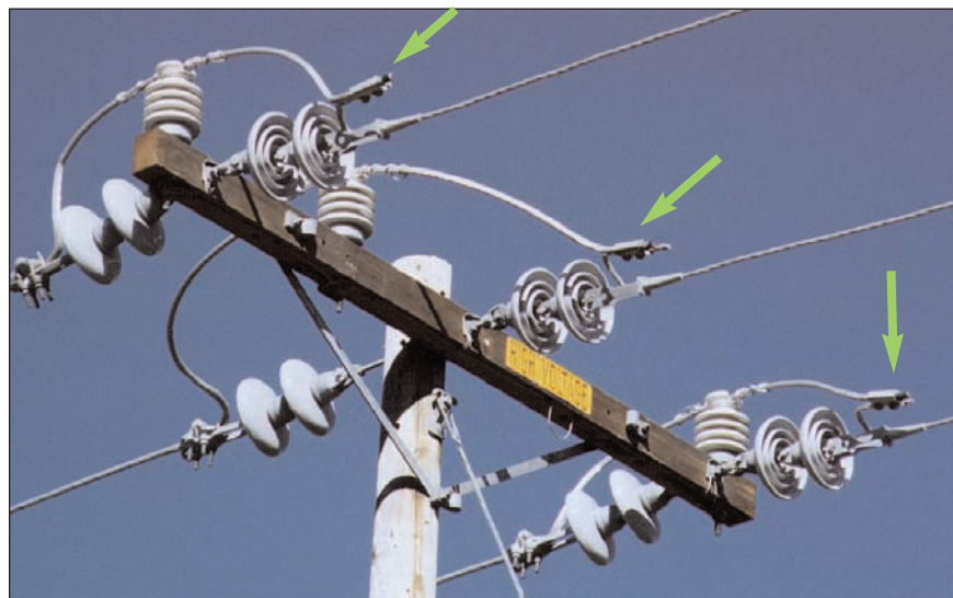
Figure 3-48 Parallel Groove Connectors on Jumpers
