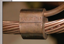
Figure 3-63 Copper Compression Connector, (compressed)
