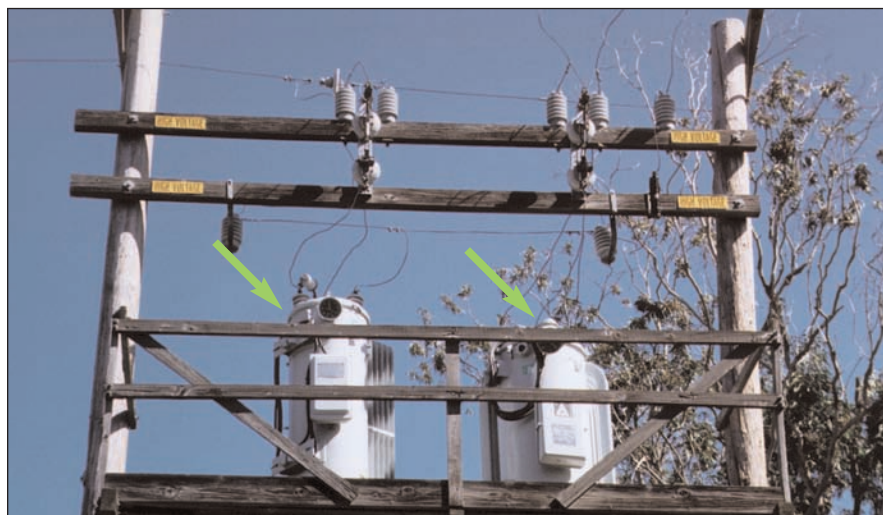
Figure 3-41 Voltage Regulator
