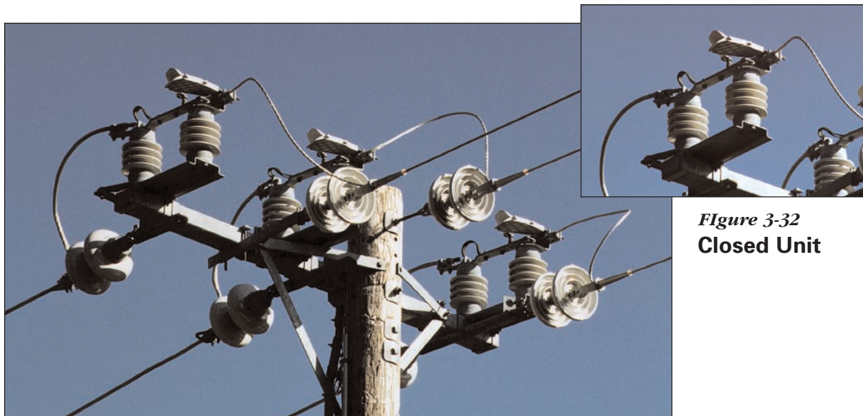
Figure 3-31 S&C Omni-Ruptor Switch, Tangent Construction (closed position)
