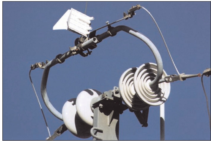
Figure 3-20 600 Amp KPF Air Switch, Triangular Construction (closed position)
