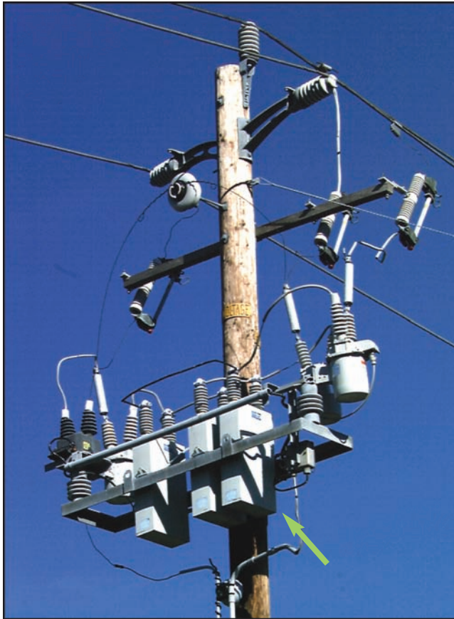
Figure 3-42 Capacitor Bank
