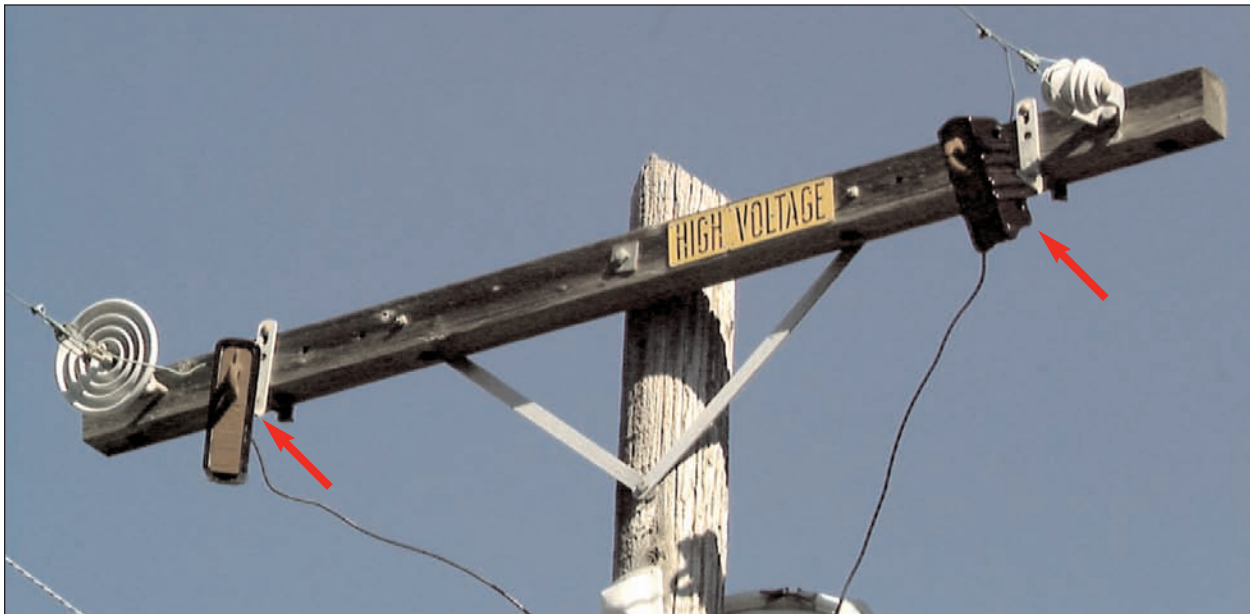
Figure 2-10 Arm Mounted Enclosed Cutout with Universal Fuses
