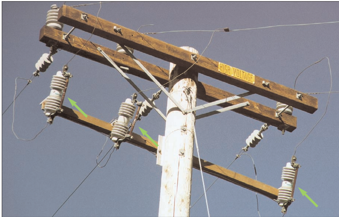
Figure 3-10 Arm Mounted Cutout with Liquid Filled Fuse
