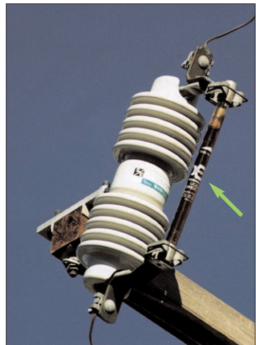
Figure 3-11 Liquid Filled Fuse
