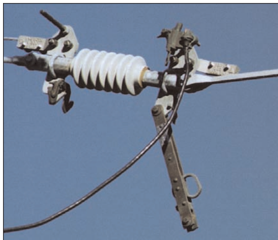
Figure 2-17 In-Line Disconnect (open position)
