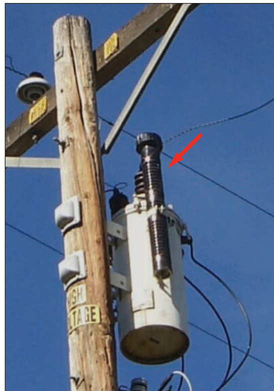
Figure 2-28 Lightning Arrester
