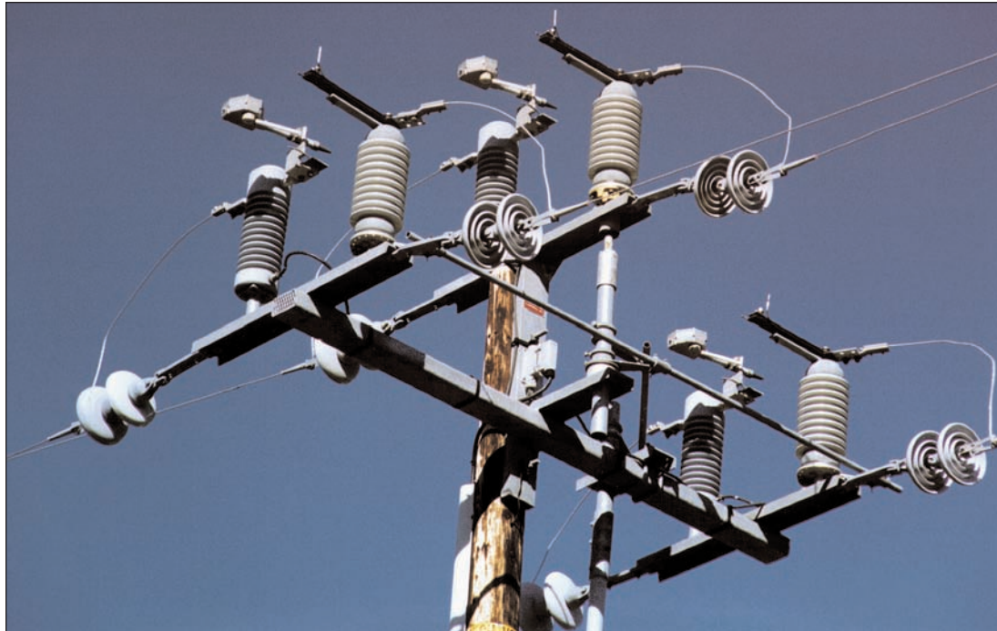
Figure 3-30 S&C Omni-Ruptor Switch, Triangular Construction (open position)
