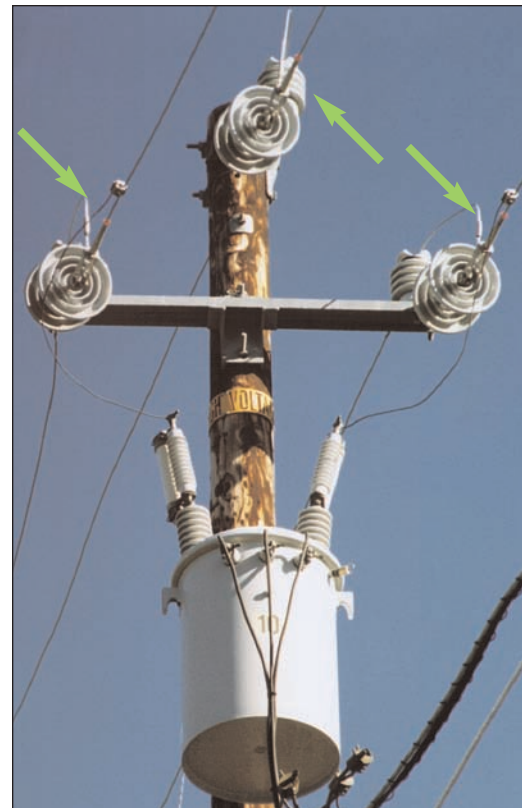
Figure 3-69 Automatic Deadends Attached to Pole and Crossarm
