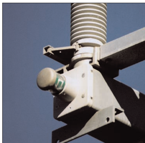
Figure 3-34 Open Position Indicator Green Letter "O" visible
