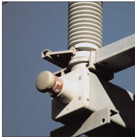
Figure 3-35 Closed Position Indicator Red
