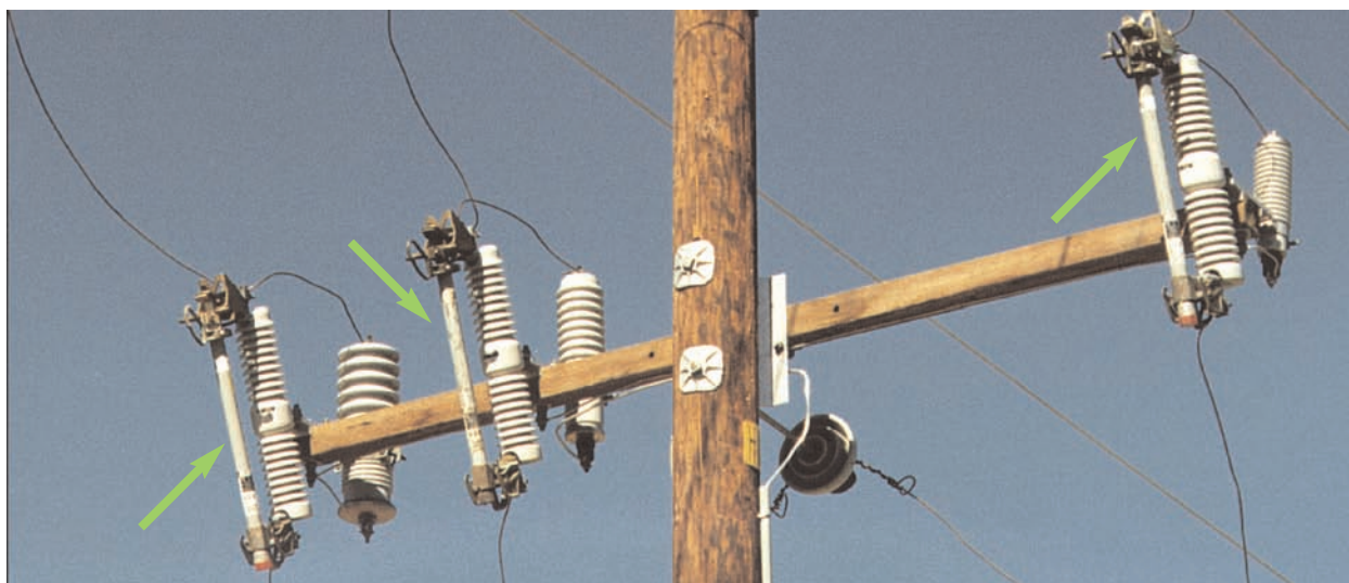
Figure 3-16 Arm Mounted Cutout with SMU-20 Fuses
