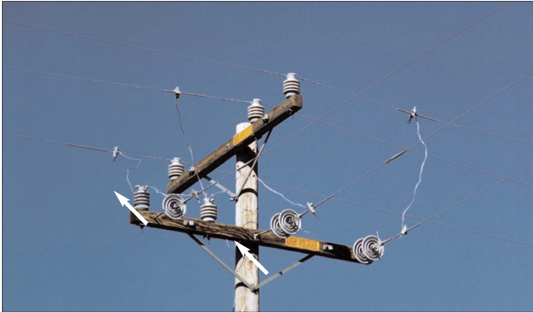
Figure 4-5 Tangent Crossarm with Deadend Tap (T-Tap)
