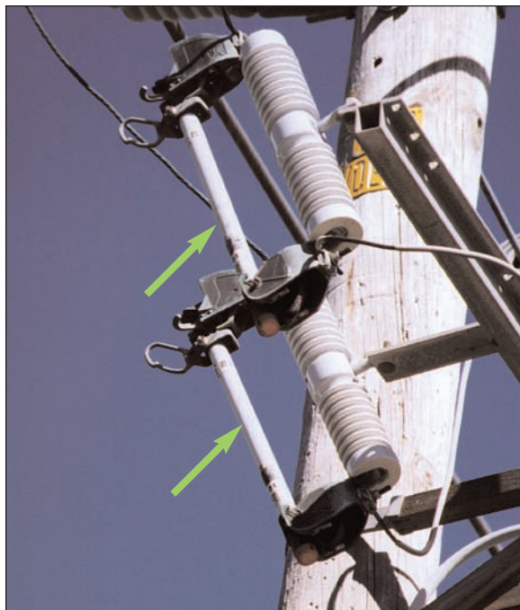
Figure 3-14 Arm Mounted Cutout with SMU-20 Fuses
