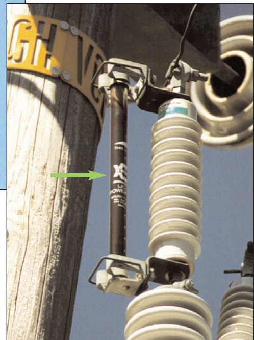
Figure 3-13 Liquid Filled Fuse
