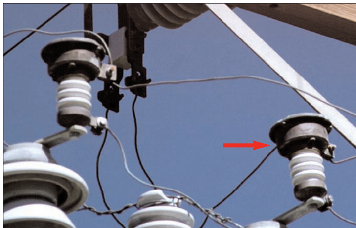
Figure 2-22 Lightning Arrester
