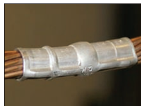
Figure 3-72 Compressed Line Splice
