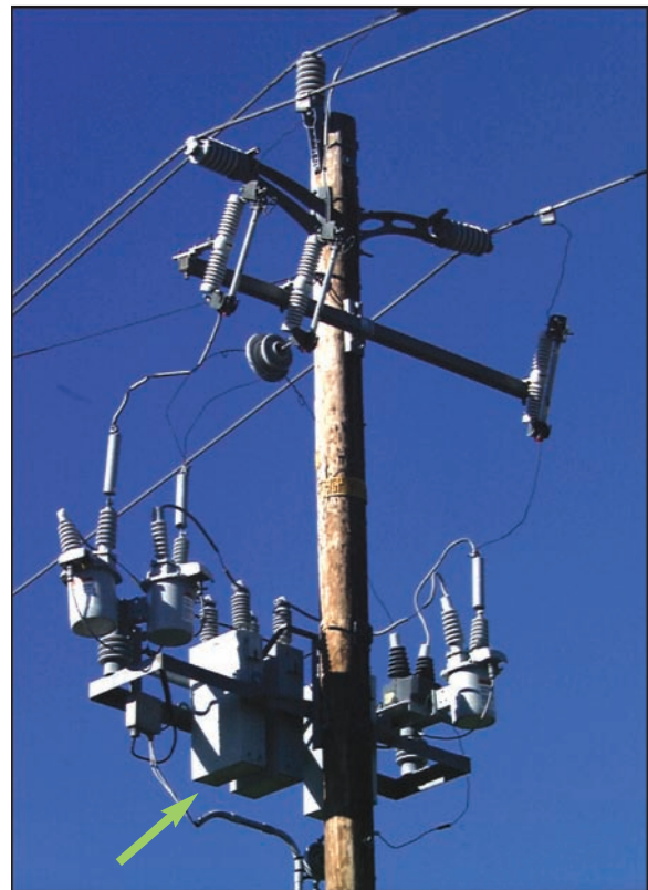
Figure 3-43 Capacitor Unit
