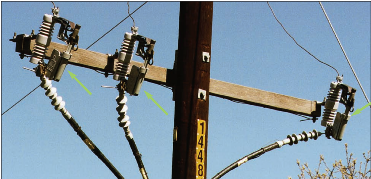
Figure 3-17 Arm Mounted Cutout with S&C Fault Tamer Fuse
