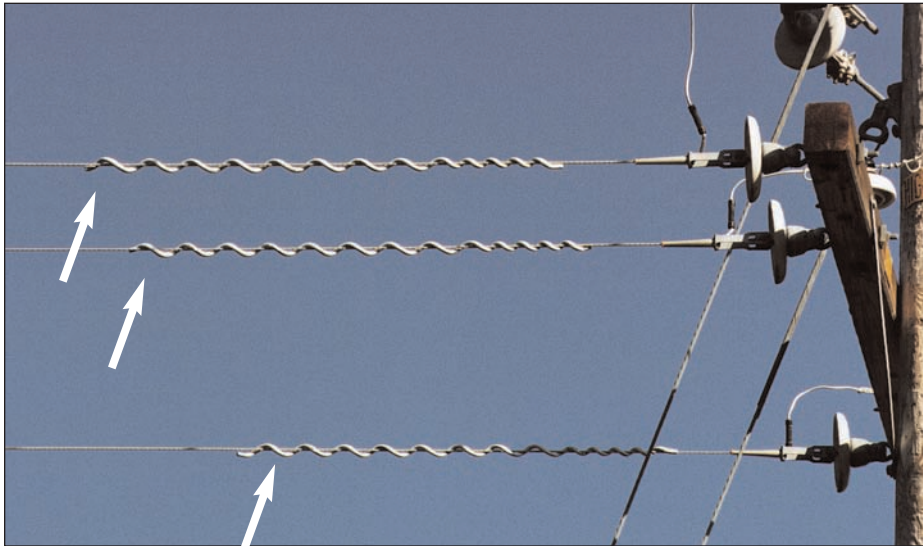
Figure 4-13 Vibration Damper
