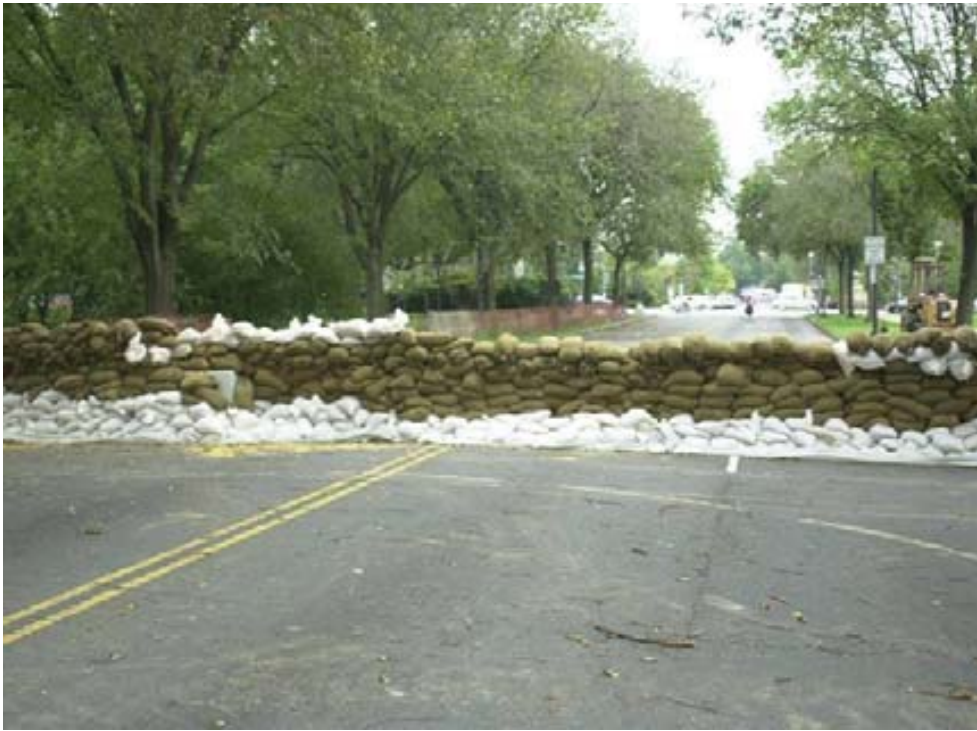
Sandbag closure on 17th Street, NW
