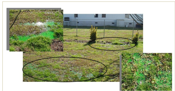
Figure 1. Surfacing fluorescein dye around leach lines and in ditches indicate the failing of septic systems.
