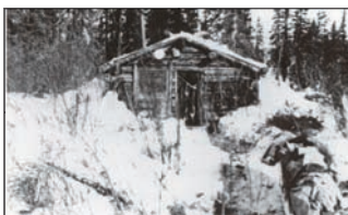
4-Mile Trapper Cabin
