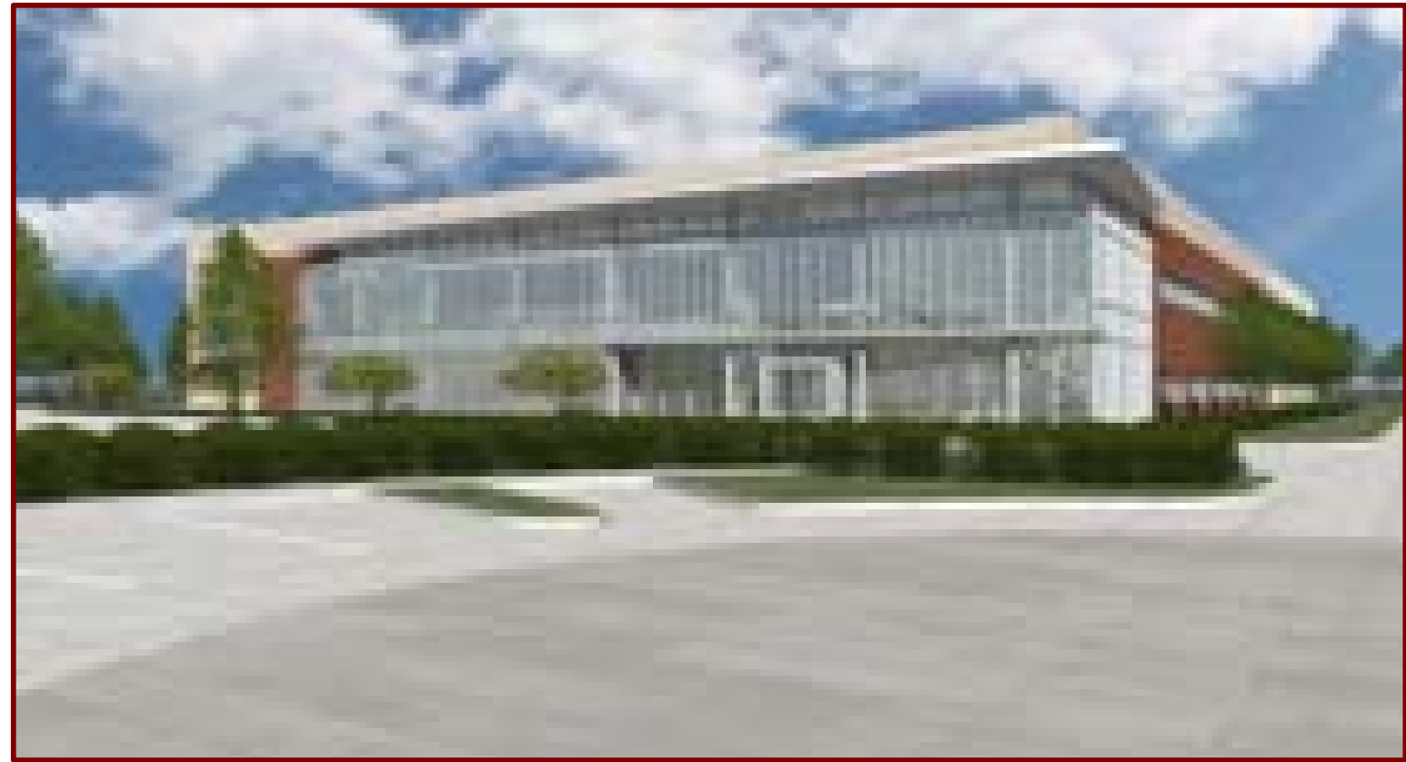
Pandemic Influenza Facility (PIF) *NEW CONSTRUCTION*
