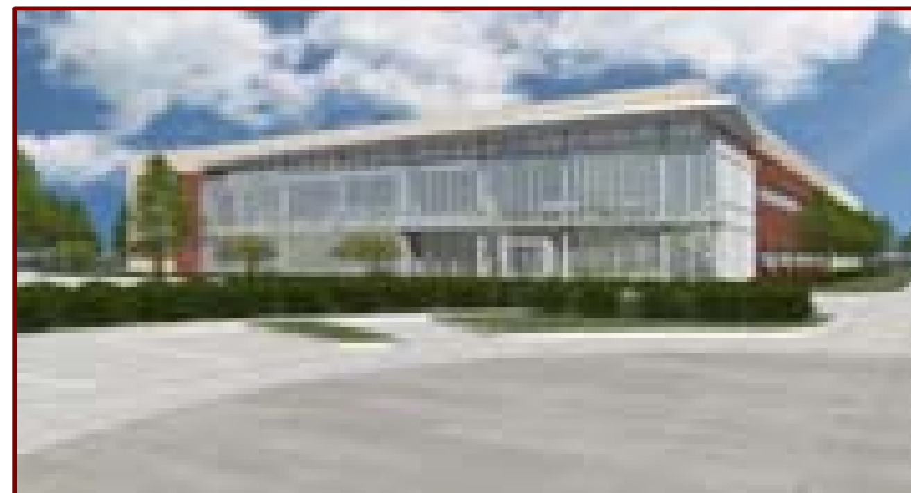
LONZA Facility *NEW CONSTRUCTION*
