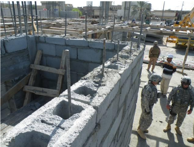
Site Photo 8. CMU vertical reinforcing
