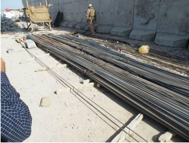
Site Photo 5. Stockpiled reinforcing steel
