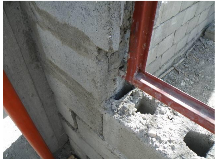
Site Photo 12. CMU wall window frame
