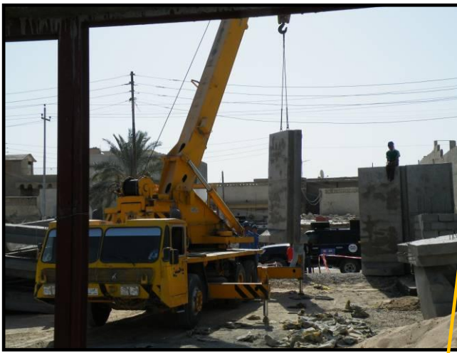
Site Photo 3. T-wall installation
