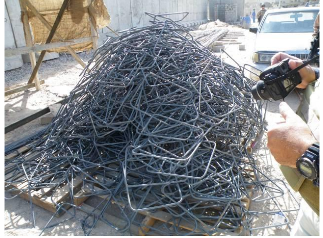
Site Photo 6. Fabricated reinforcing steel
