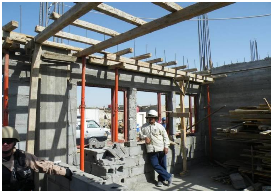
Site Photo 7. Reinforced concrete beam formwork
