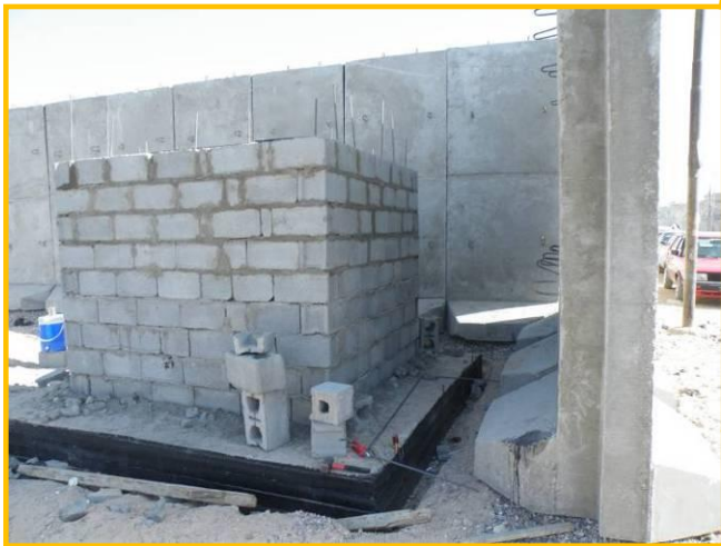
Site Photo 4. 4 Guard towers
