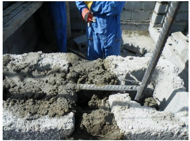
Site Photo 9. CMU horizontal reinforcing
