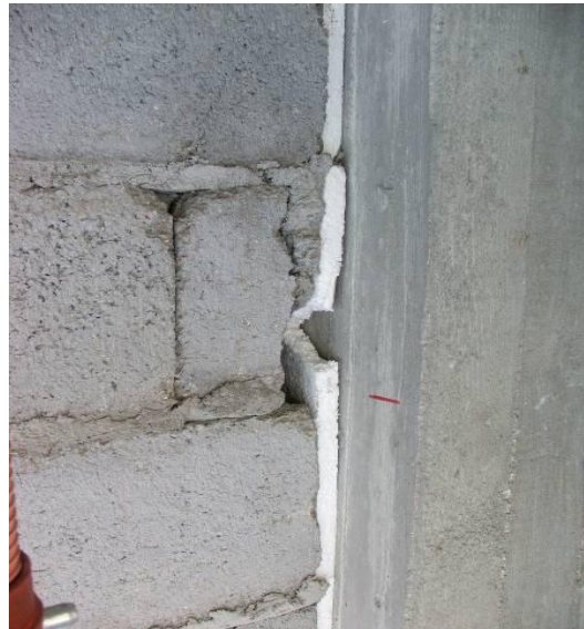
Site Photo 10. Expansion joint between infill and frame
