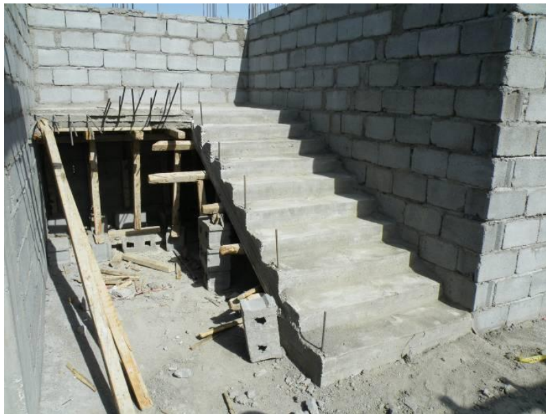
Site Photo 13. Reinforced concrete stairs
