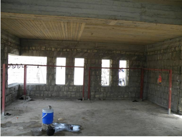
Site Photo 12. Interior view of winter hall
