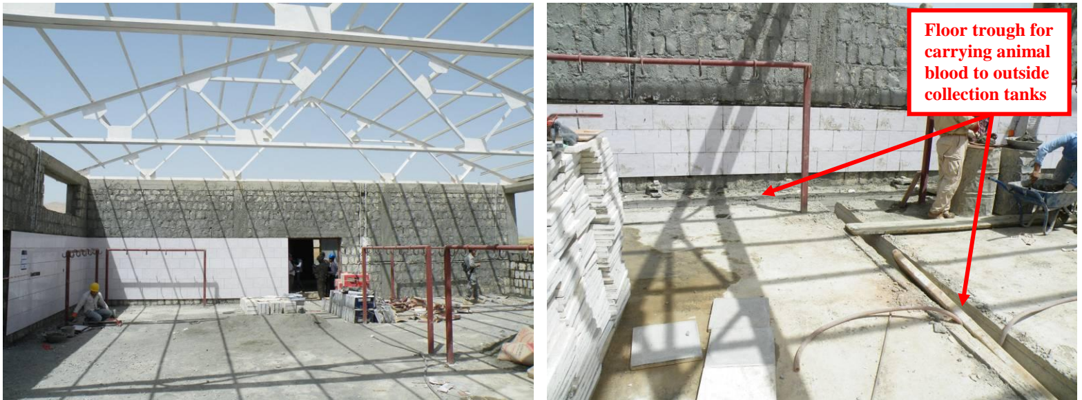
Site Photos 10 and 11. Interior views of the slaughterhouse room
