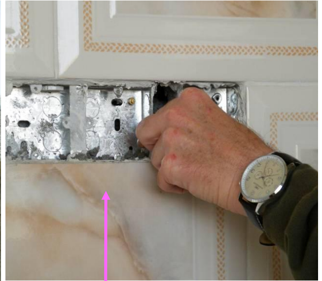
Site Photo 8. Preliminary electrical wiring
