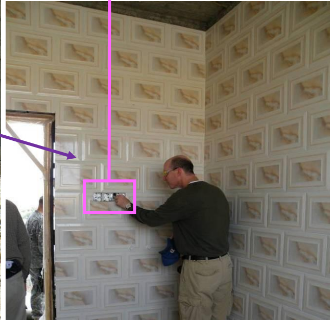
Site Photo 9. Glazed ceramic tiles on the interior walls
