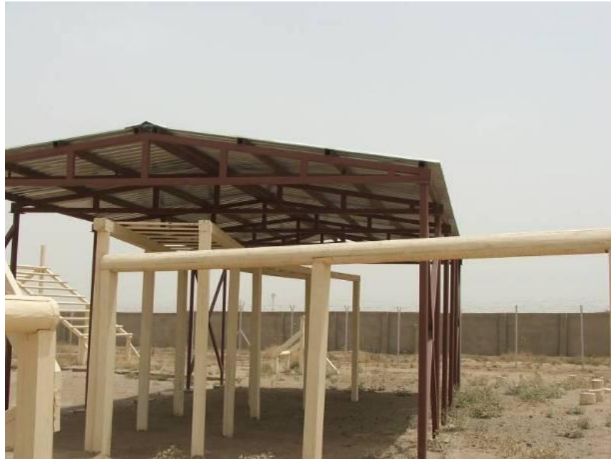
Site Photo 21. Sunshade over obstacles for combat assault course
