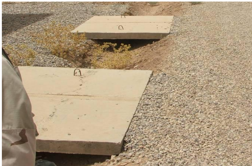
Site Photo 10. Precast concrete panel footbridge
