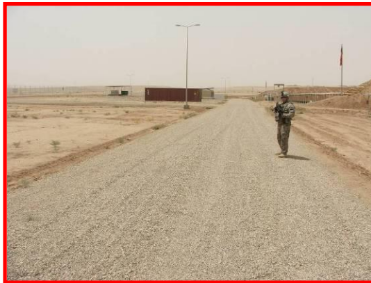
Site Photo 2. Access road
