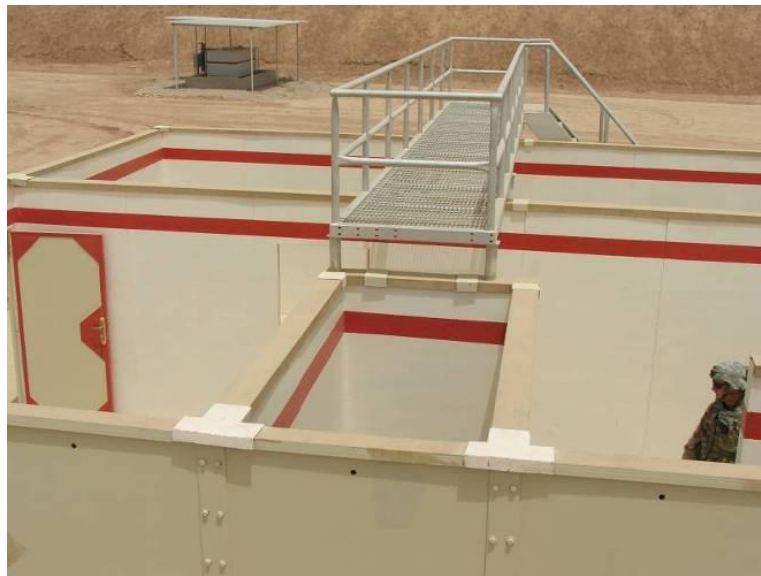
Site Photo 15. Observation platform
