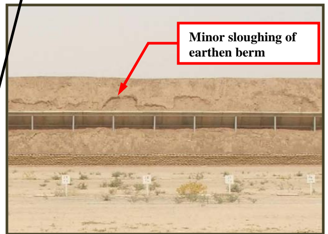
Site Photo 7. Earthen berm
