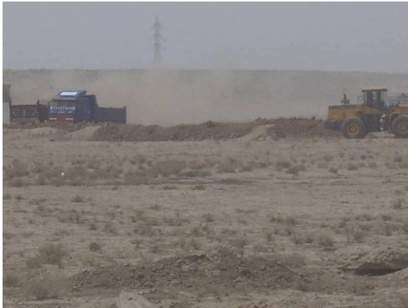
Site Photo 1. Site location prior to construction (Courtesy of USACE)
