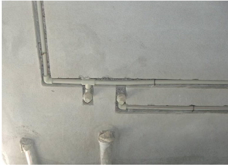
Site Photo 6. "Pilsatherm" water pipes embedded along exterior wall
