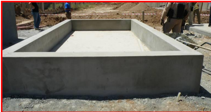
Site Photo 3. Fuel tank base
