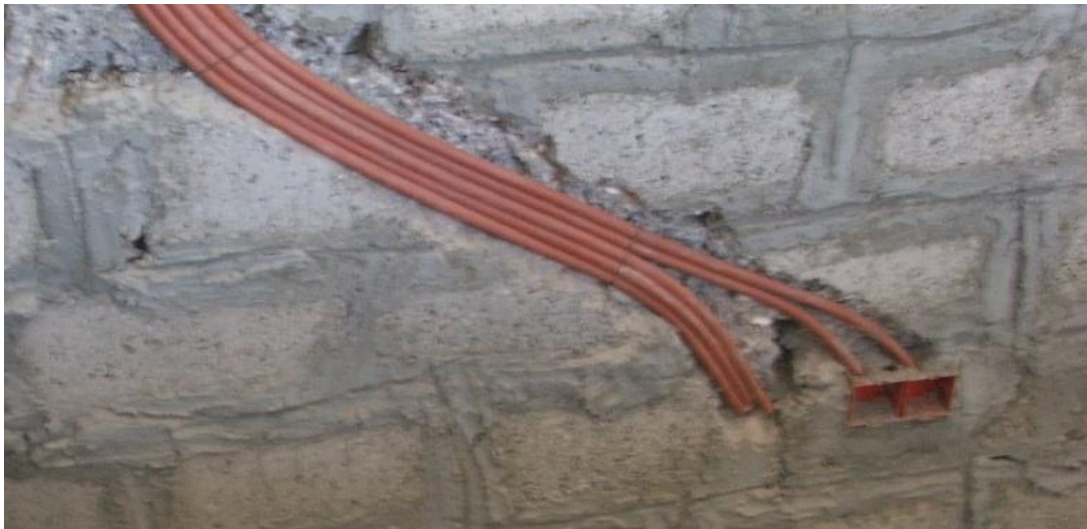
Site Photo 5. Electrical conduit embedded in interior wall
