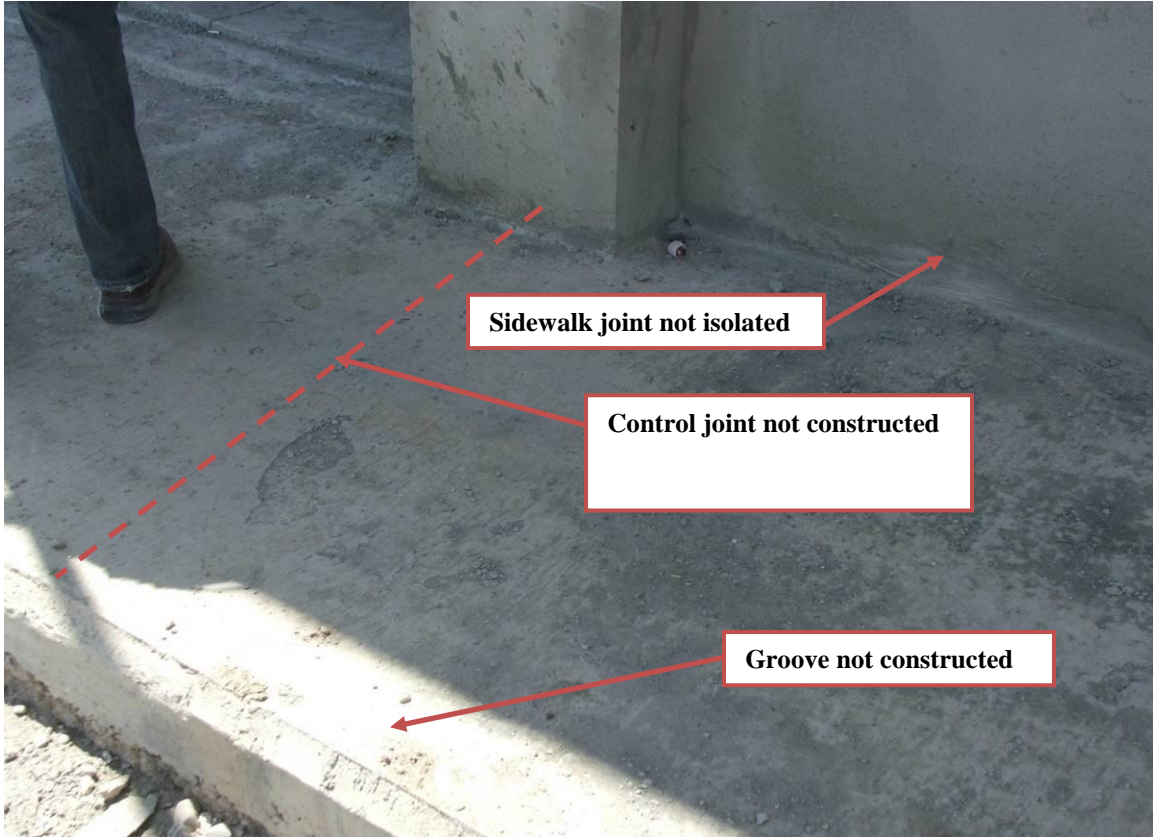
Site Photo 9. Construction of exterior sidewalk
