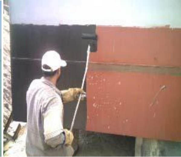
Site Photo 8. Painting with coal tar epoxy (Courtesy of GRS)
