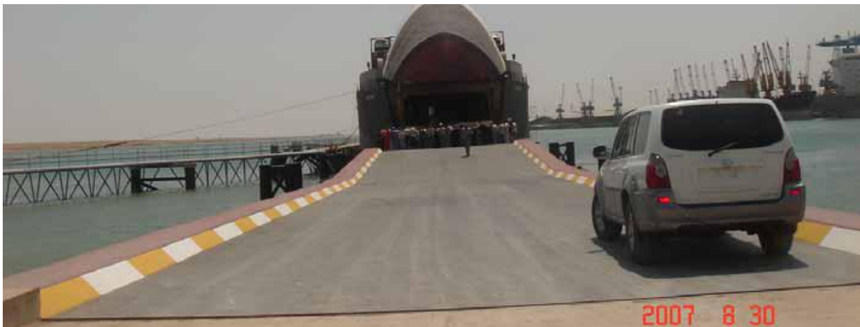
Site Photo 4. Constructed RORO Berth 22 (Courtesy of GRS)
