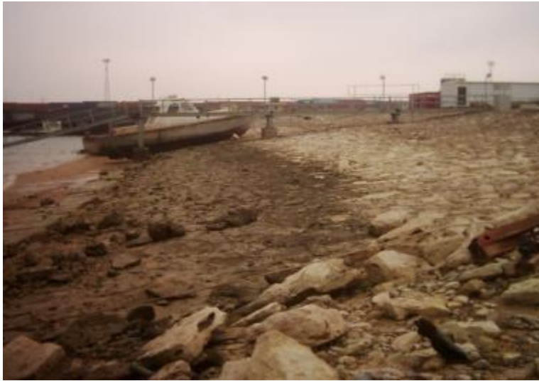
Site Photo 1. Obstructed future RORO Berth 22 site (Courtesy of GRS)
