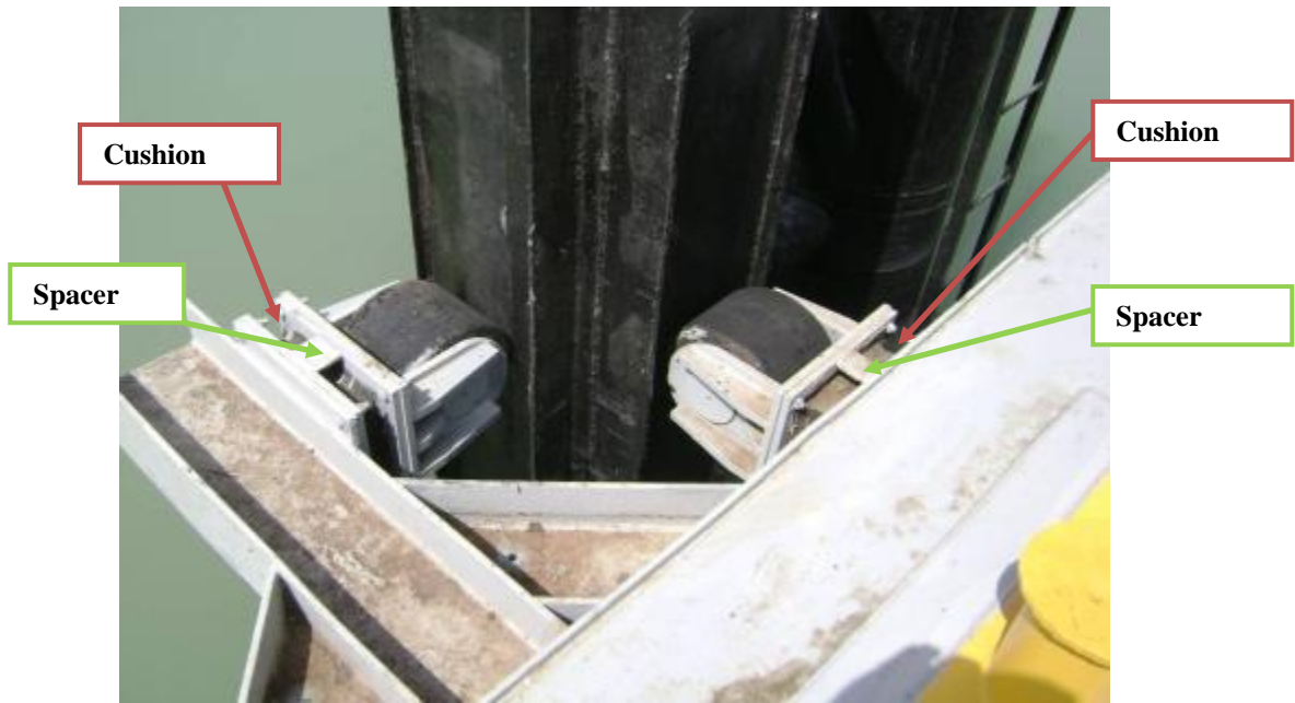
Site Photo 11. Cushion rollers with steel spacer plates (Courtesy of GRS)
