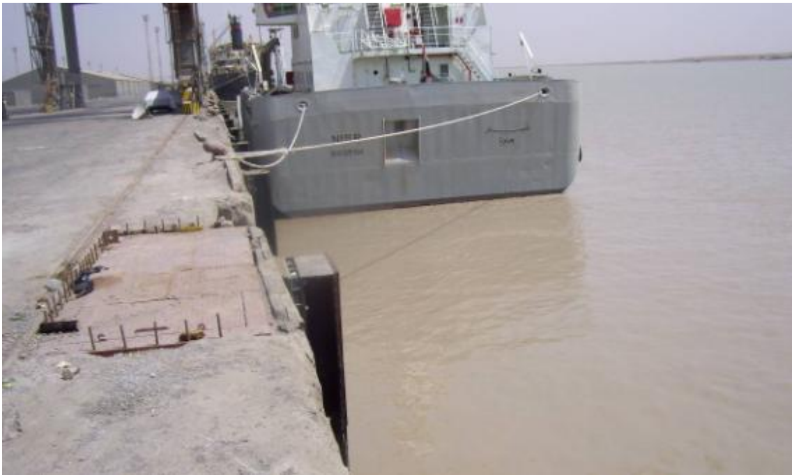
Site Photo 9. Berth 5 new jetty fenders (Courtesy of GRS)
