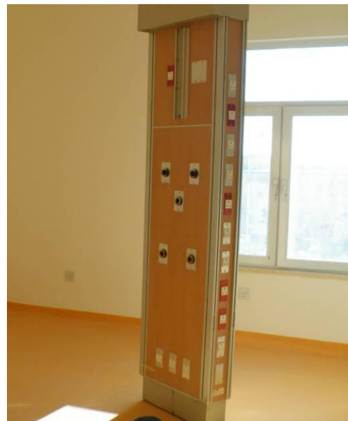
Site Photos 8 and 9. Hook-ups for medical equipment
