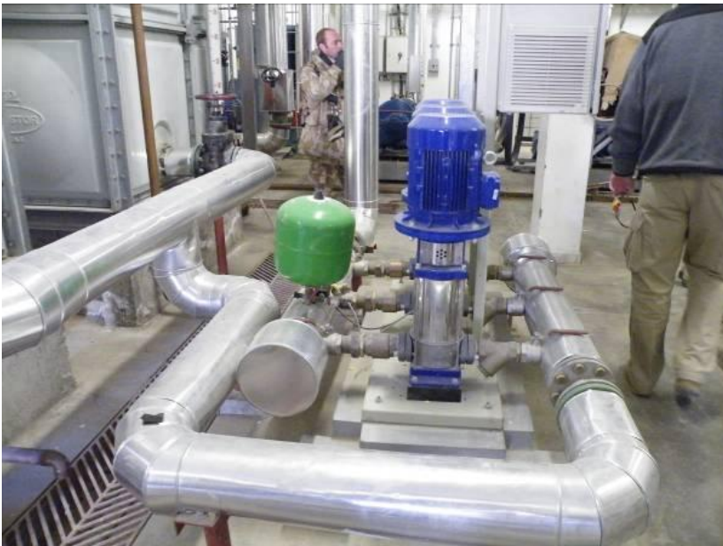
Site Photos 19 and 20. Water booster pumps and storage tanks
