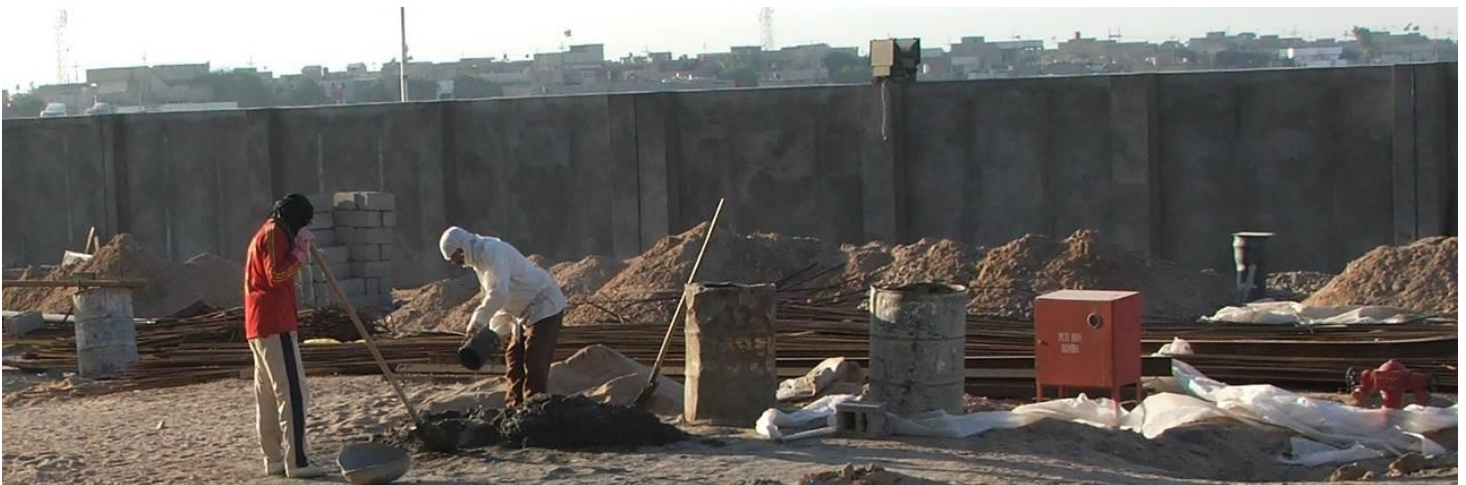
Site Photo 23. Perimeter security wall construction
