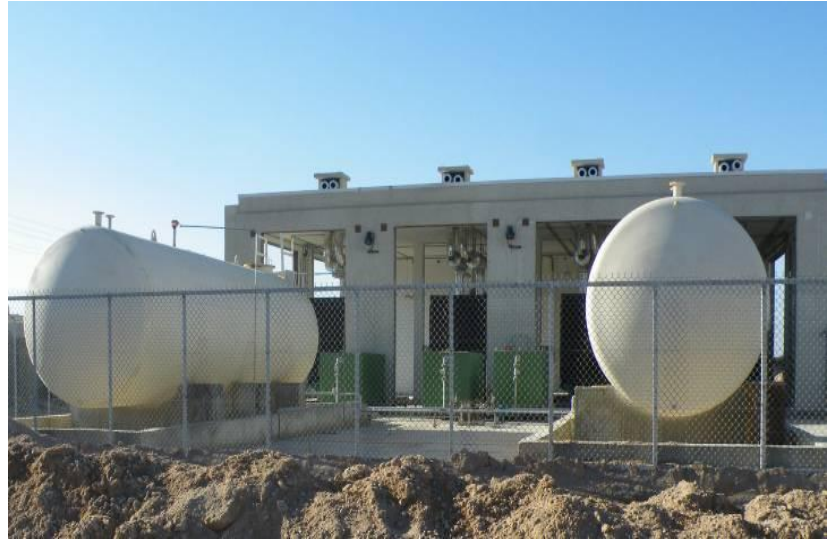
Site Photos 21 and 22. Electrical generators and diesel fuel storage tanks
