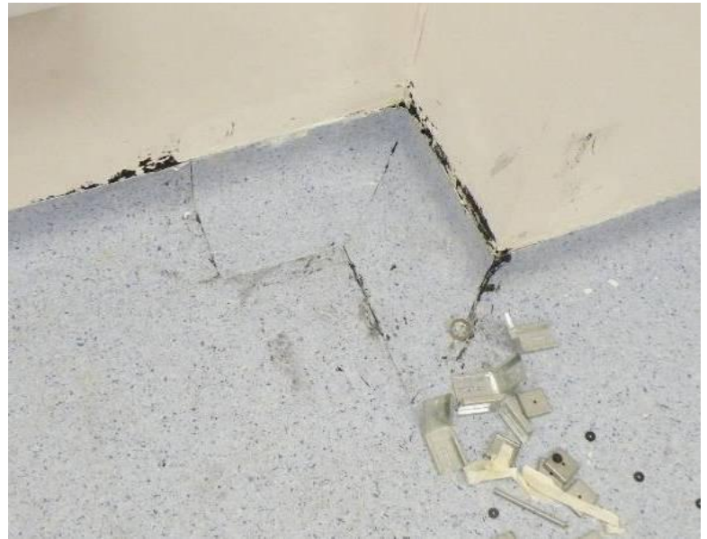
Site Photos 16 and 17. Poor installation of vinyl flooring as noted on punch list
