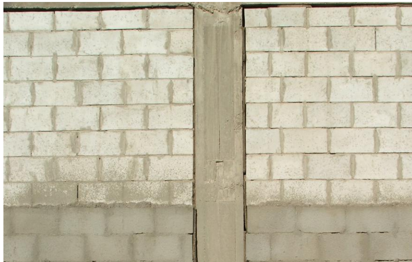
Site Photo 3. Masonry block wall & concrete column--typical construction
