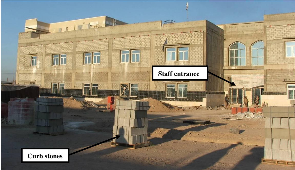
Site Photo 2. Curb stones and grading for the staff parking lot
