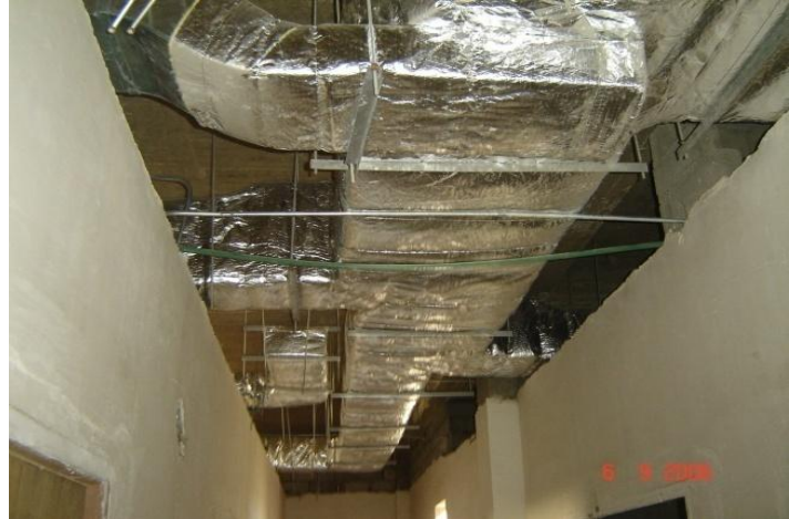
Site Photos 2 and 3. Installation of electrical wiring and HVAC duct work, respectively (Courtesy of USACE)
