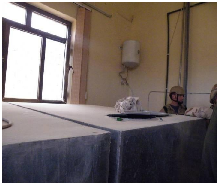
Site Photo 7. Uncovered equalization tank
