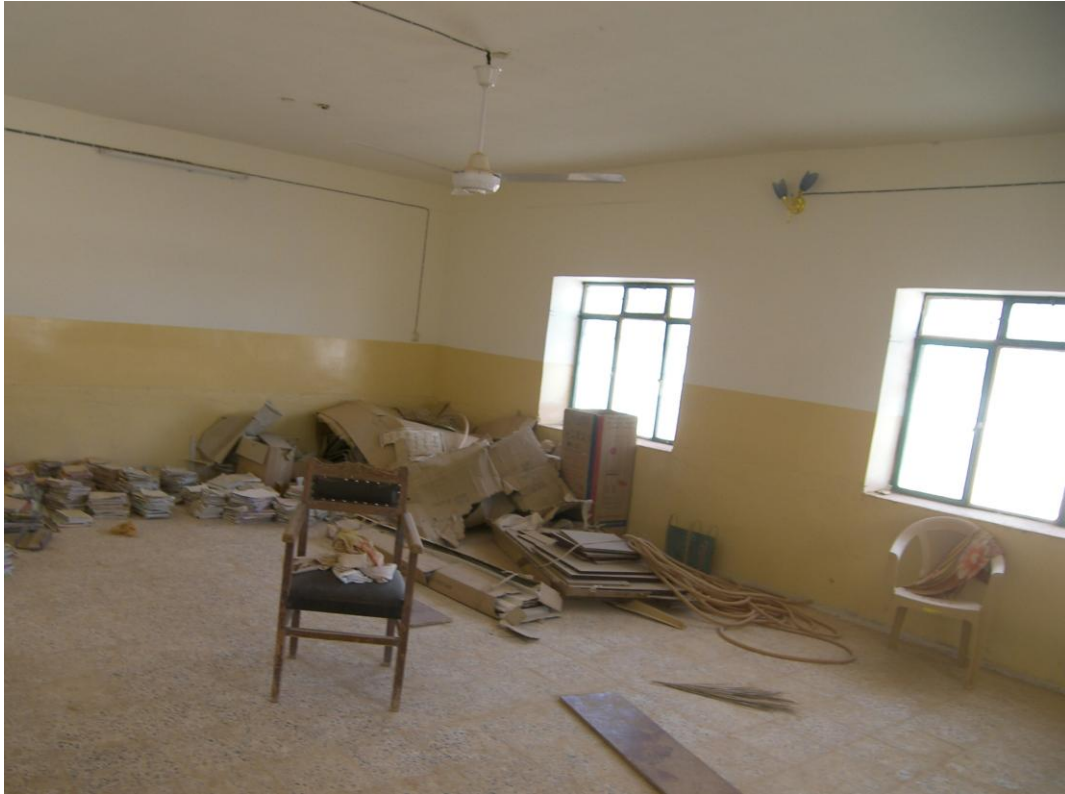
Site Photo 10. Schoolroom debris
