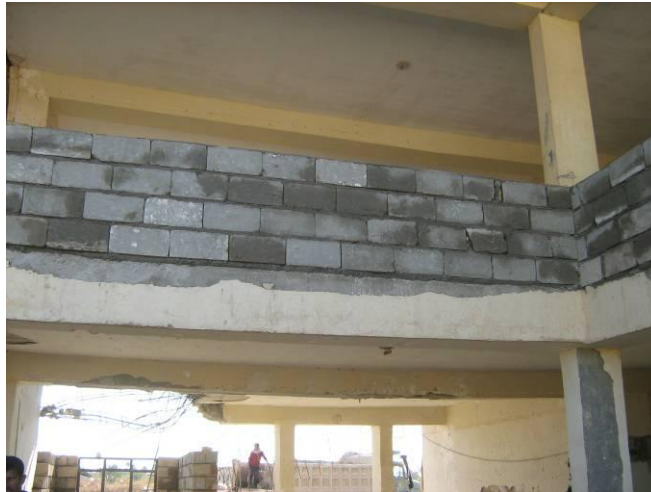
Site Photo 4. Masonry work during rebuilding (Courtesy MNC-I)
