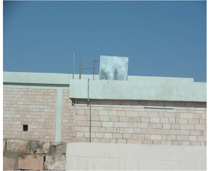
Site Photo 4. Exposed concrete masonry units
