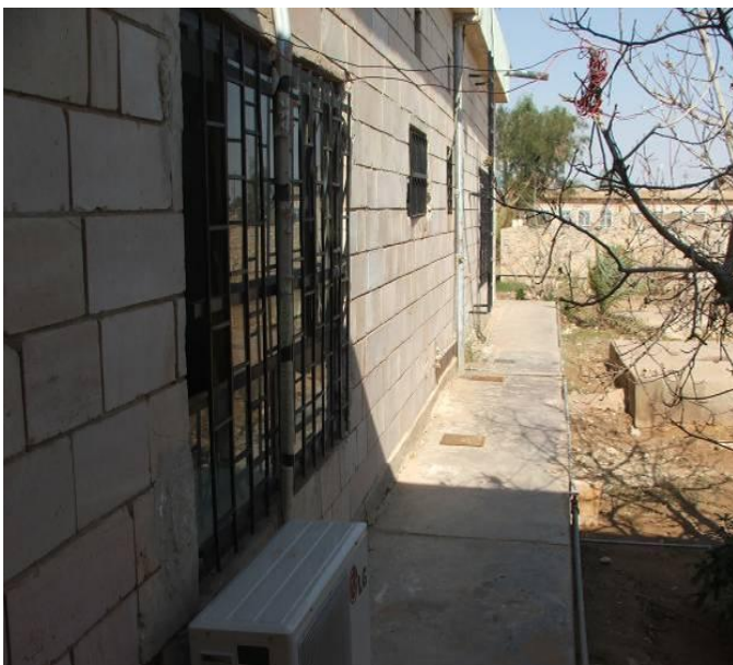
Site Photo 5. Newly constructed exterior windows
