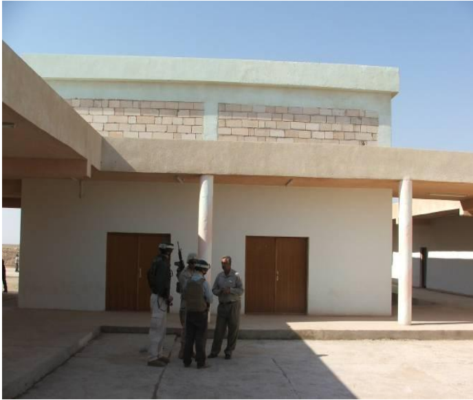
Site Photo 3. Structure with reinforced concrete frame
