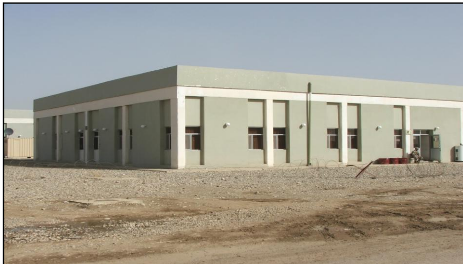
2 nd Brigade base DFAC building
