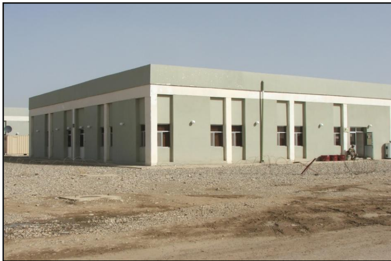
Exterior of the Al Kut East barracks building
