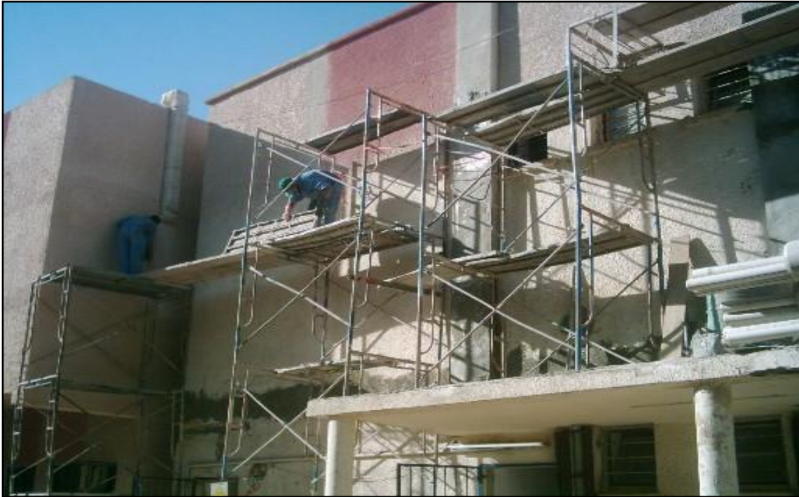
Construction work at the Al Alwaiya Children's Hospital
