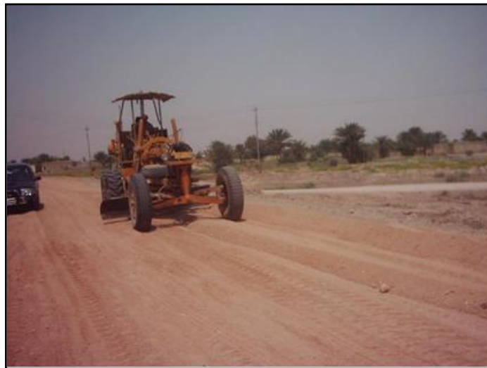
Muthanna village roads under construction
