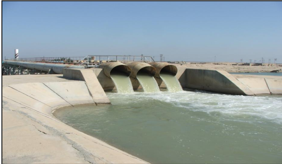
Port of Umm Qasr water canal in use
