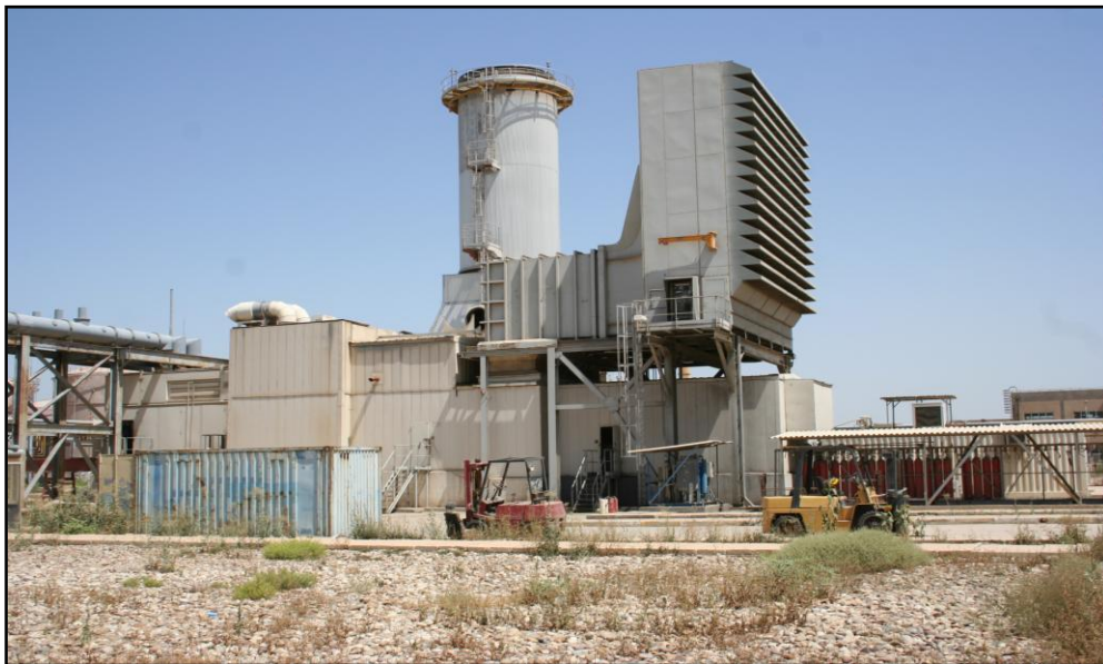
Qudas Power Plant
