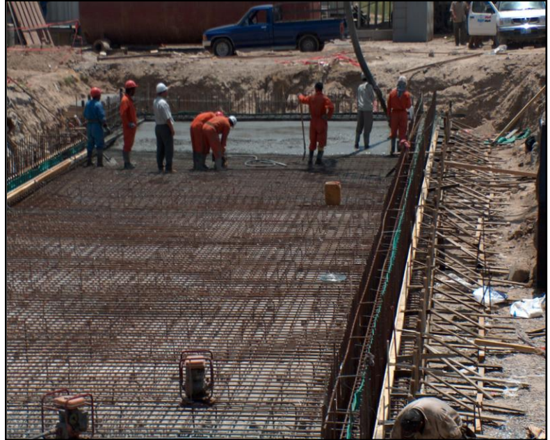
Construction work at Al Wathba Water Treatment Plant
