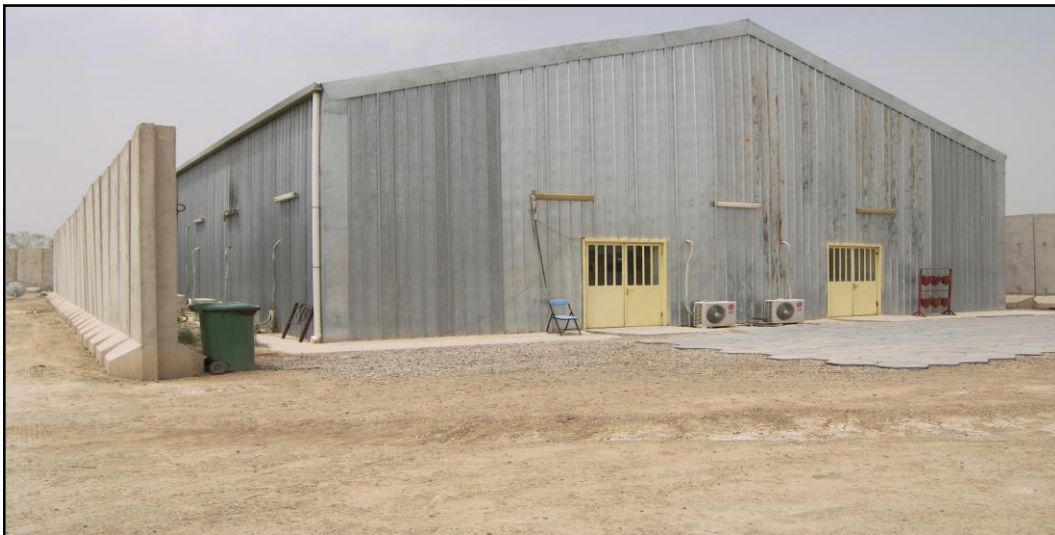
Exterior of an aircraft hangar at the Iraqi C-130 Base
