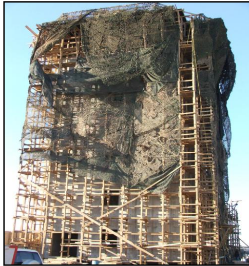
Air traffic control tower under construction at the Mosul Airport
