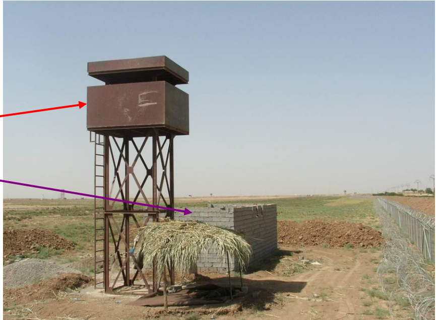
Site Photo 21. Partial construction of the MOD guard towers
