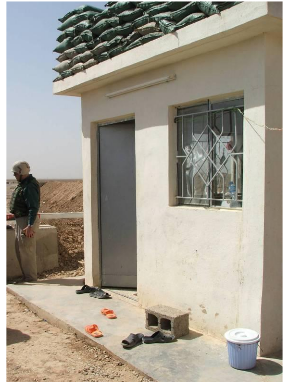
Site Photo 18. Window with screen and lockable steel door
