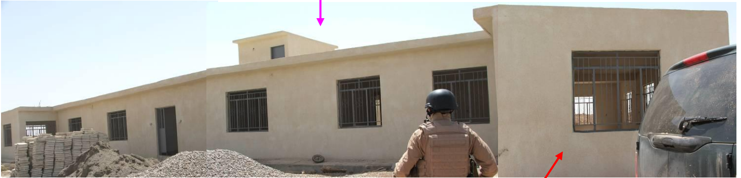
Site Photo 25. View of exterior of partially constructed company headquarters
