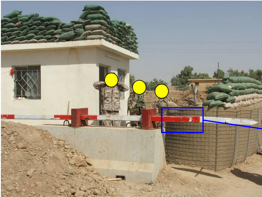
Site Photo 15. Gate post in for the guard house
