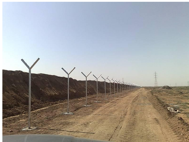
Site Photo 6. Installed PEZ fence posts (Photo courtesy of the USACE)
