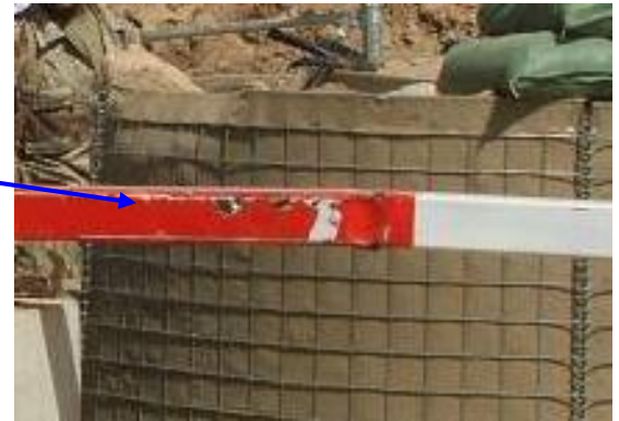
Site Photo 16. Close-up of Site Photo 15
