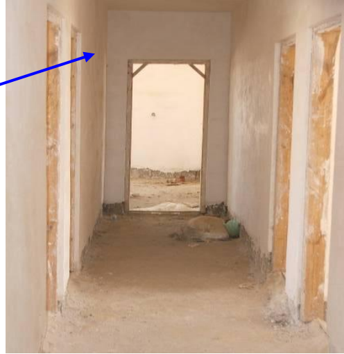
Site Photo 24. Partially constructed hallway
