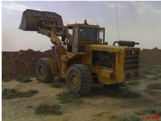
Site Photo 4. Formation of the PEZ berm (Photo courtesy of the USACE)
