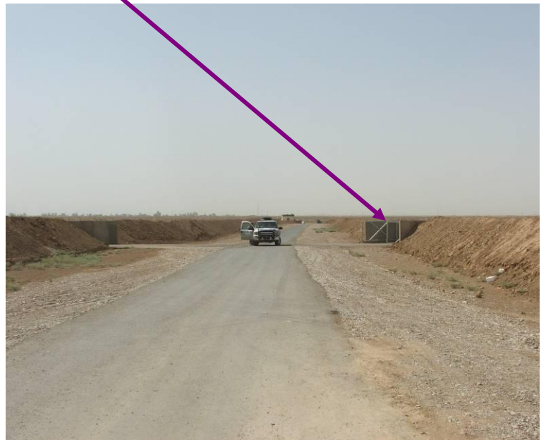
Site Photos 13 and 14. Asphalt road and chain link gate for the road crossing
