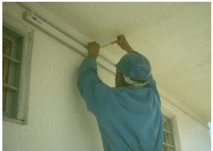
Site Photo 4. New lighting installation (Courtesy of GRC)
