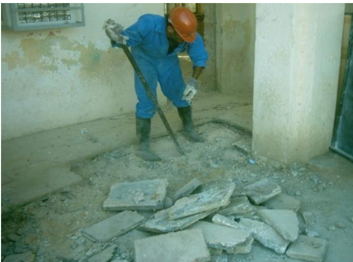
Site Photo 3. Demolition of tiles (Courtesy of GRC)
