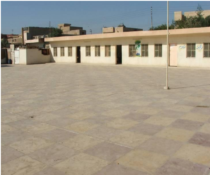
Site Photos 5. New walkway tiles
