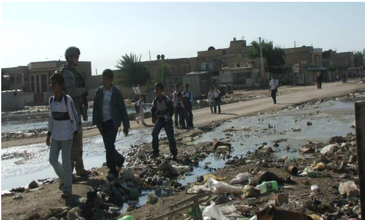
Site Photo 15. Make-shift levee for students to avoid walking through standing water and sewage
