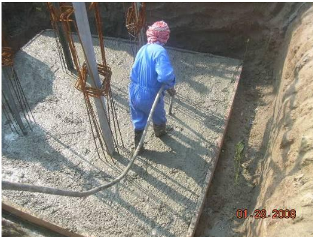
Site Photo 7. Vibrating concrete (Courtesy of the USACE)
