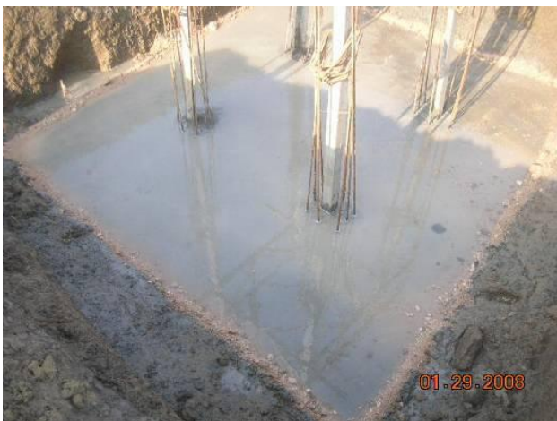
Site Photo 9. Curing concrete (Courtesy of the USACE)
