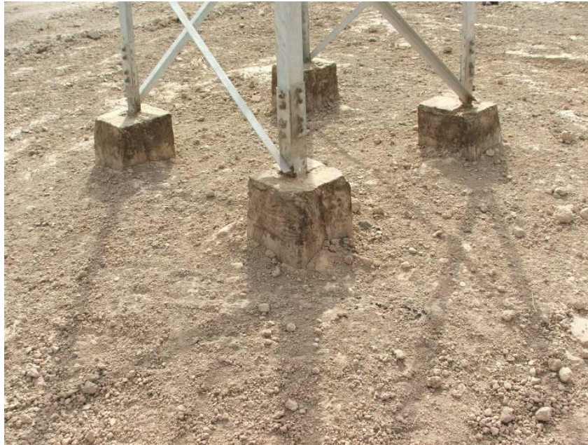
Site Photo 1. Completed tower foundation
