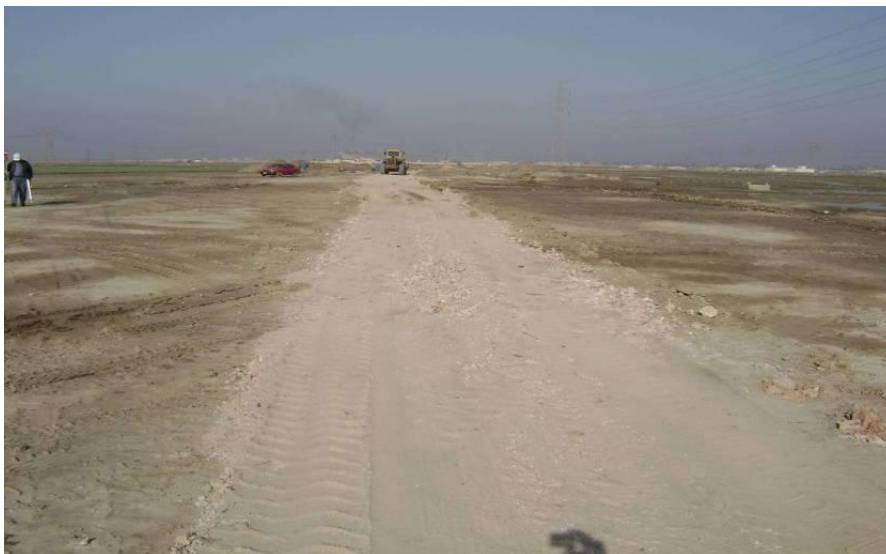
Site Photo 2. Construction of service road (Courtesy of the USACE))
