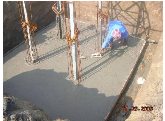
Site Photo 8. Finishing concrete (Courtesy of the USACE)
