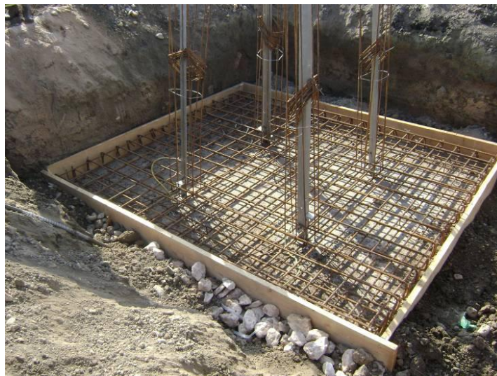
Site Photo 4. Forming up tower foundation (Courtesy of the USACE))
