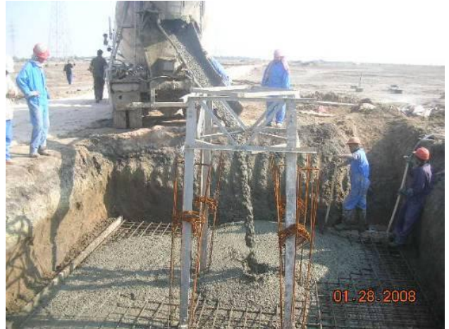
Site Photo 6. Concrete pour for tower (Courtesy of the USACE)
