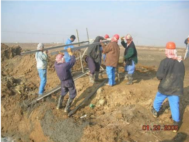
Site Photo 5. Erecting base of tower (Courtesy of the USACE)
