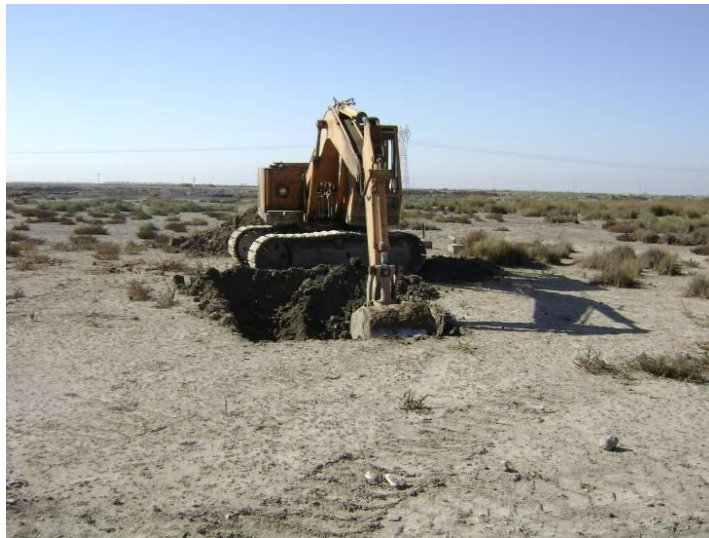
Site Photo 3. Excavation for tower foundation (Courtesy of the USACE))
