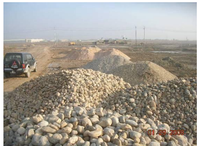
Site Photo 10. Aggregate delivered to site (Courtesy of the USACE)
