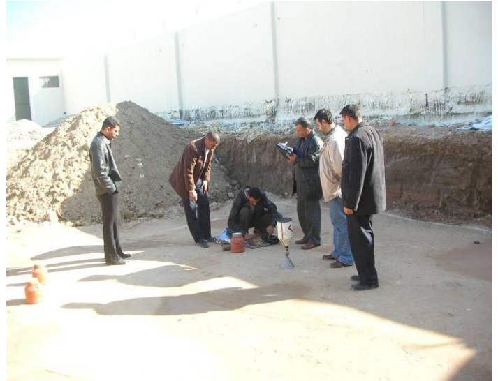
Site Photo 5. Concrete testing being performed.
