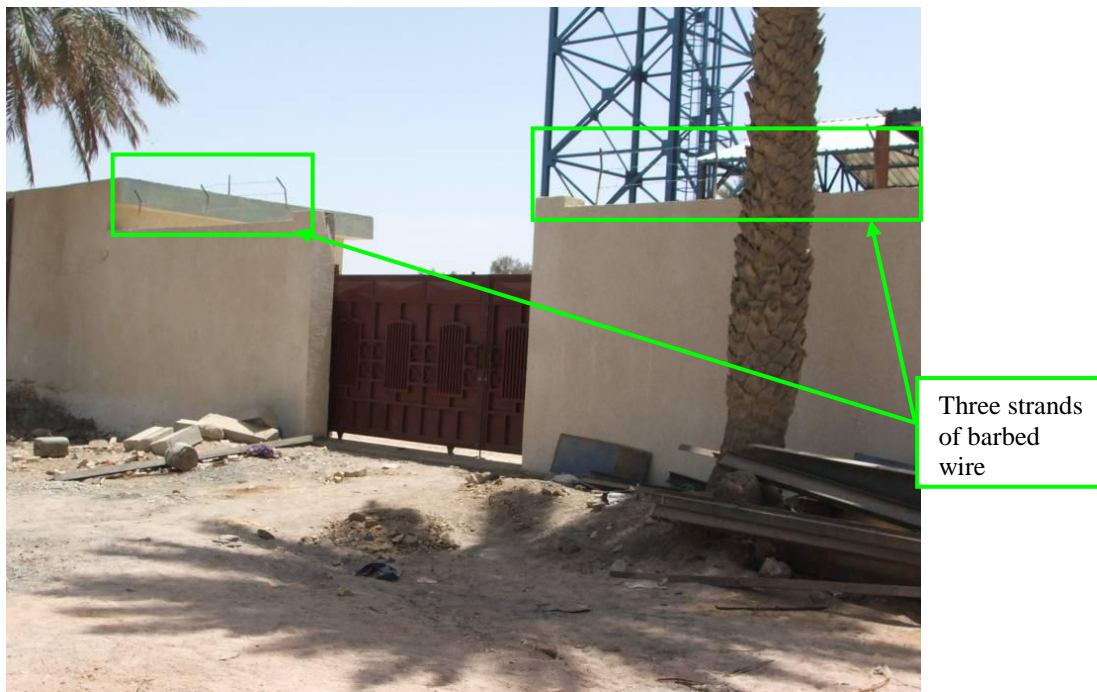
Site Photo 8. Finished exterior site fencing
