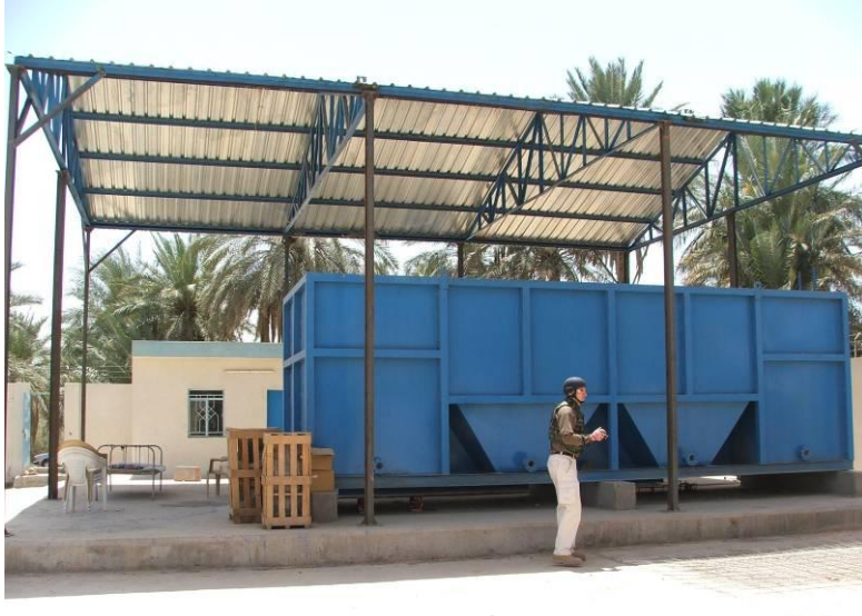
Site Photo 4. Reinforced concrete pad for the WTP.
