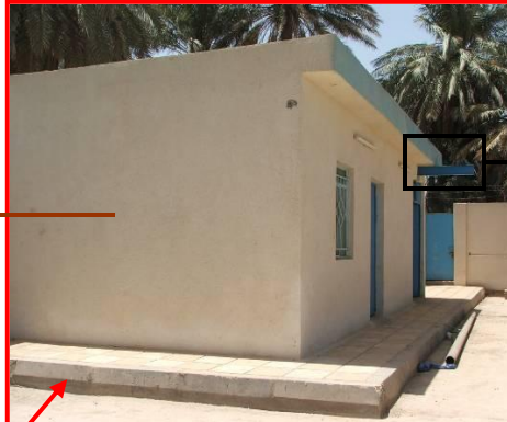
Site Photo 10. Chemical building
