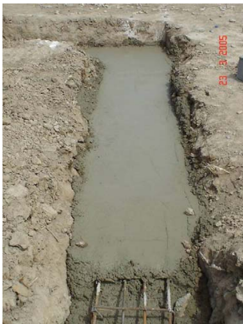
USACE Construction Progress Photo 3. Trench following pouring concrete.
