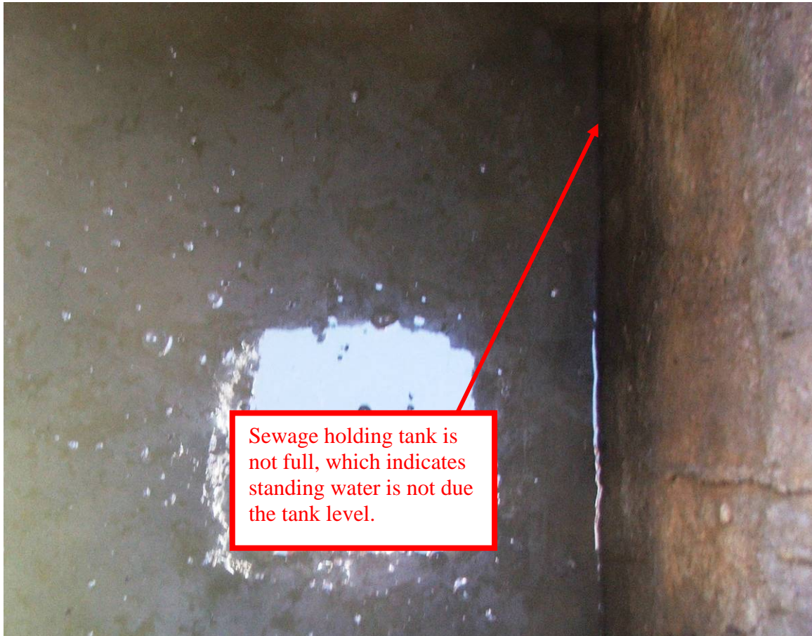
Site Photo 7. Sewage tank outside company barracks.
