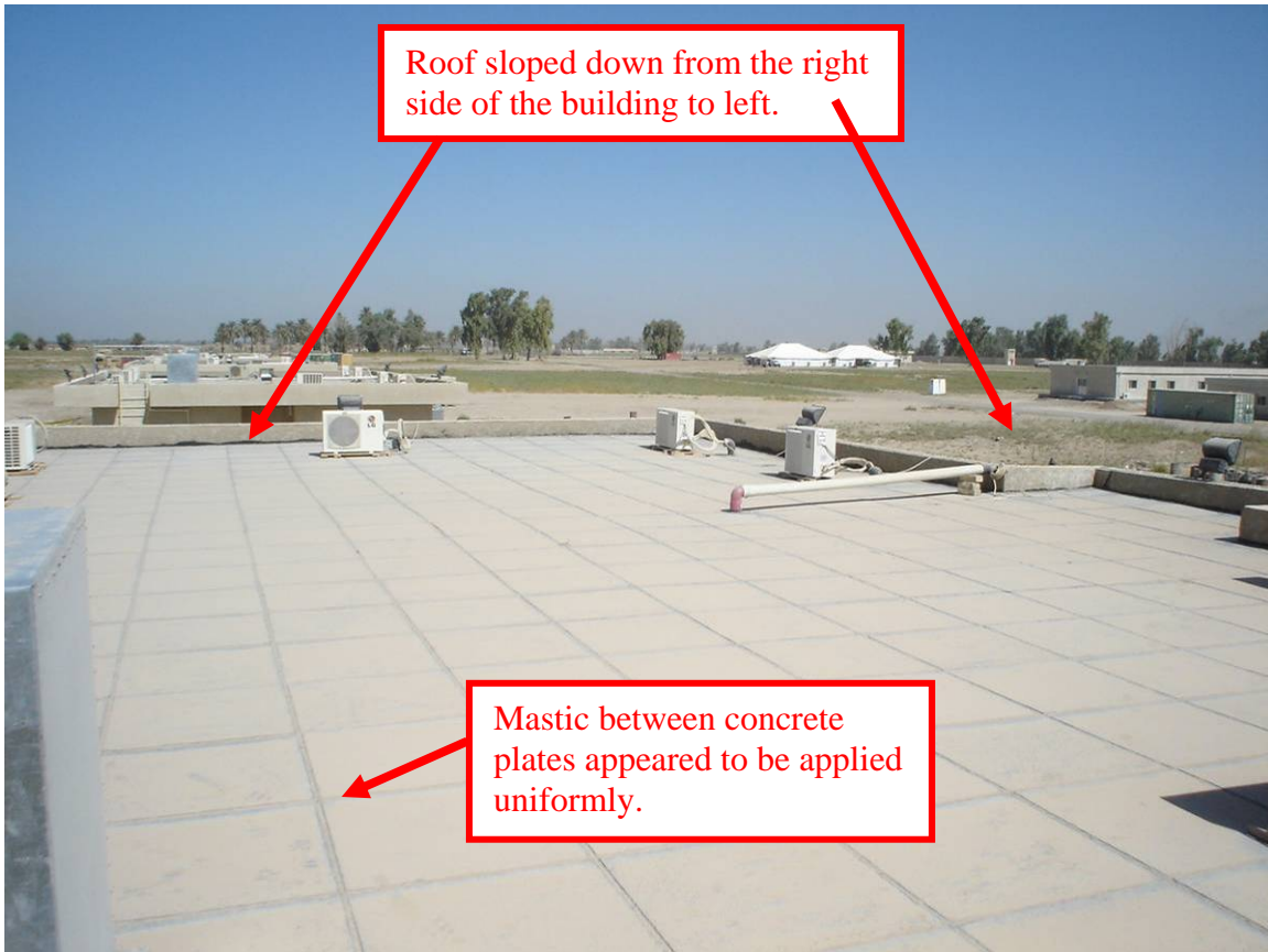
USACE Construction Progress Photo 7. Roofs were sloped to facilitate drainage.
