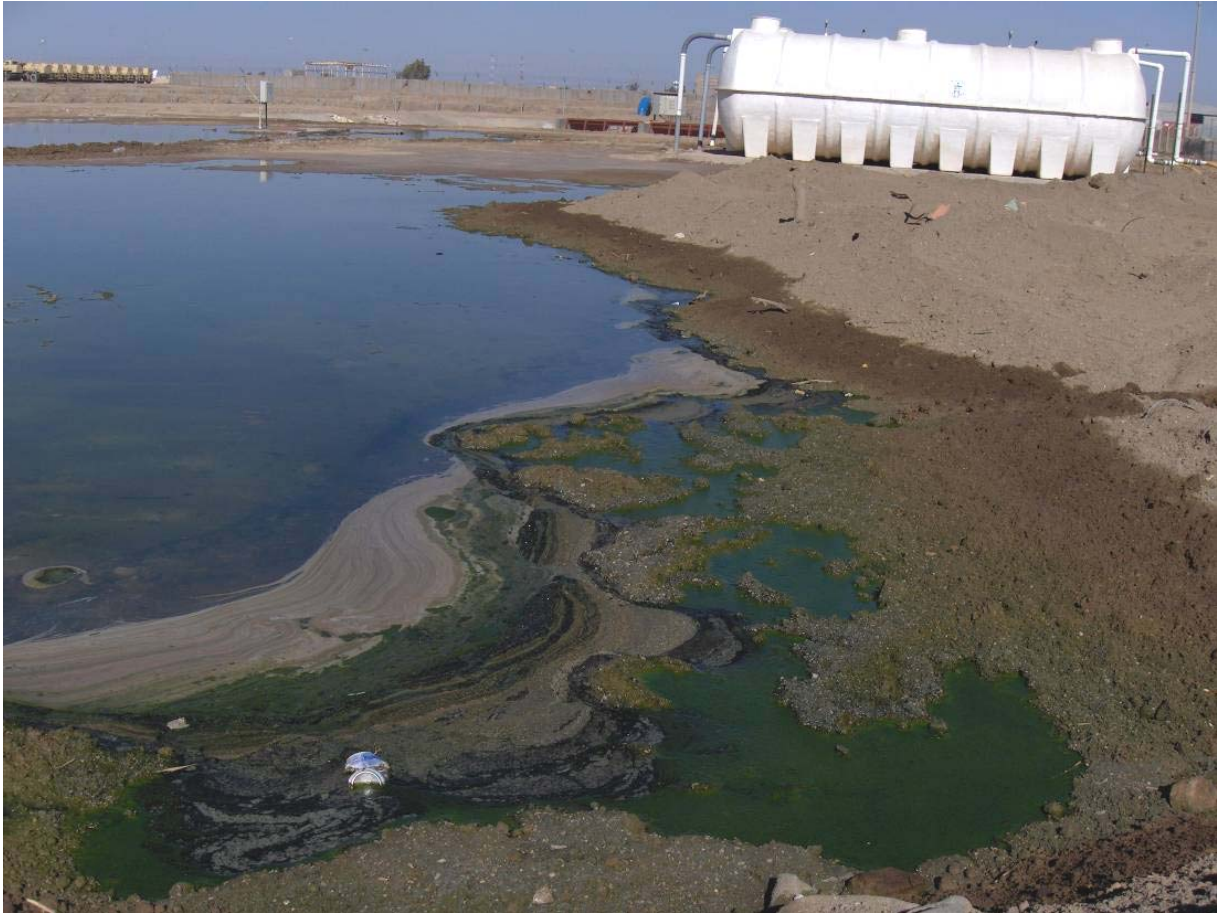
Site Photo 4. Sewage overflows around the holding tanks. (Contractor provided photo)
