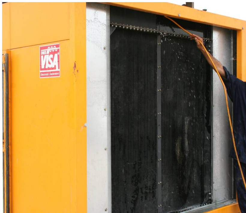
Site Photo 12. Worker cools a running generator with water.
