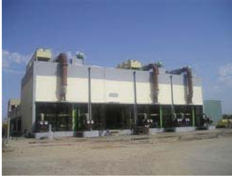
Site Photo 2. Exterior view of the generator's building (Photo provided by USAID)
