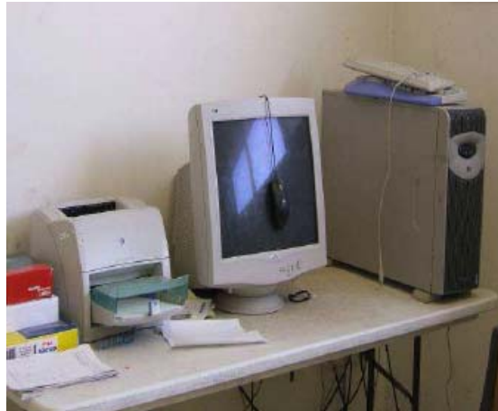
Site Photo 10. Programmable Logic Controller system workstation (Photo provided by USAID)
