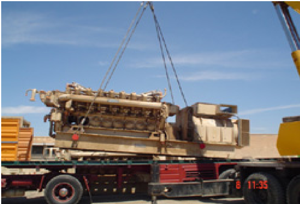
Site Photo 1. Existing Cockrill generator removal (Photo provided by USAID)
