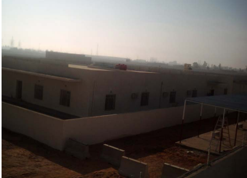
Site Photo 3. Jersey barriers blocking vehicle access to the building rear where the sewage holding tanks are located. (From Weston Photo Log)
