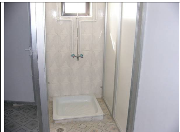
Site Photo 3. Example of a finished shower immediately after construction (From Weston photo log)
