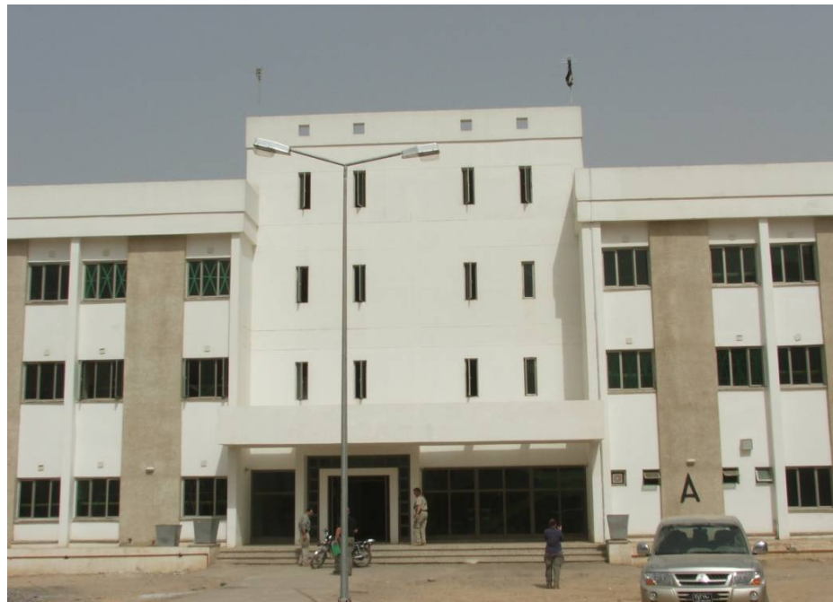
Site Photo 3. Outside view of cadet barracks building
