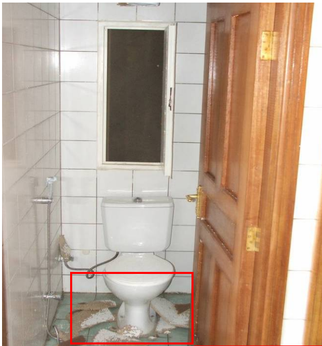
Site Photo 223. Damaged ceiling panels that fell to the ground
