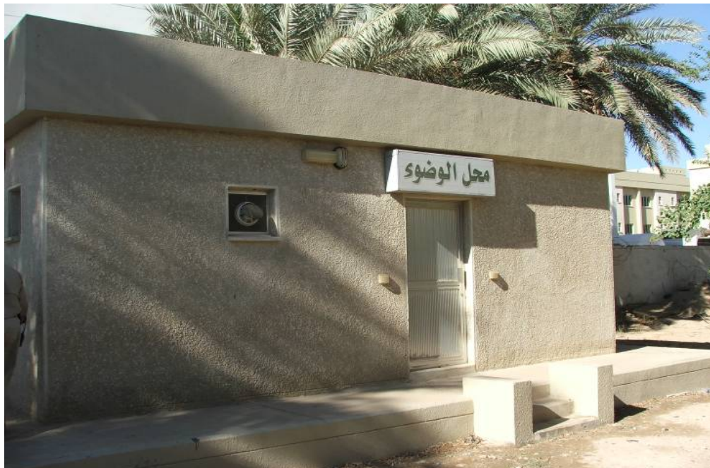
Site Photo 144. Exterior view of the ablution unit
