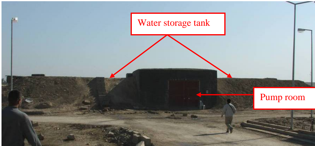
Site Photo 170. Exterior view of water storage tank and pump room
