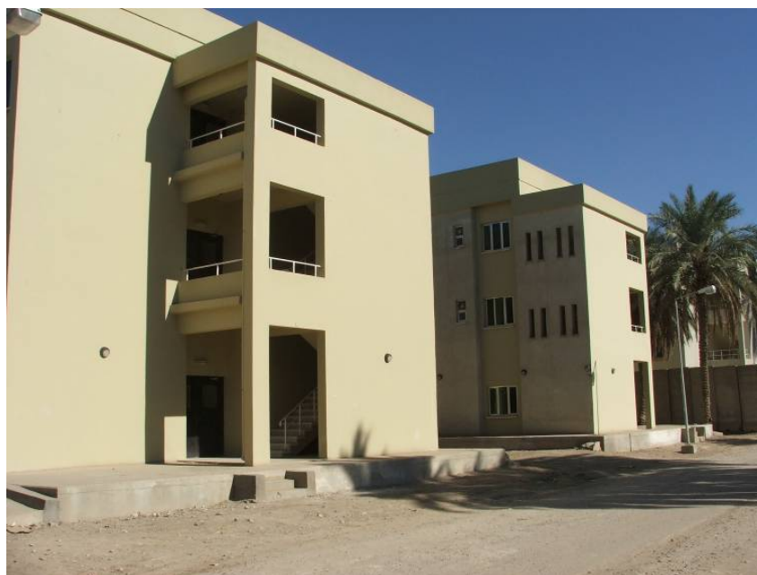
Site Photo 136. Exterior view of the language instructors' barracks
