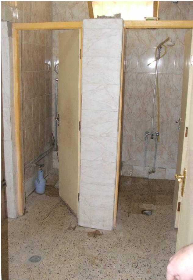
Site Photo 87. Renovated interior of BPC security office
