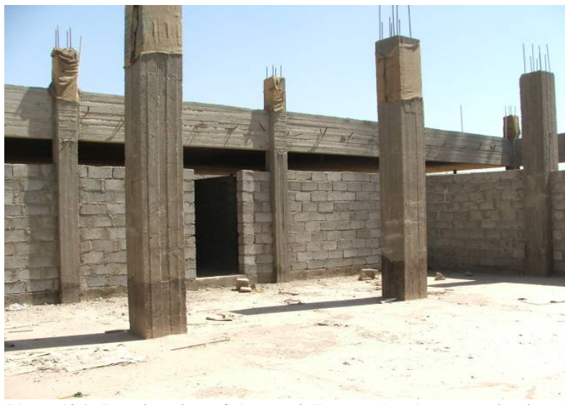
Site Photo 196. Interior view of the partially completed communications building
