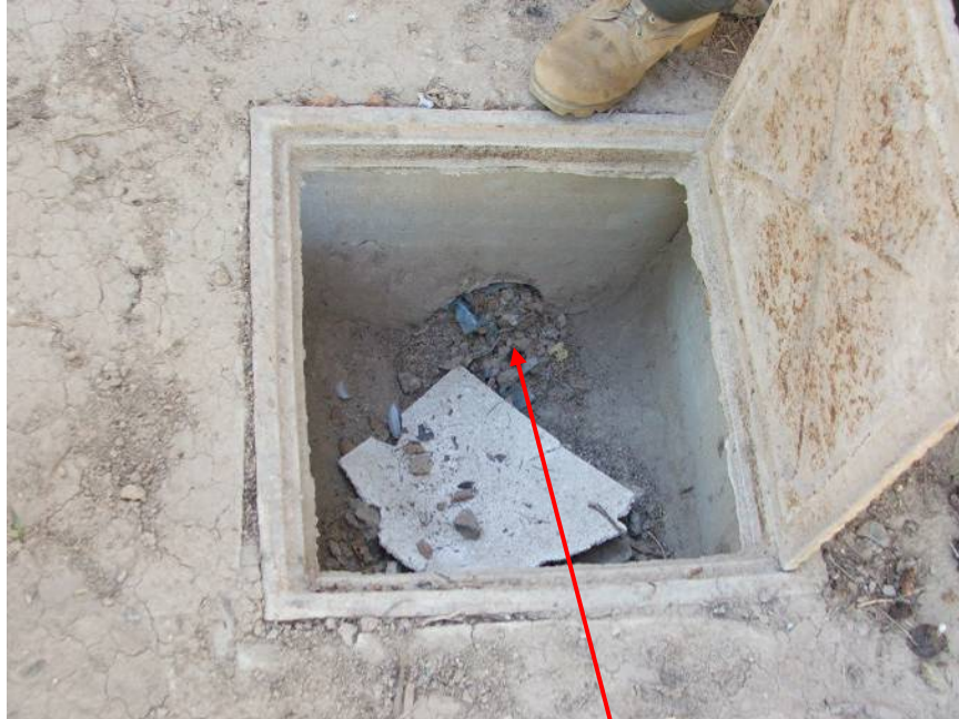
Site Photo 71. 10 November 2006 site visit, documenting ablation unit not connected to the sewer network.
