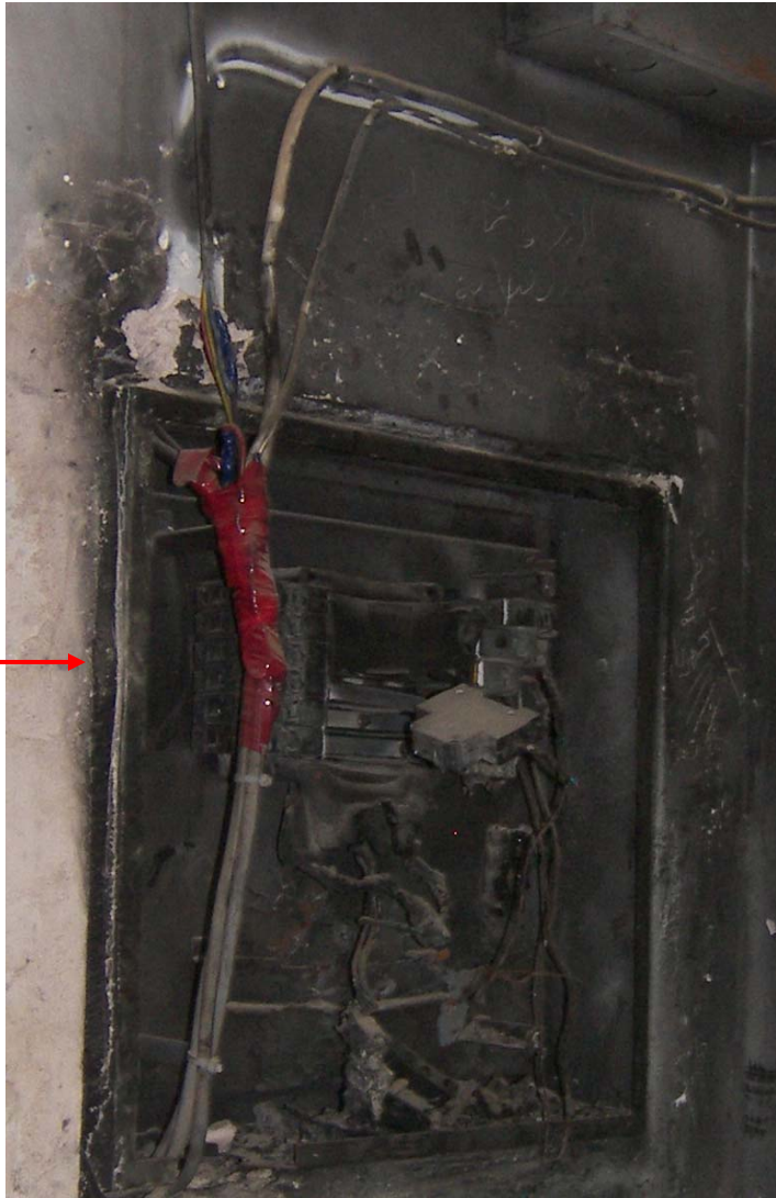
Site Photo 201. Close-up view of Site Photo 200.
