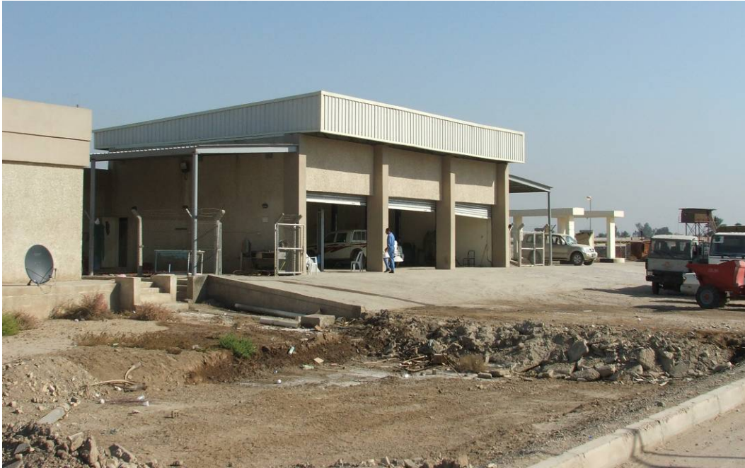
Site Photo 167. Exterior view of motor pool facility
