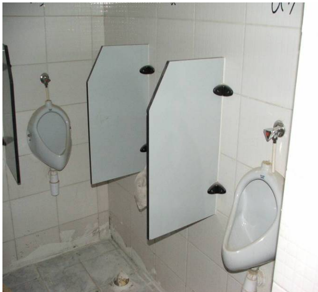
Site Photo 113. Urinals in cadet barracks
