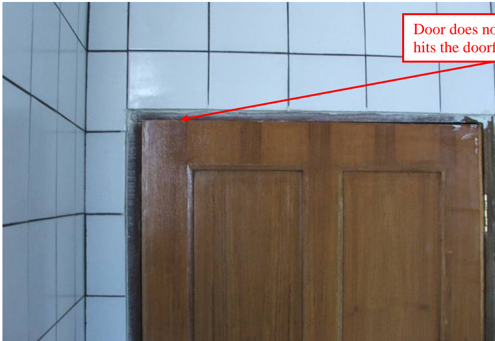
Site Photo 227. Door in Classroom E will not close completely since the floor was replaced
