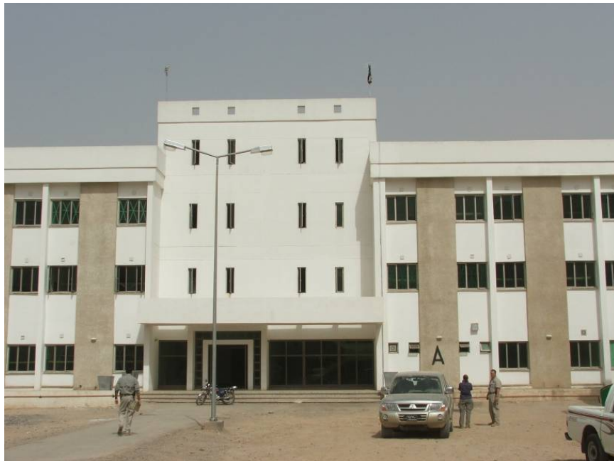
Site Photo 103. View of exterior of cadets' building
