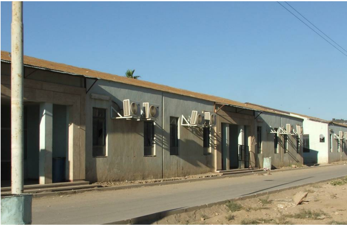
Site Photo 85. Example of typical existing BPC building exterior
