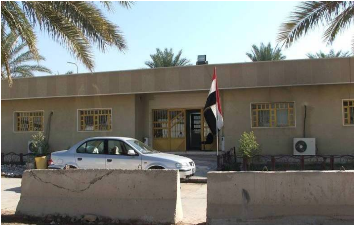
Site Photo 86. Front view of the BPC security office
