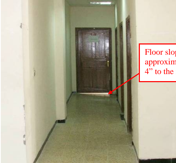
Site Photo 225. View of sloped floor in Classroom E
