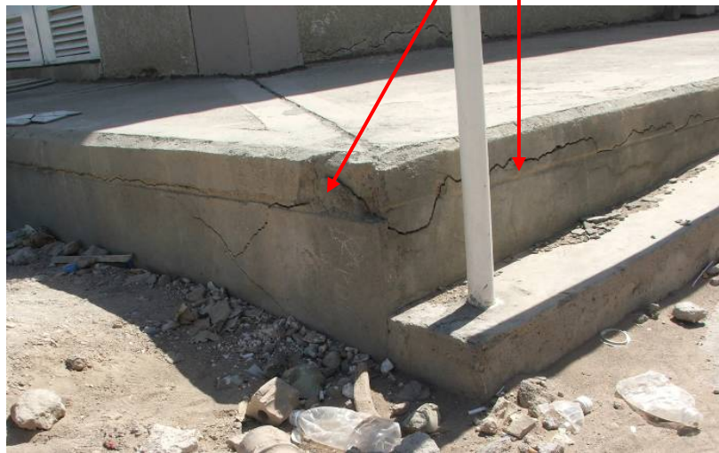
Site Photo 154. Close-up view of Site Photo 153
