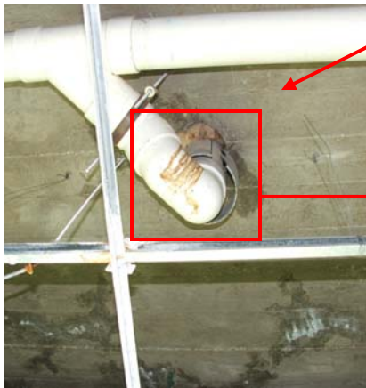
Site Photo 39. Plumbing installation in cadet barracks in August 2006
