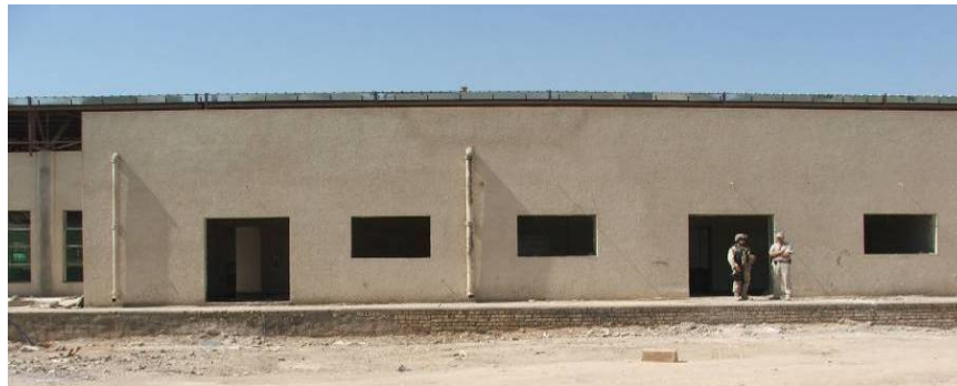
Site Photo 188. Exterior front view of partially completed indoor dining facility
