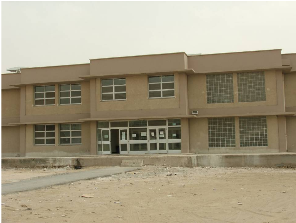
Site Photo 140. Exterior view of Classroom E
