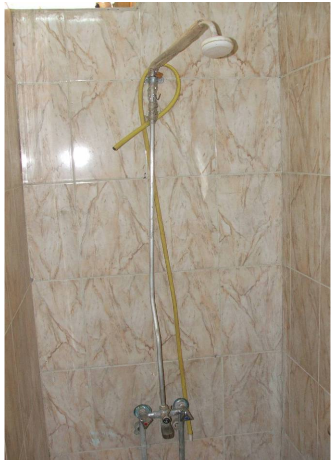
Site Photo 88. New bathroom tile with the BPC security office
