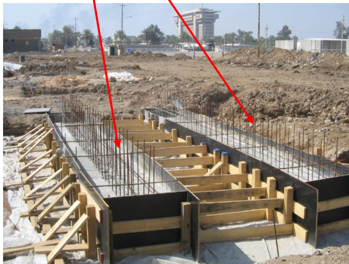
Site Photo 198. PT field foundation with reinforcement bars
