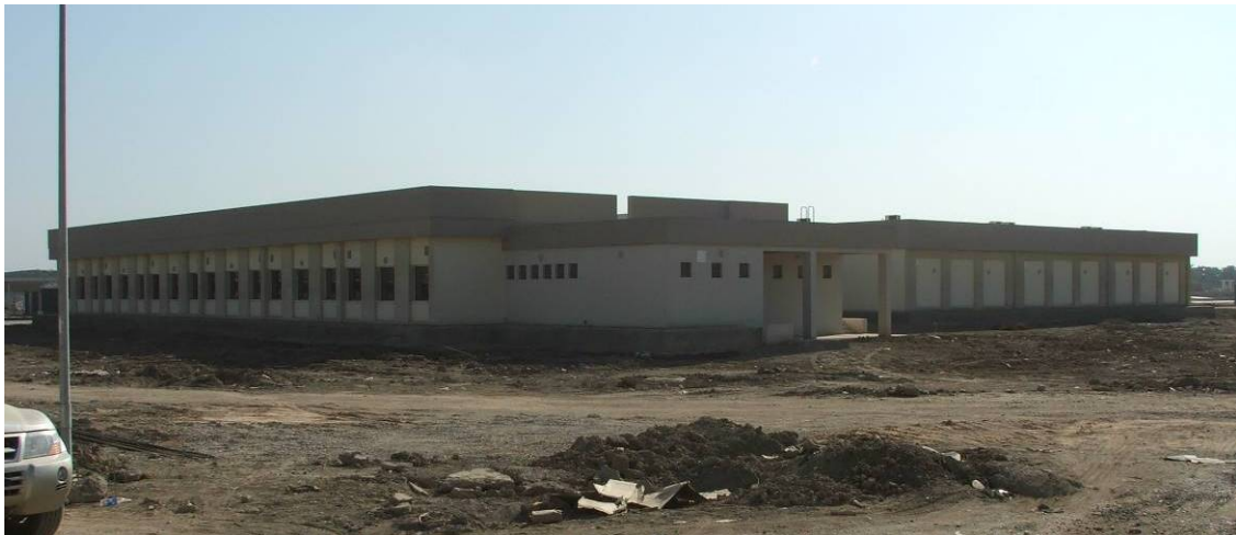
Site Photo 156. Exterior view of range administration building
