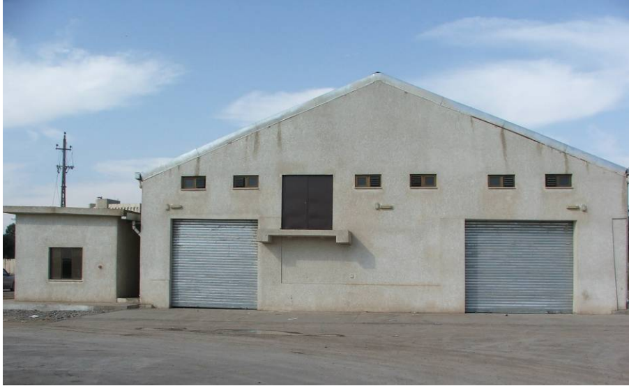
Site Photo 155. Exterior view of the armory building
