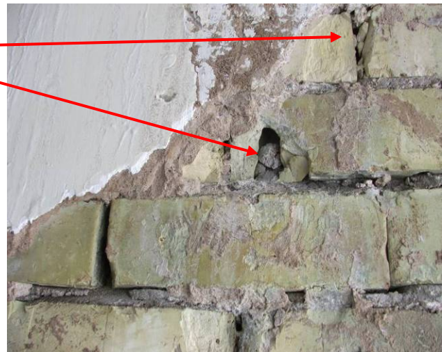
Site Photo 110. Close-up view of brickwork from Site Photo 109
