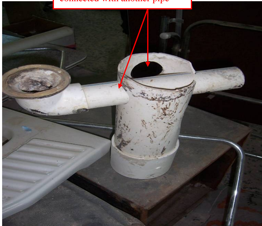
Site Photo 3. Typical cadet barracks plumbing fixture
