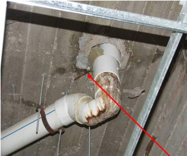
Site Photo 104. Cadet barracks concrete work
