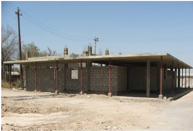
Site Photo 195. Exterior view of the partially completed communications building
