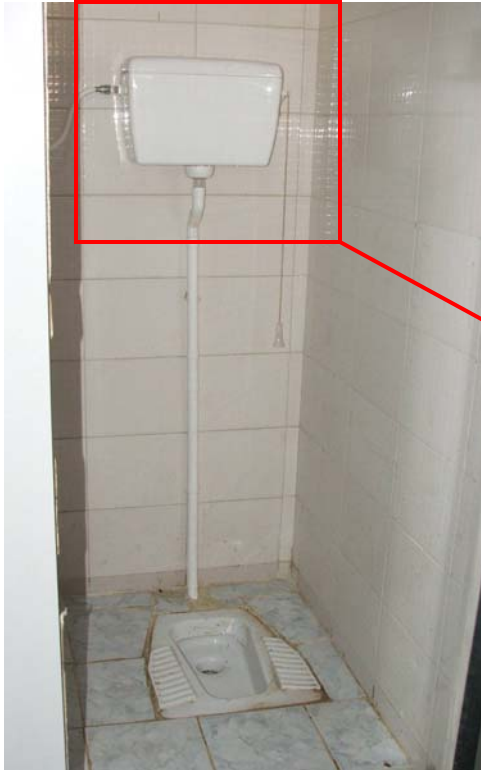
Site Photo 28. Water closet in cadet barracks
