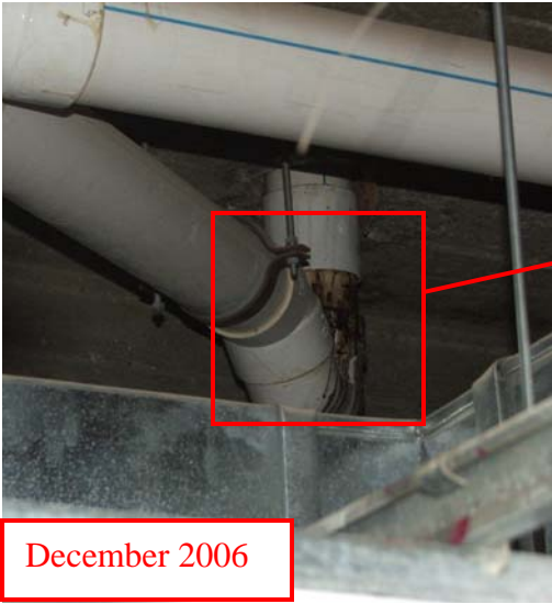
Site Photo 43. Leaking waste water from poorly sealed pipes
