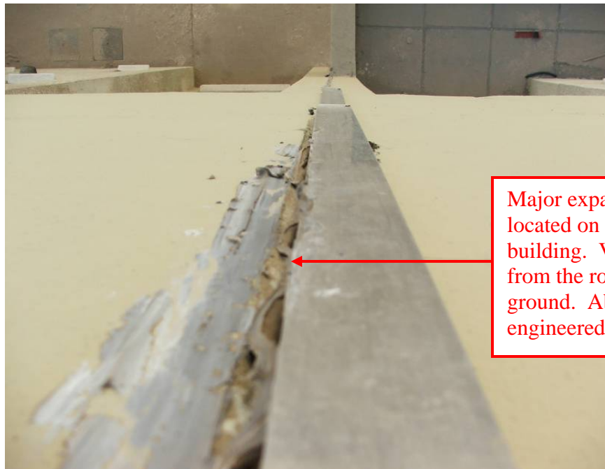
Site Photo 139. Significant exterior crack in the language instructors' barracks
