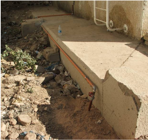
Site Photo 145. Connection to water network
