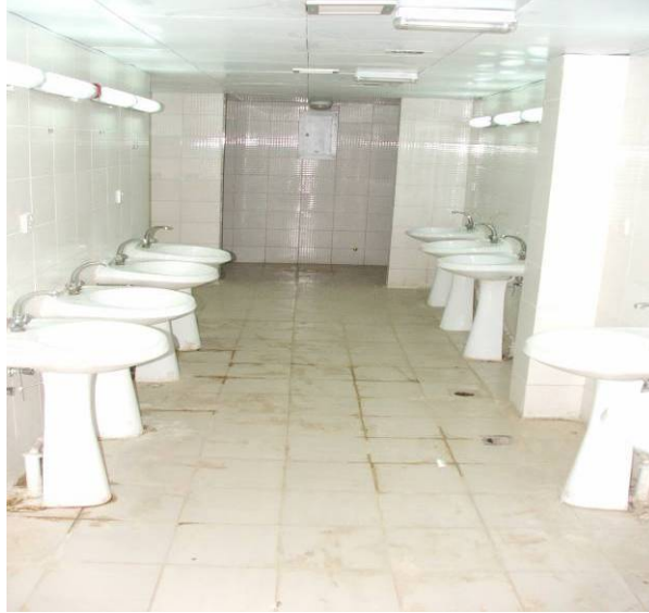
Site Photo 115. Sinks in cadet barracks bathroom
