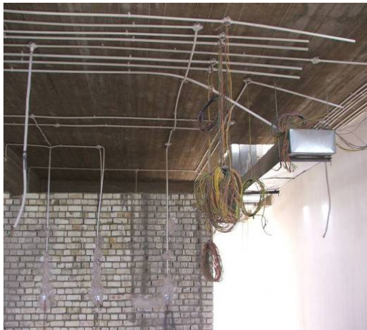
Site Photo 191. Work completed by Parsons
