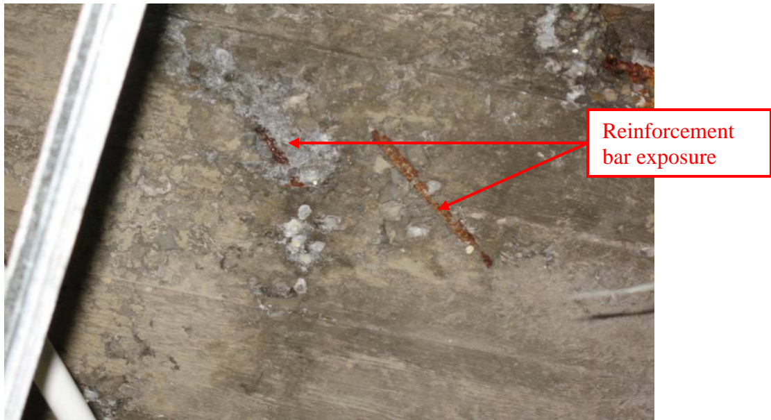
Site Photo 5. Reinforcement bar exposure in cadet barracks
