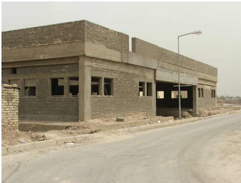
Site Photo 177. Exterior view of the central laundry facility
