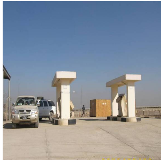
Site Photo 169. Re-fueling station
