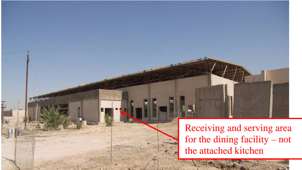
Site Photo 194. Exterior rear view of indoor dining facility
