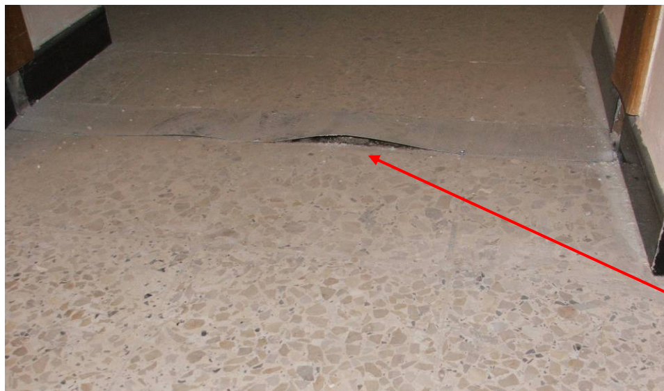
Site Photo 133. Interior expansion crack in the instructors' barracks
