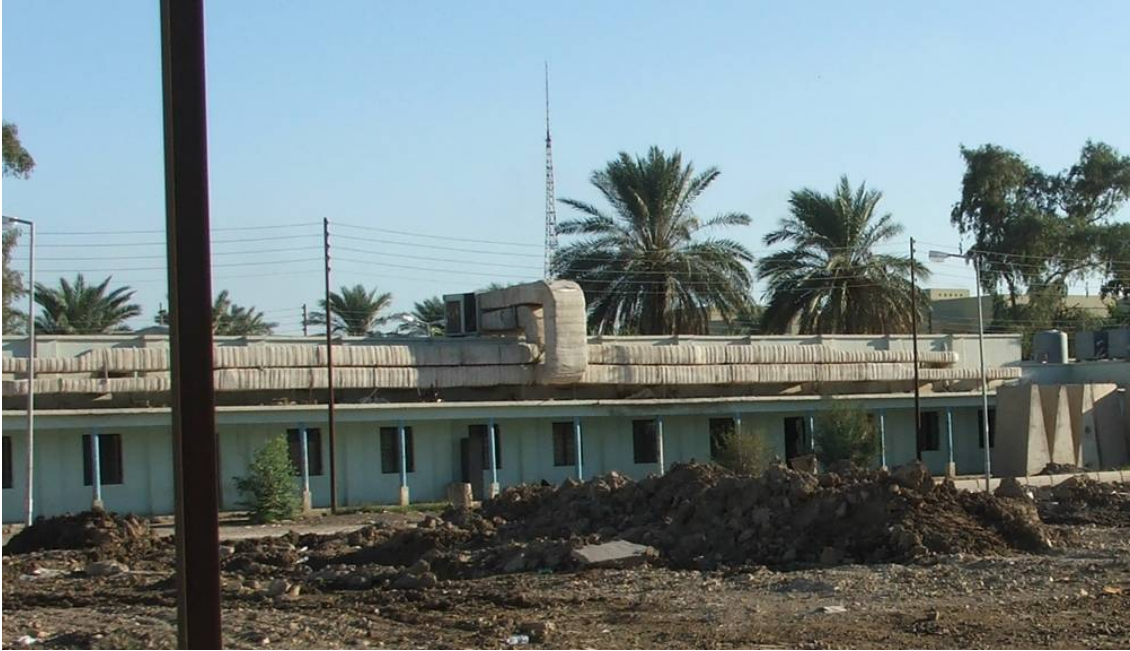
Site Photo 84. Example of typical existing BPC building exterior
