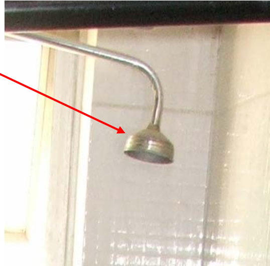
Site Photo 31. Close-up view of shower head
