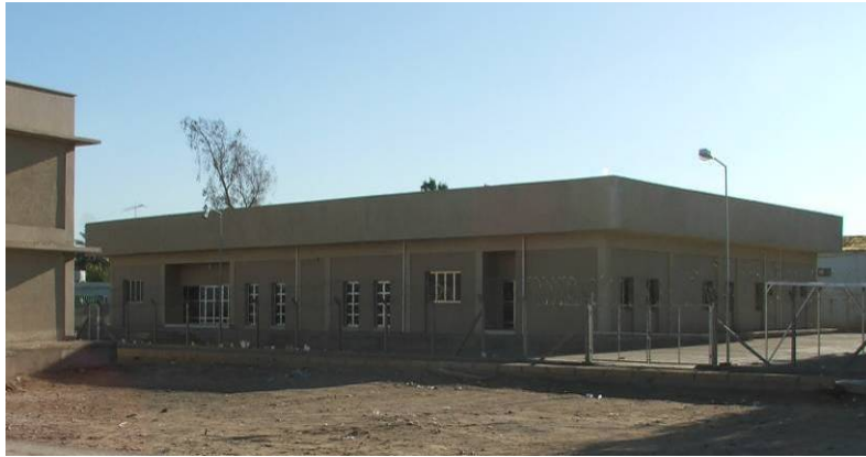
Site Photo 149. Exterior view of forensic laboratory
