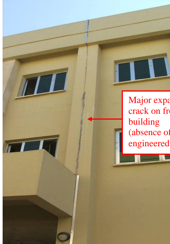
Site Photo 138. Exterior expansion crack
