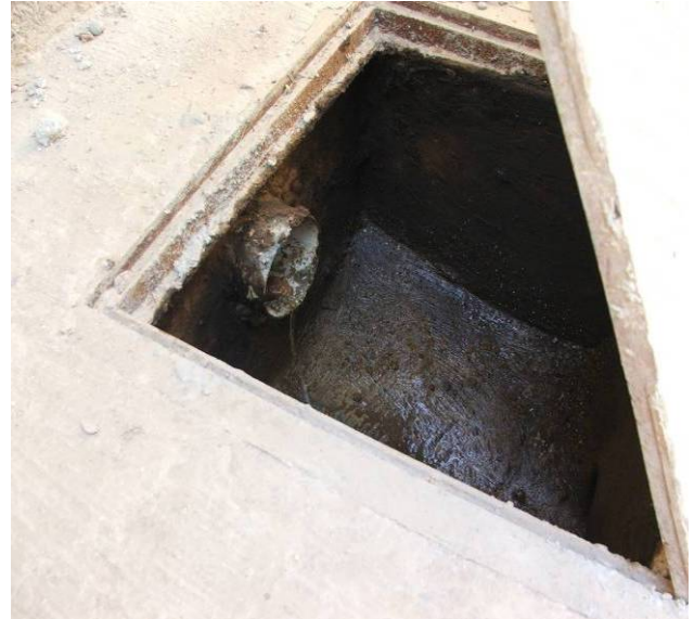
Site Photo 146. Connection to main sewer network
