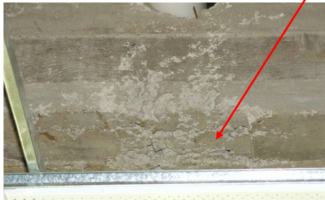
Site Photo 108. Cadet barracks concrete work
