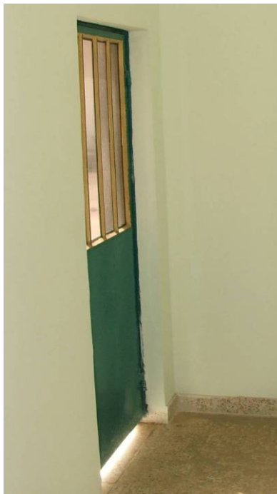
Site Photo 8. Medical clinic exterior door
