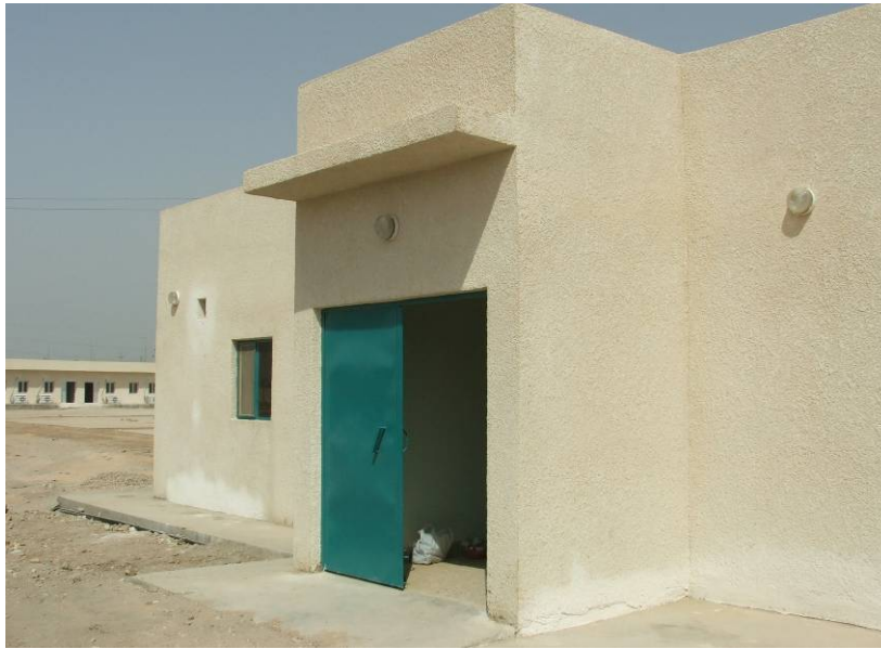
Site Photo 7. Exterior of the medical clinic
