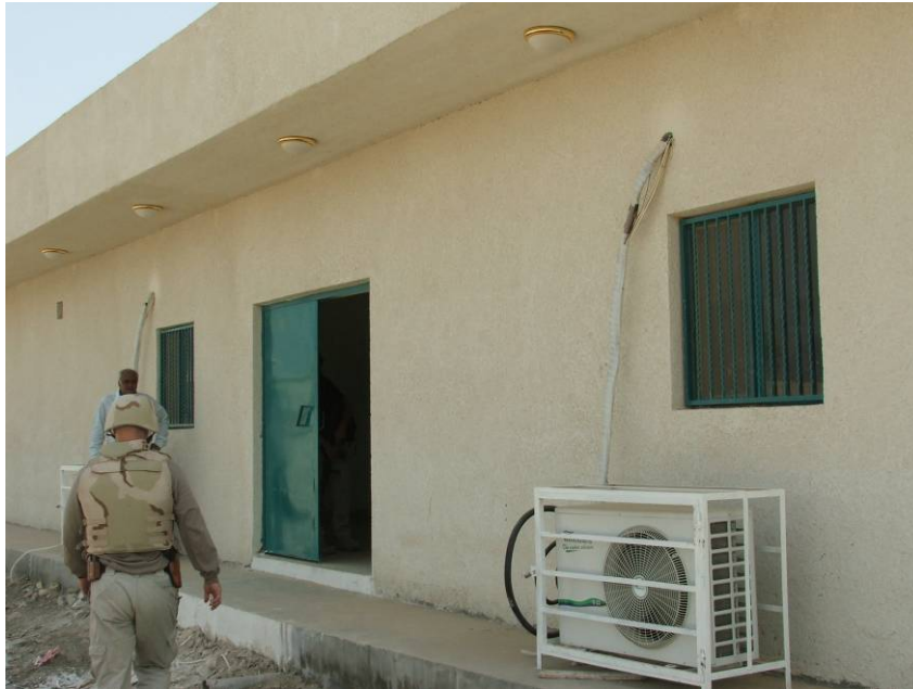
Site Photo 12. Exterior view of armory entrance
