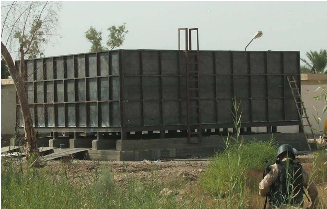
Site Photo 14. 300 m 3 water storage tank under construction
