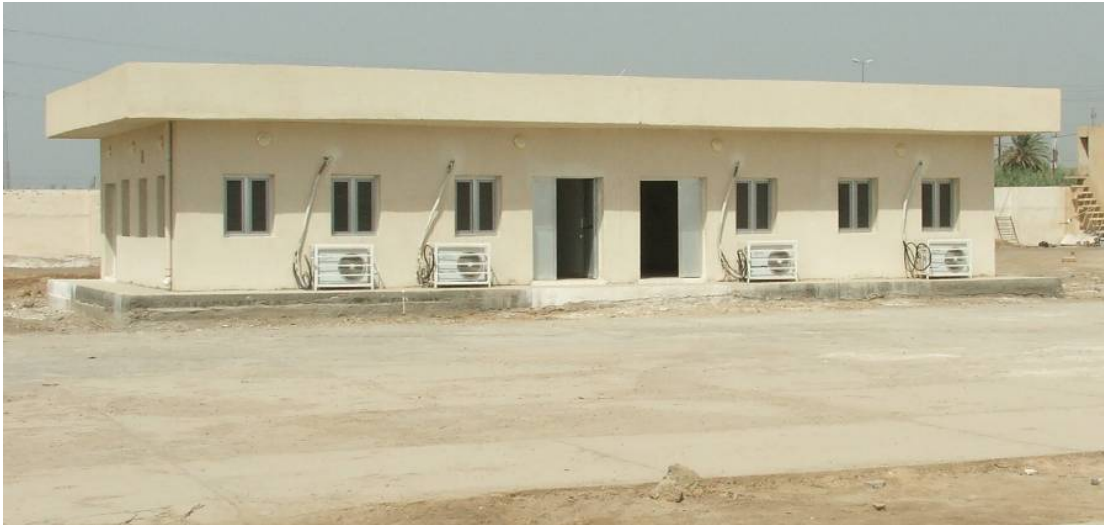
Site Photo 4. Classroom building with four classrooms
