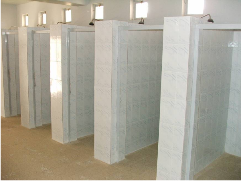
Site Photo 10. Ceramic tile finish on shower walls in ablution buildings
