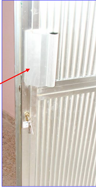
Site Photo 2. Barracks entrance door
