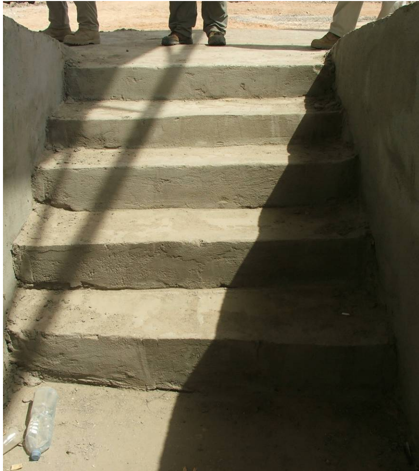
Site Photo 19. Concrete steps into the maintenance pit
