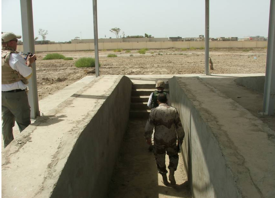
Site Photo 18. One of the three vehicle ramps and maintenance pits at the VMF
