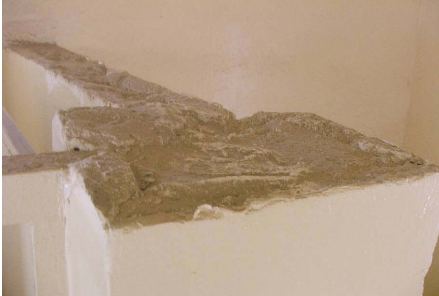
Site Photo 8. Top of privacy walls constructed in ablution buildings
