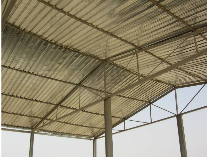
Site Photo 23. Roof truss system supporting the motor pool roof
