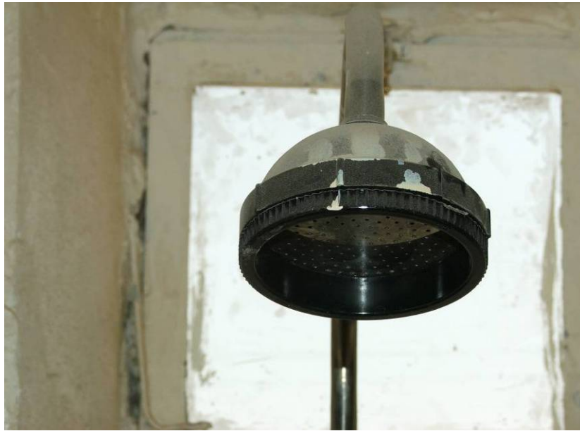
Site Photo 10. Shower head in ablution building
