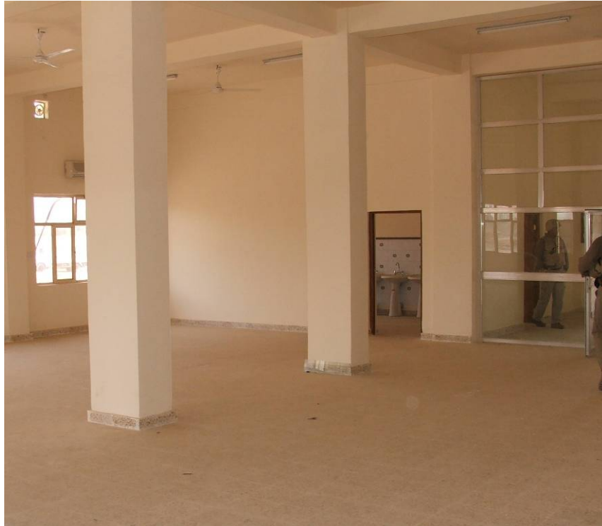
Site Photo 3. Dining room interior
