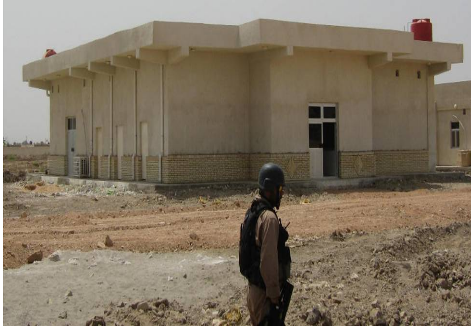
Site Photo 1. Dining facility exterior
