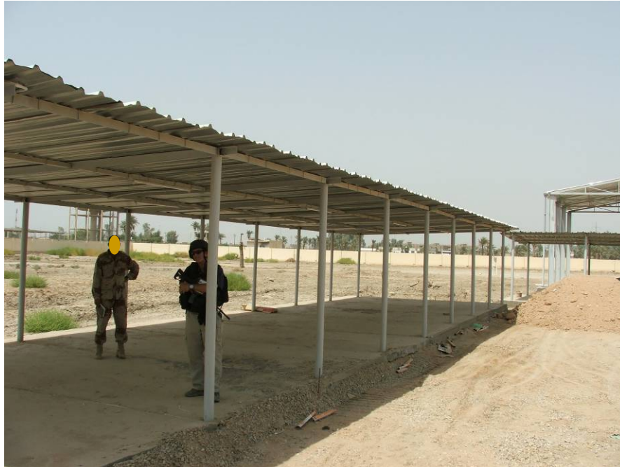
Site Photo 13. 40- vehicle parking sunshade
