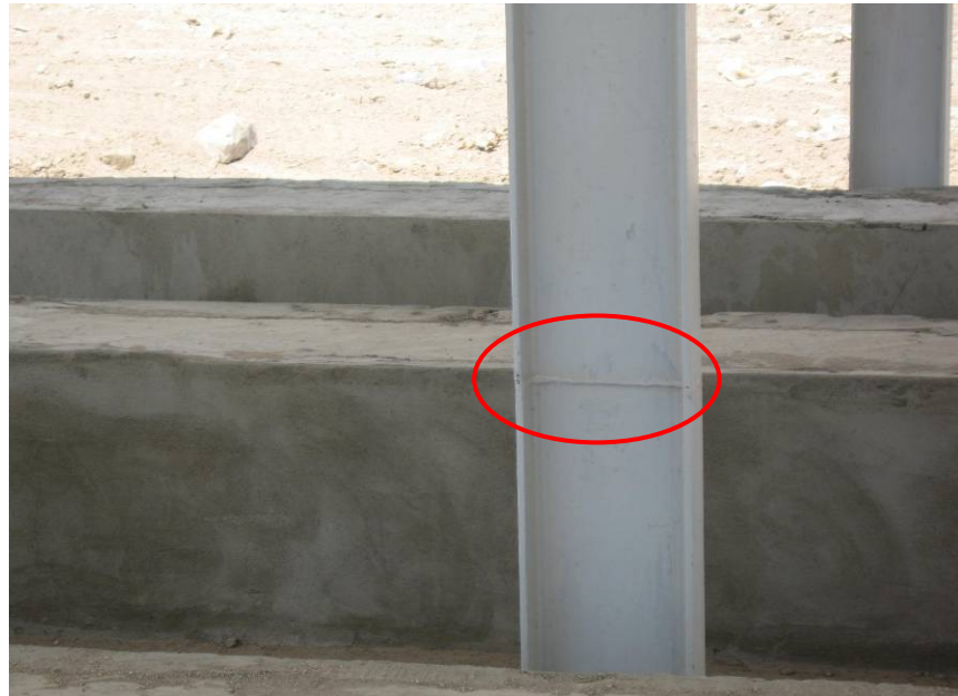
Site Photo 21. Spliced steel H-column at the motor pool
