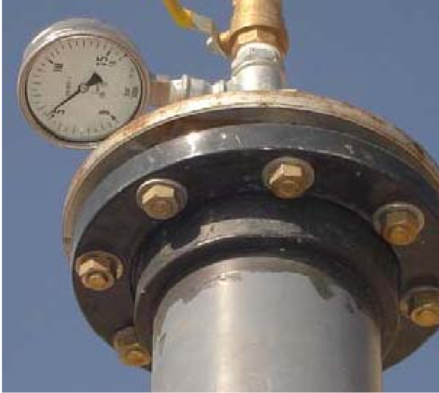
QA Photo 1. Pressure testing a pipeline (from QA Report 4 Oct 2005).
