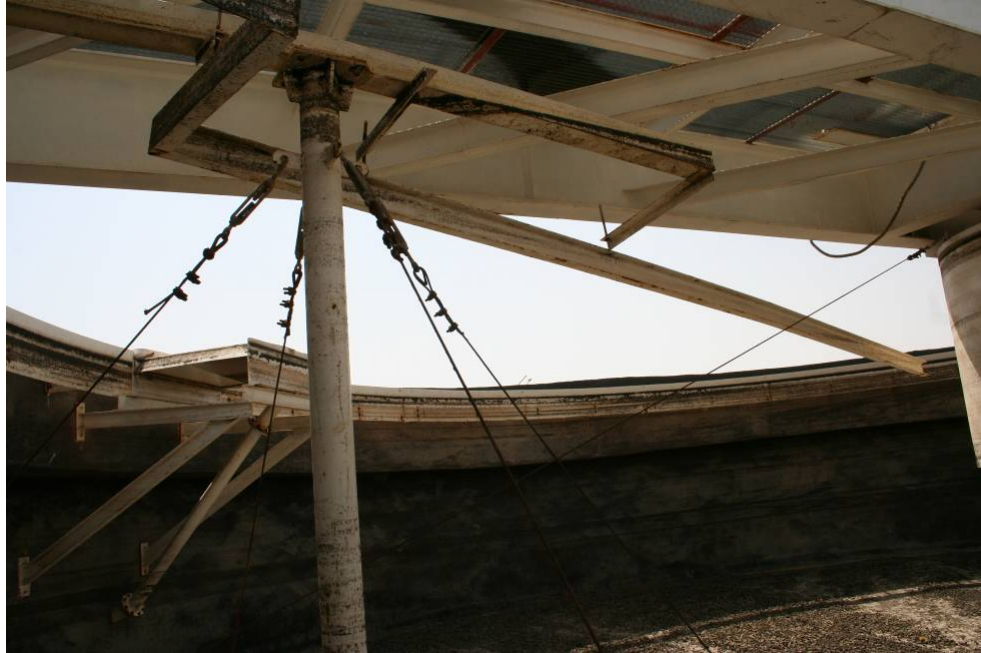
Site Photo 7. Skimmer structure viewed from inside the tank.
