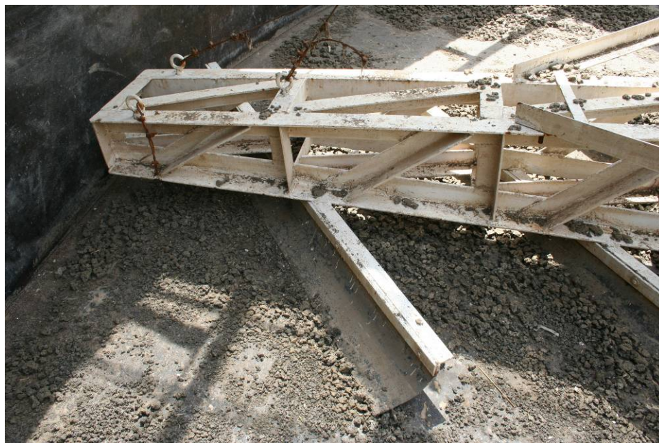
Site Photos 8. Rubber scrapers contact the floor on side that experienced cable failure.
