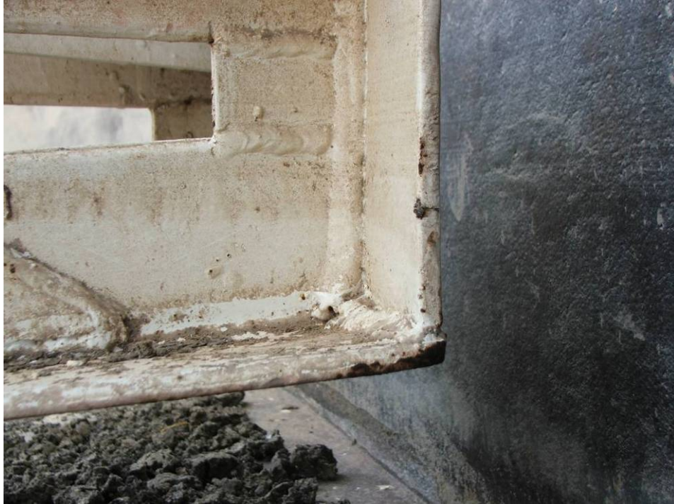
Site Photo 4. Sweep arm contact point.
