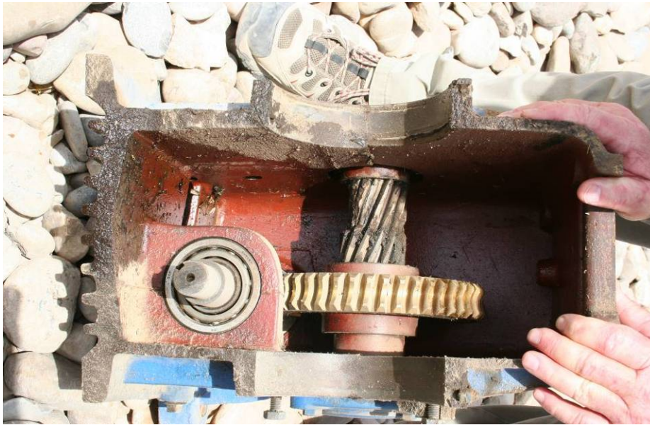
Site Photo 10. "Chewed/sheared" gear teeth and a fractured gearbox case illustrate that abnormal force broke the gear box.
