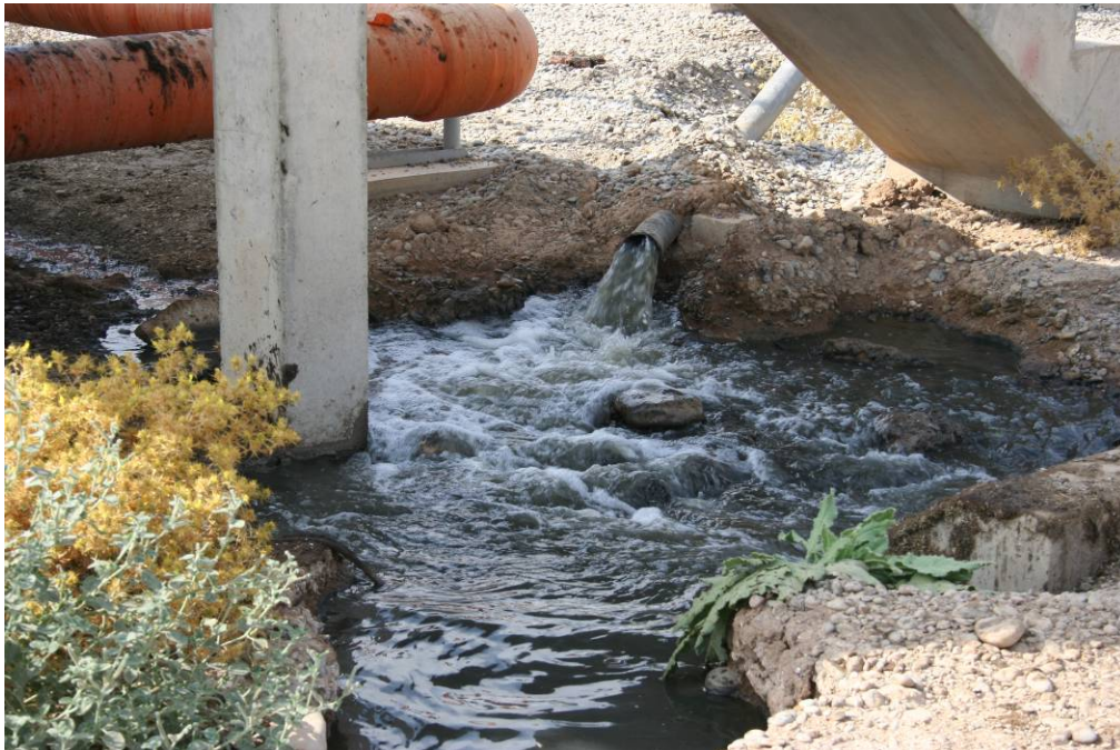
Site Photo 23. Raw sewage pumped off site via surface ditch.
