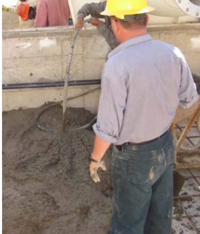
QA Photo 7. Supervisor watched worker consolidate concrete with a hand held mechanical vibrator 4 (from QA Report 26 Oct 2005).
