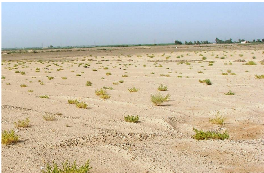
Site Photo 4. Surface of the drainage layer
