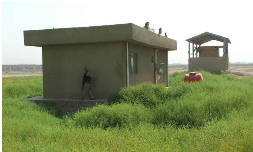
Site Photo 16. Administration building (truck maintenance building to the right)
