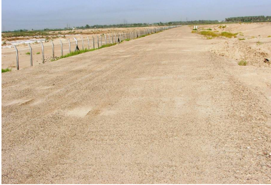
Site Photo 10. Perimeter road along the MSW landfill cell
