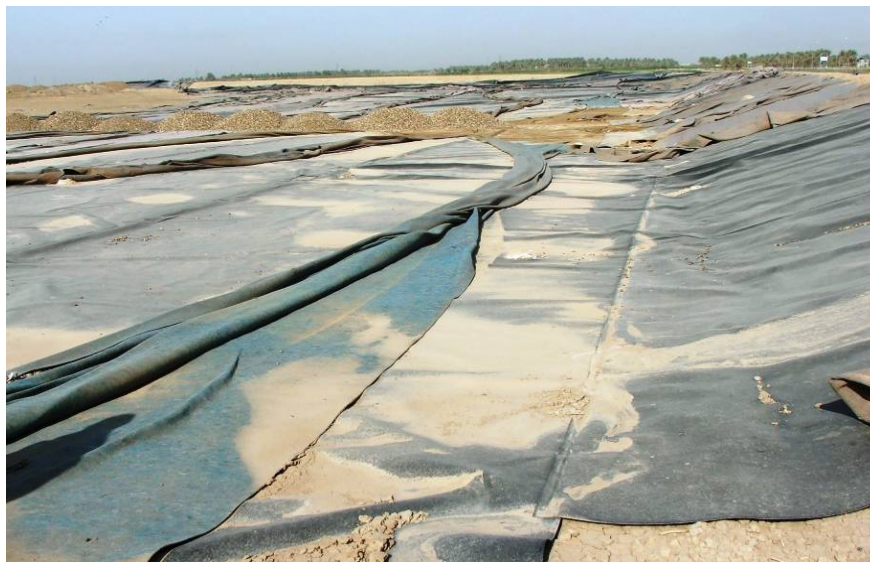
Site Photo 1. Geotextile protective liner covering
