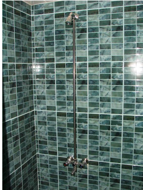
Site Photo 3. Renovated patient bathroom shower assembly
