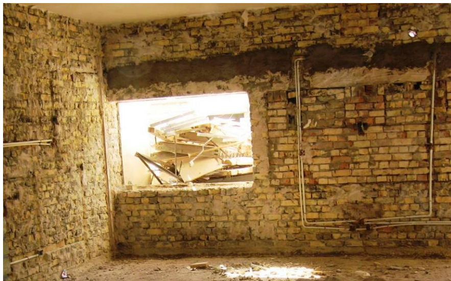
Site Photo 8. Patient ward in building B9 after demolition
