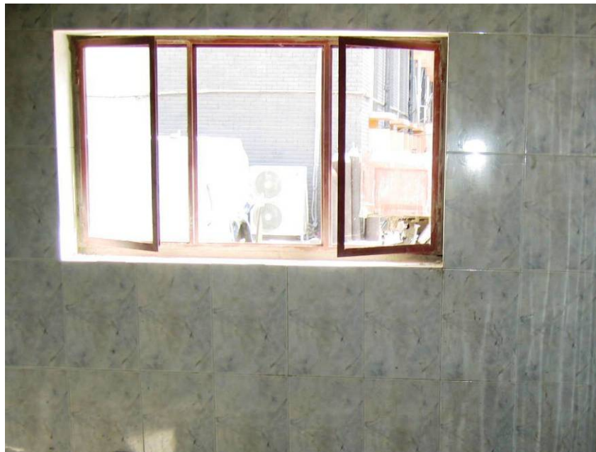
Site Photo 10. Ceramic tile installation in kitchen and laundry building (B2)
