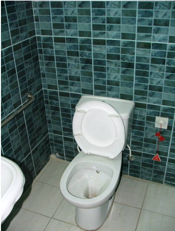
Site Photo 2. Renovated patient bathroom with western toilet
