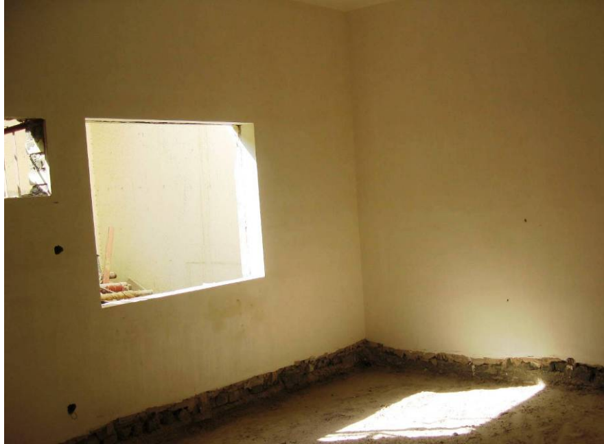
Site Photo 9. Patient ward in building B9 after plastering and painting
