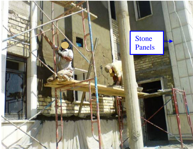
Site Photo 4. Plastering exterior wall between windows (Photo provided by USACE)
