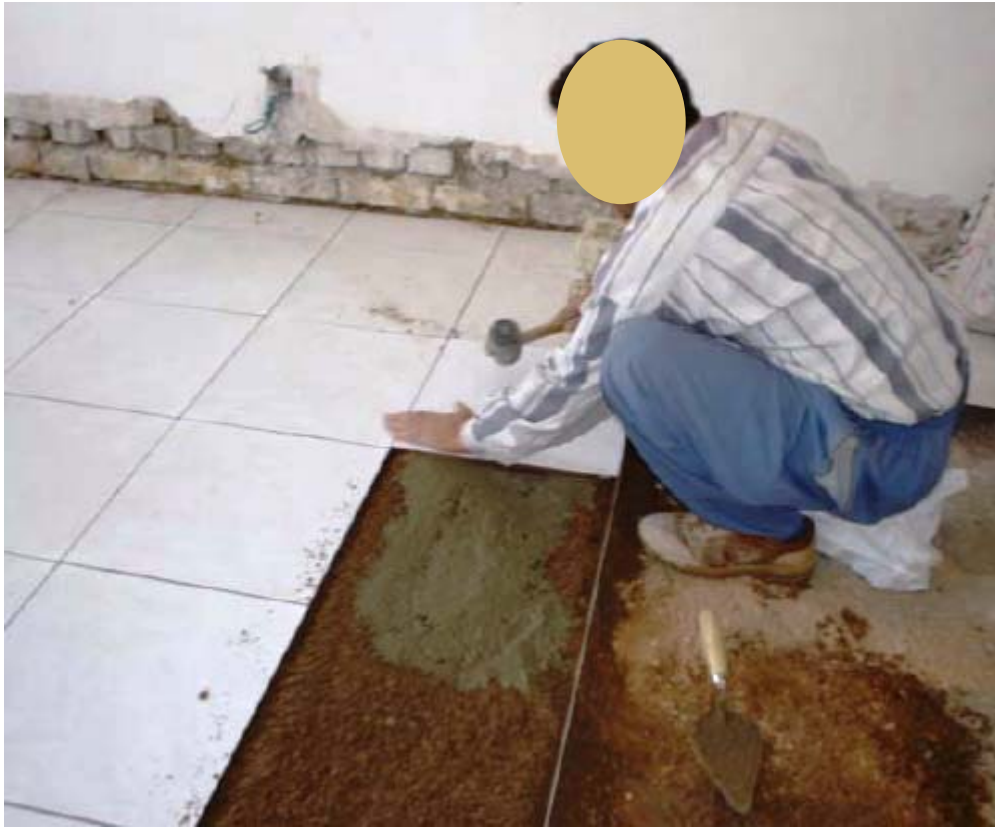
Site Photo 7. Laying ceramic tile (Photo provided by USACE)
