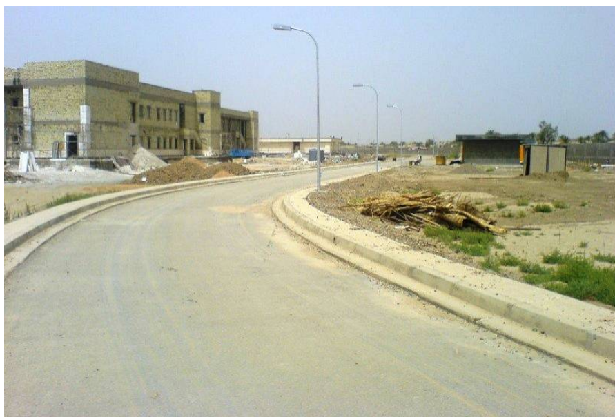
Site Photo 19. Asphalt concrete base course with concrete curb and gutter (Photo provided by USACE).
