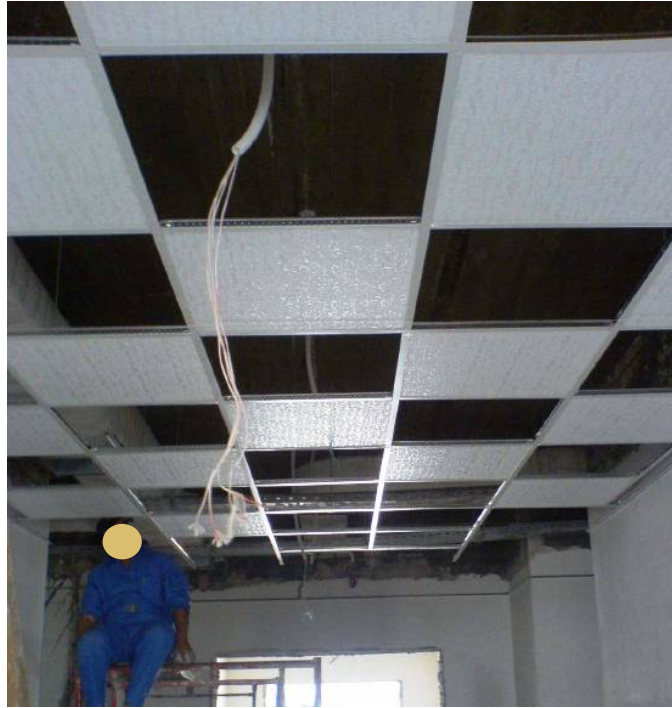
Site Photo 8. Suspended ceiling and tile installation (Photo provided by USACE)
