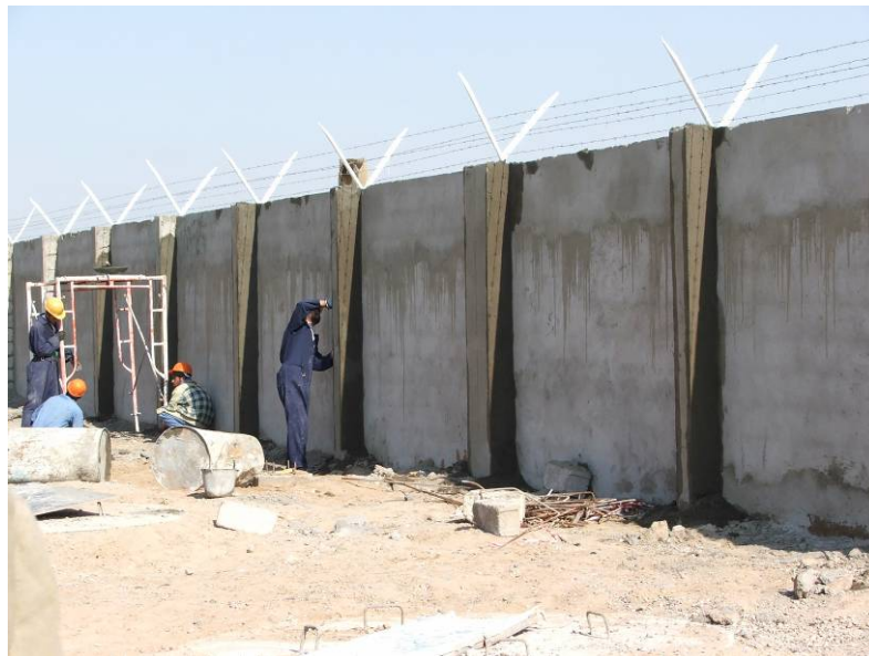
Site Photo 7: Finishing work of section of perimeter wall
