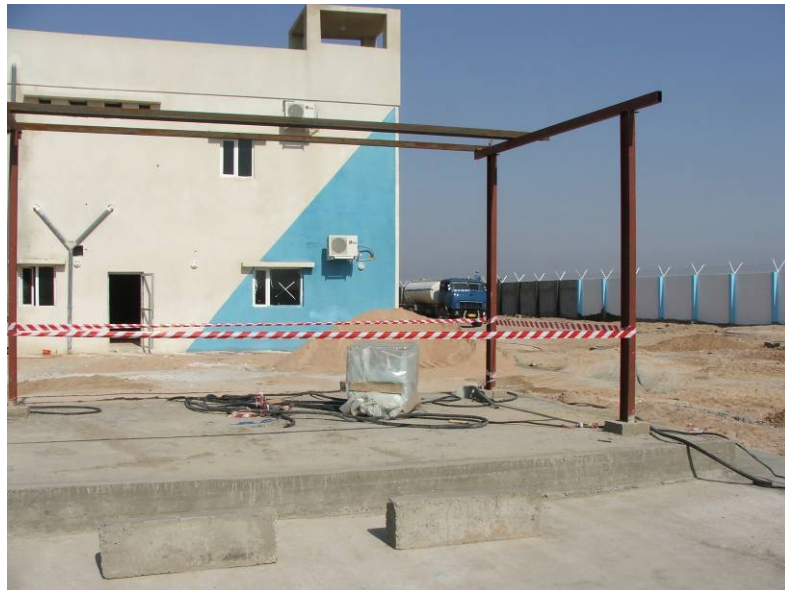
Site Photo 17: Concrete pad for generator unit
