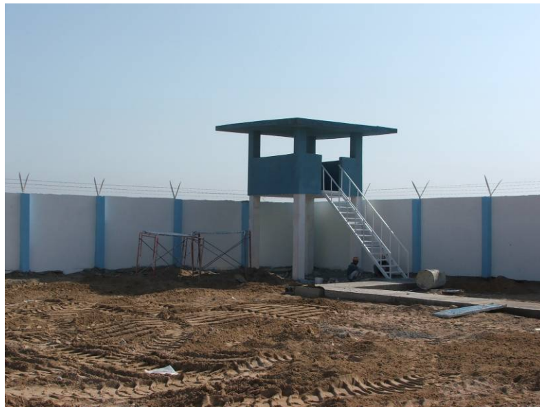
Site Photo 11: Exterior view of corner guard tower
