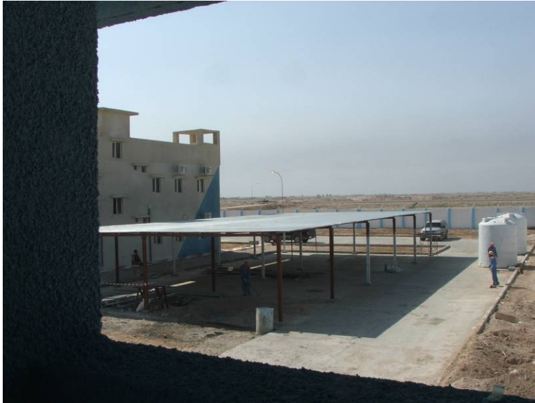
Site Photo 19: Covered parking area
