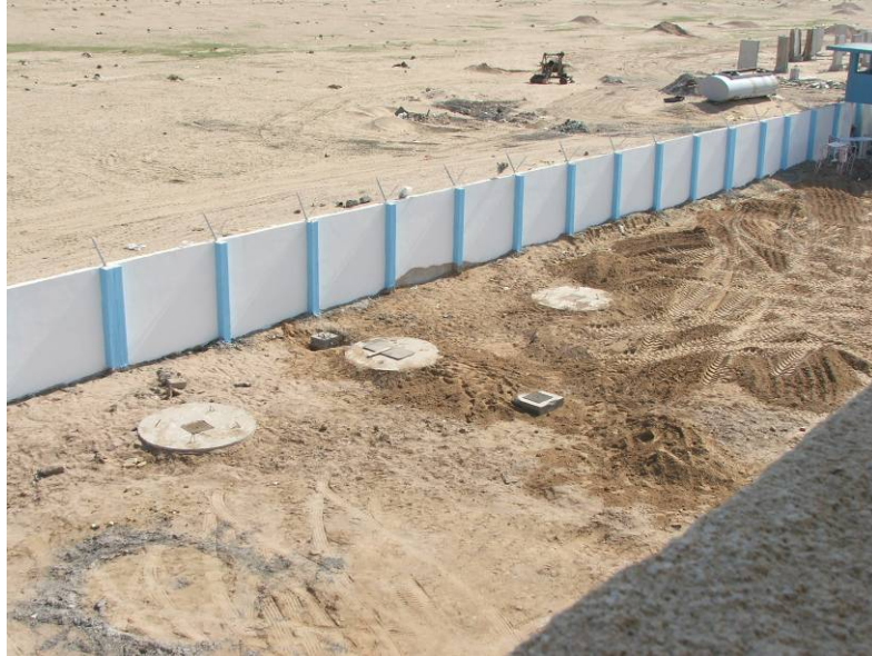
Site Photo 6: Completed section of perimeter wall
