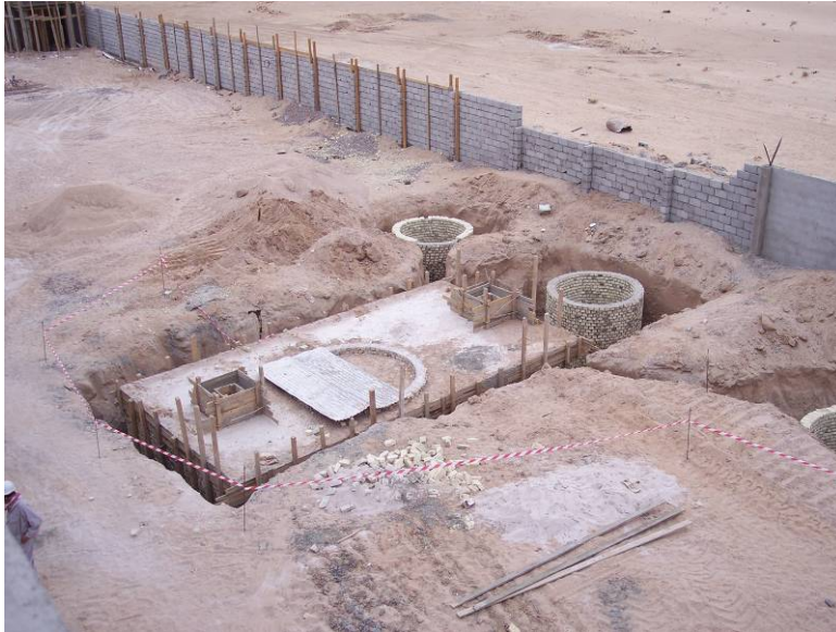
Site Photo 16: Septic system during installation (Courtesy of USACE)
