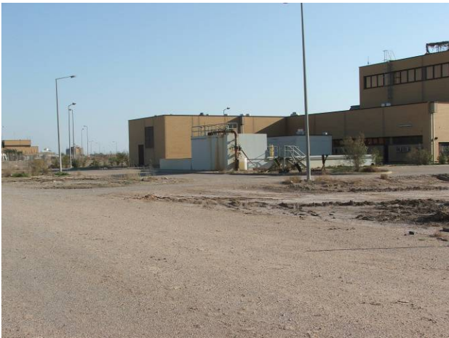
Site Photo 3. Exterior view of water treatment facility
