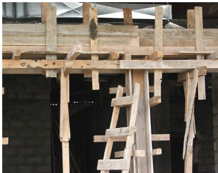
Site Photo 78. Example of remaining formwork
