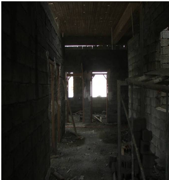
Site Photo 59. Doorframes partially completed
