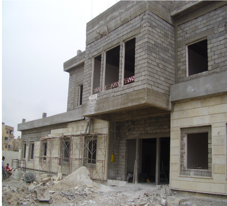
Site Photo 41. View of outside of Shiqaq Hai Musalla PHC
