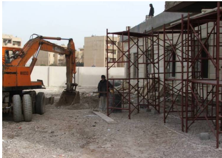
Site Photo 42. Beginning excavation of the septic tank
