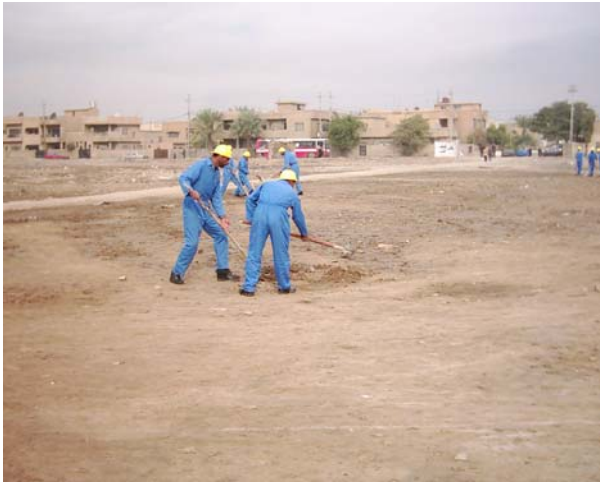
Site Photo 14. View of construction site (Photo courtesy of USACE)
