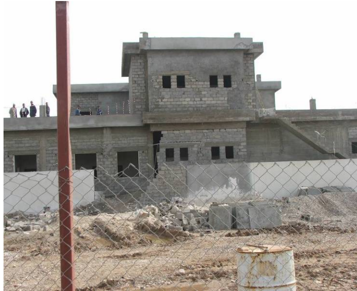
Site Photo 29. View of outside of Hai Alhajaj PHC
