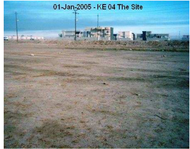
Site Photo 15. View of construction site (Photo courtesy of USACE)
