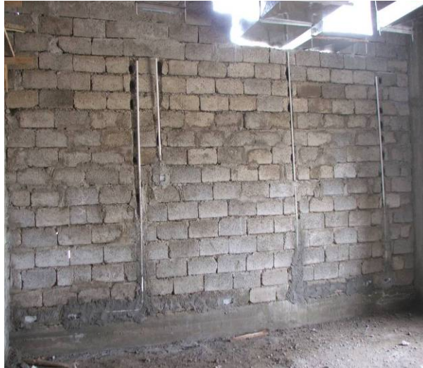
Site Photo 81. PVC conduits attached to brick wall
