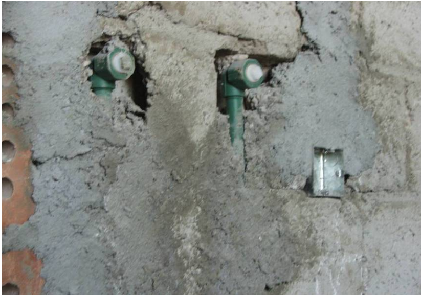
Site Photo 37. Plumbing pipes placed in block wall
