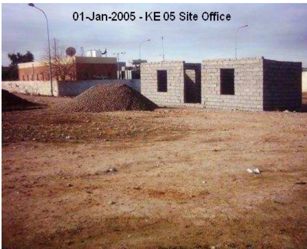
Site Photo 16. View of construction site (Photo courtesy of USACE)
