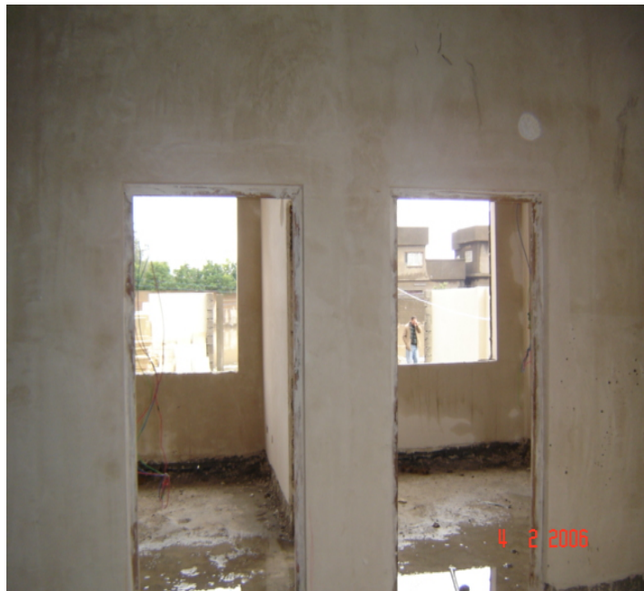
Site Photo 73. View of completed doorframes (Photo courtesy of the USACE)
