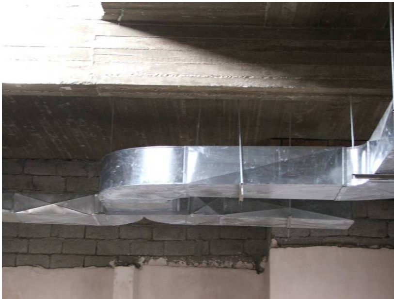
Site Photo 35. Installation of ventilation ductwork
