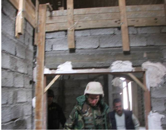
Site Photo 52. View of remaining formwork
