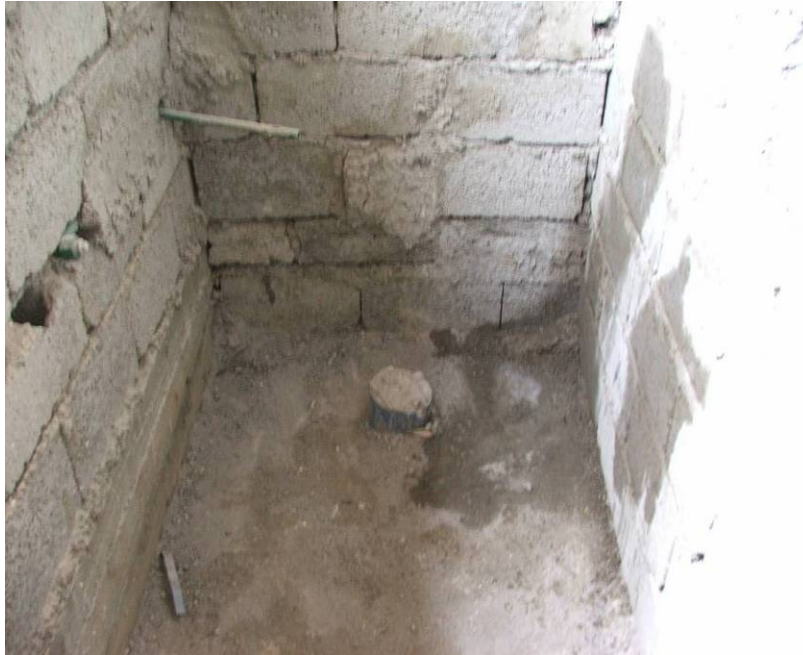
Site Photo 72. Plumbing pipes placed in concrete slab
