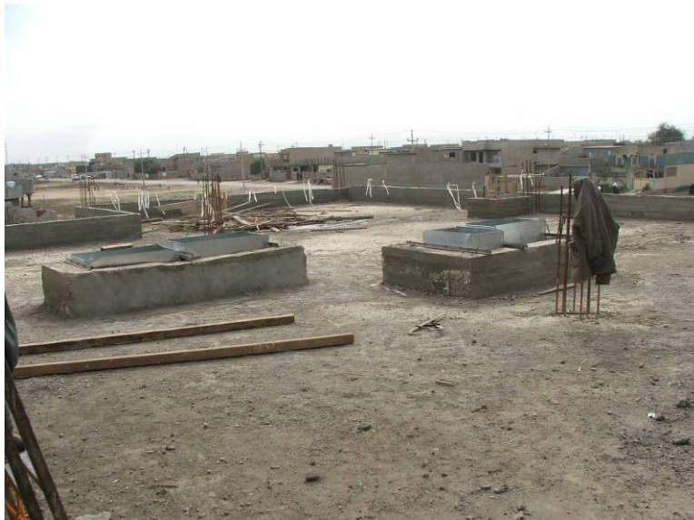
Site Photo 80. Condition of the roof
