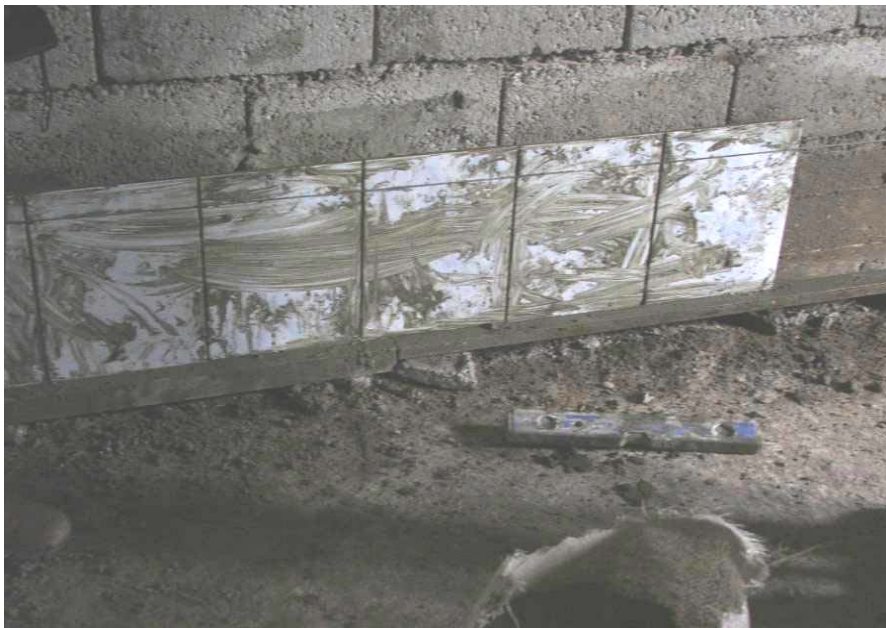
Site Photo 50. Example of tile work
