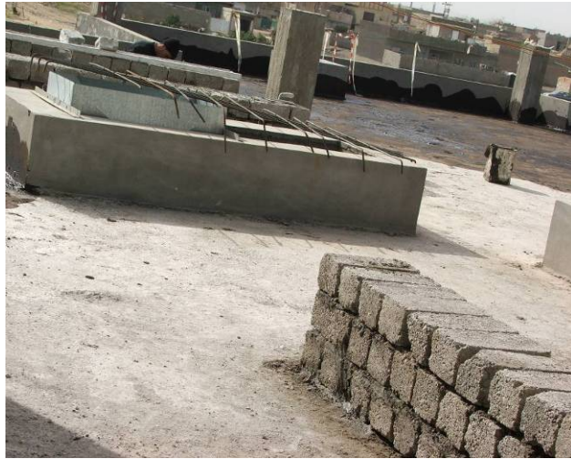
Site Photo 33. Roof partially covered with tar
