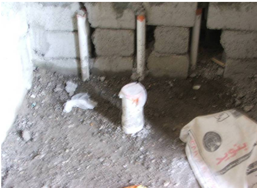
Site Photo 38. Plumbing pipes placed in concrete slab
