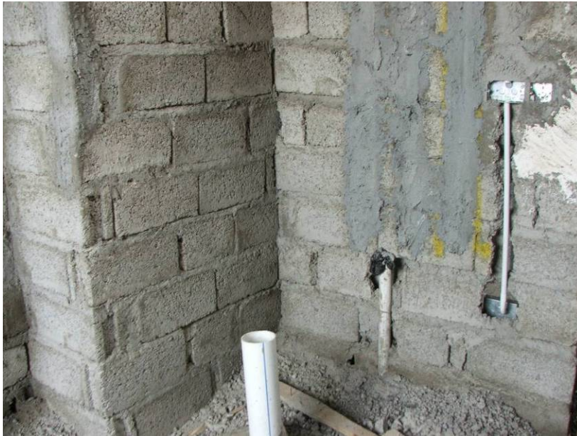
Site Photo 58. Plumbing pipes placed in concrete slab
