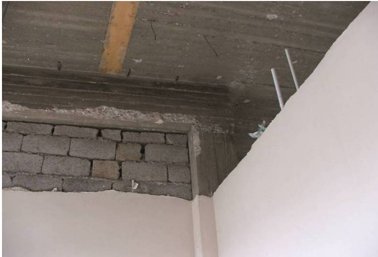
Site Photo 1. Load-bearing ceiling beam (PHC Hai Alasra Wa Al Mafqoodeen)
