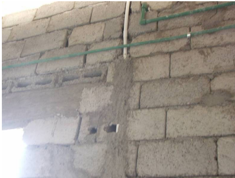
Site Photo 70. Plumbing lines installed across block wall
