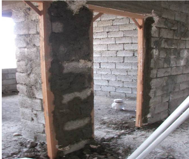
Site Photo 85. Partially installed doorframe
