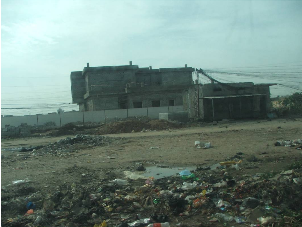
Site Photo 26. “Windshield survey” of the Hai Alhajjaj PHC
