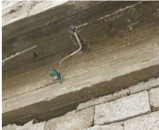
Site Photo 44. PVC conduit installed in structural concrete
