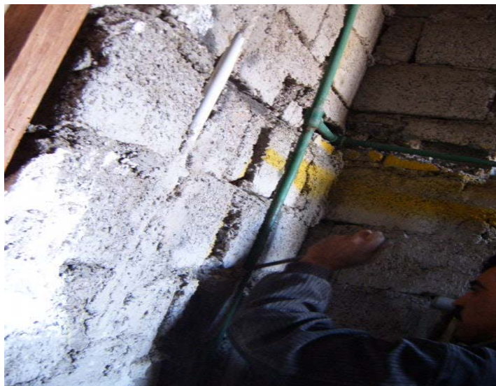
Site Photo 84. Installation of plumbing pipes into blocks
