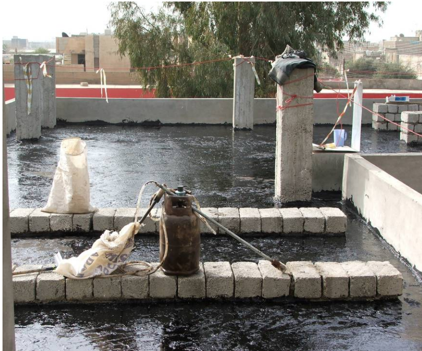
Site Photo 43. Tar applied to the roof
