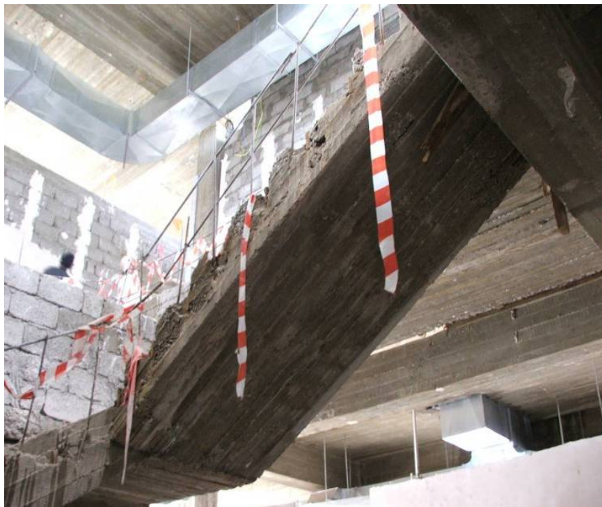
Site Photo 11. View of stairwell (PHC Hai Al Wasily)
