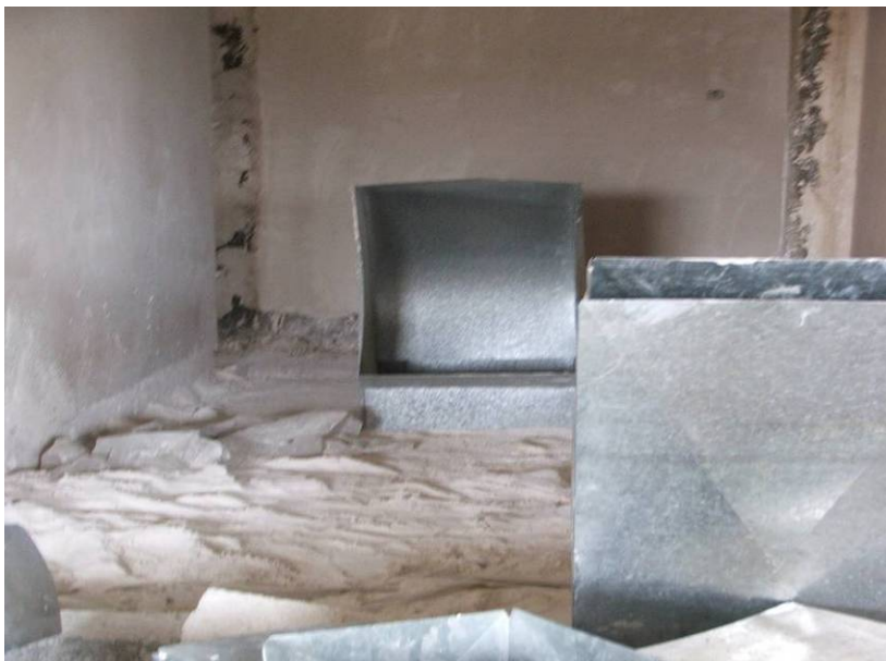
Site Photo 36. Additional pieces of ventilation ductwork to be installed
