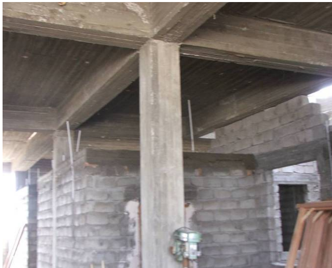
Site Photo 53. First floor structural beams
