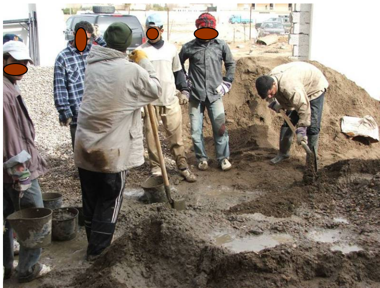
Site Photo 57. Concrete mixing
