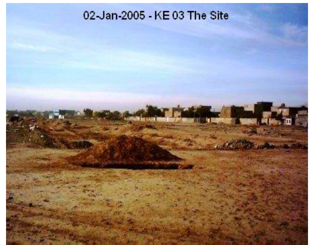
Site Photo 17. View of construction site (Photo courtesy of USACE)
