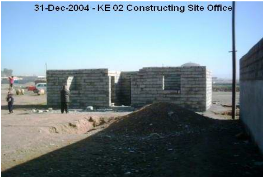
Site Photo 13. View of construction site (Photo courtesy of USACE)
