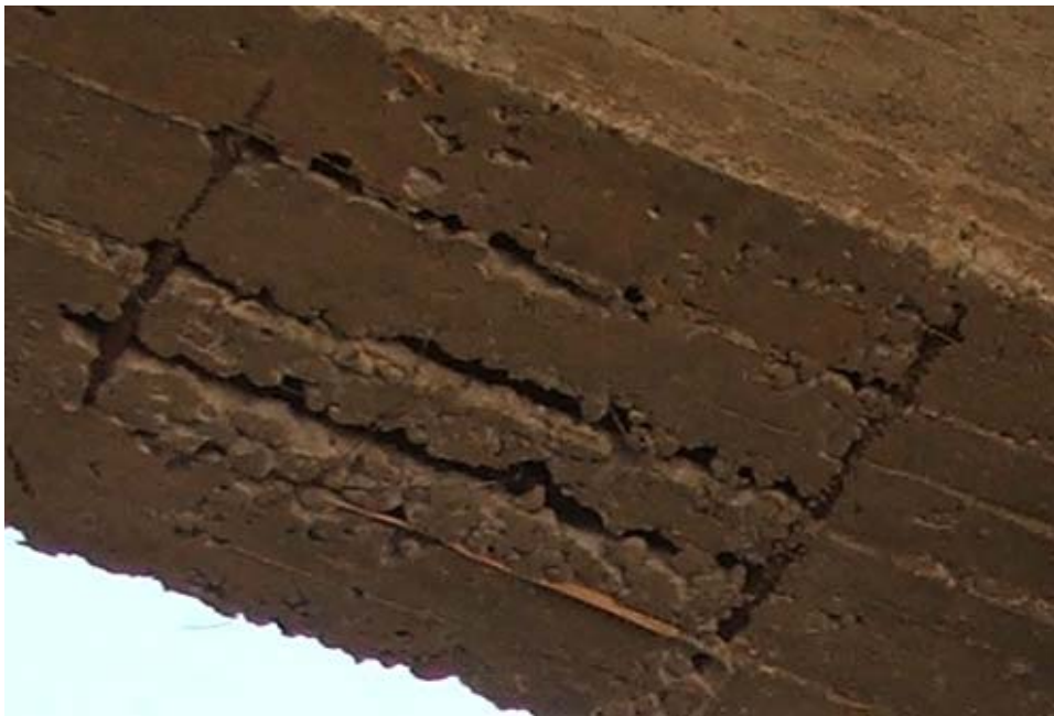
Site Photo 27. Close-up view of concrete first floor ceiling concrete beam
