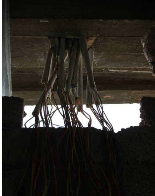
Site Photo 67. Electrical wire running through PVC conduit
