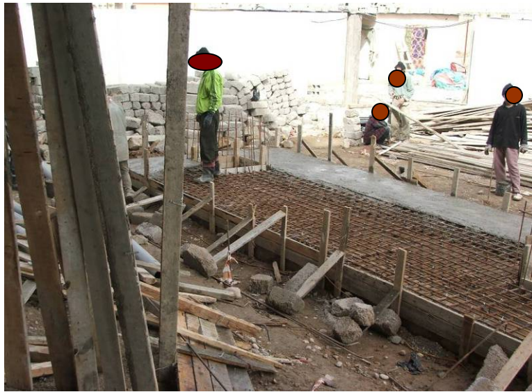
Site Photo 56. Workers applying rebar to top of septic tank
