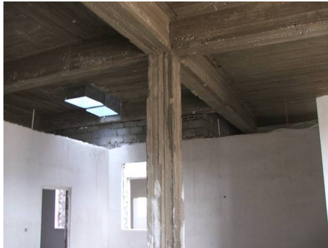
Site Photo 31. First floor structural column and beams
