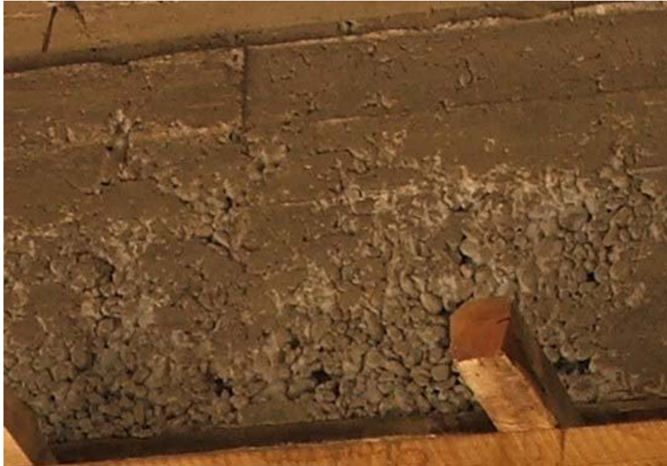
Site Photo 28. Close-up view of concrete first floor ceiling concrete beam
