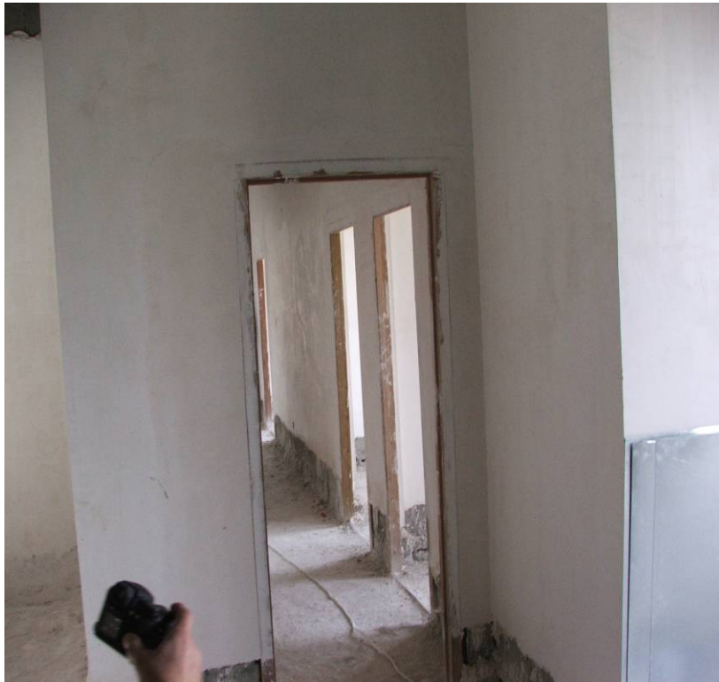
Site Photo 48. Example of completed doorframes
