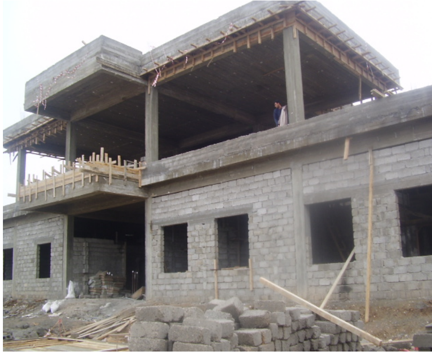
Site Photo 51. View of outside of Hai Tis'een PHC
