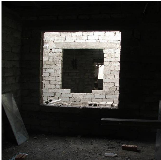
Site Photo 86. Windows without frames
