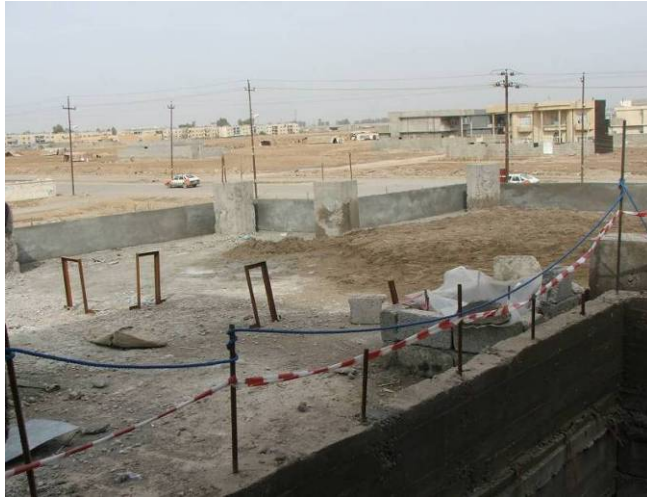
Site Photo 66. Roof in need of cleanup prior to tarring
