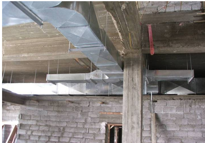
Site Photo 77. First floor structural beams and column
