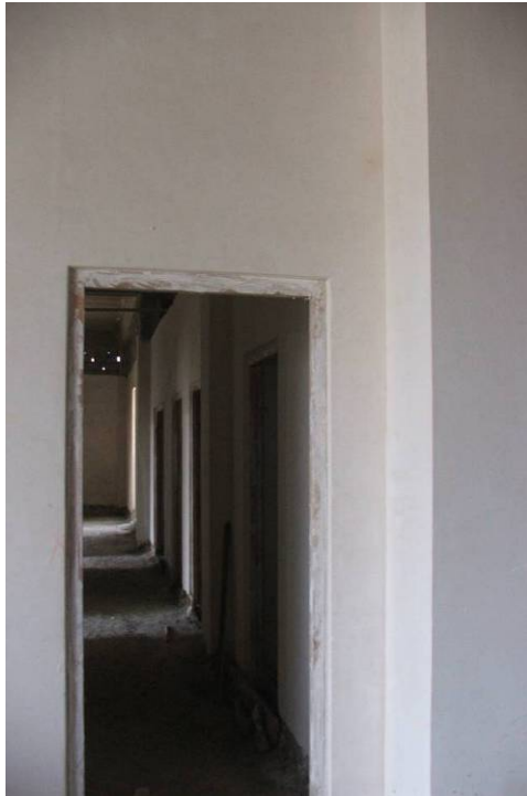
Site Photo 39. Example of completed doorframes
