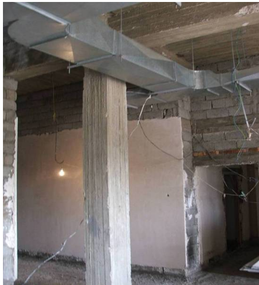
Site Photo 64. First floor structural column and beams
