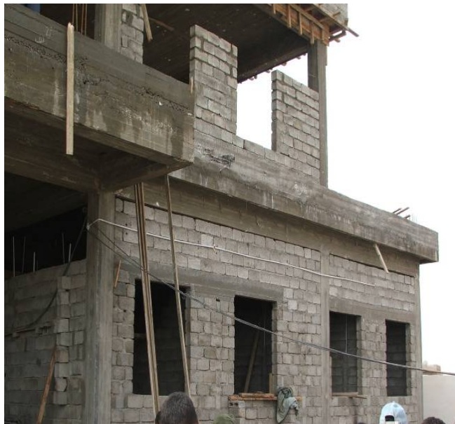
Site Photo 61. Window frames
