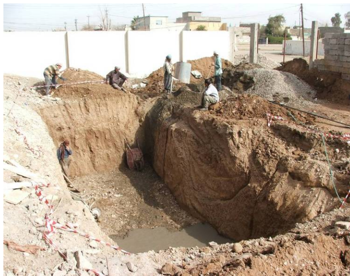
Site Photo 30. Excavated hole for septic tank
