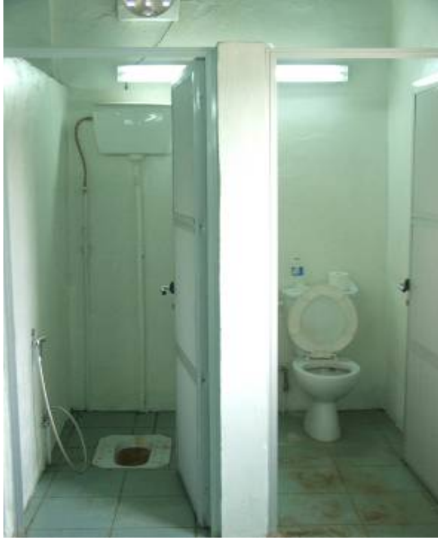
Site Photo 22. Restroom with eastern (left) and western toilets
