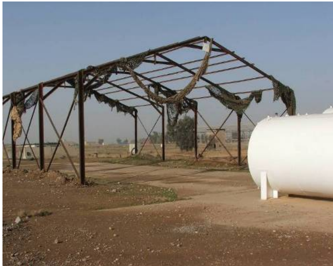
Site Photo 34. Future cover of both fuel tanks
