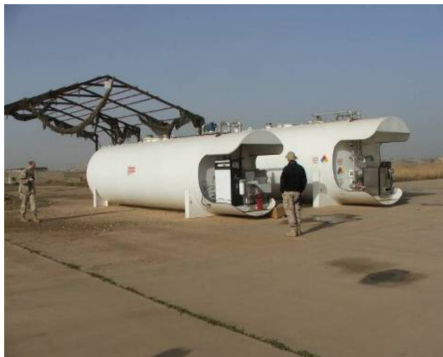
Site Photo 32. Two fuel tanks
