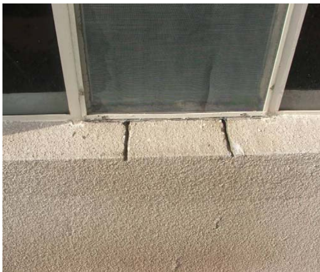
Site Photo 12. Contractor's fix for window drainage (drain lines)
