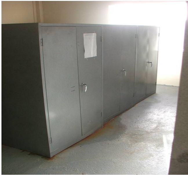
Site Photo 11. Leaking water on classroom floor
