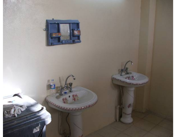
Site Photo 8. Sinks in the bathroom
