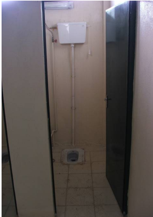
Site Photo 7. Eastern toilet in bathroom
