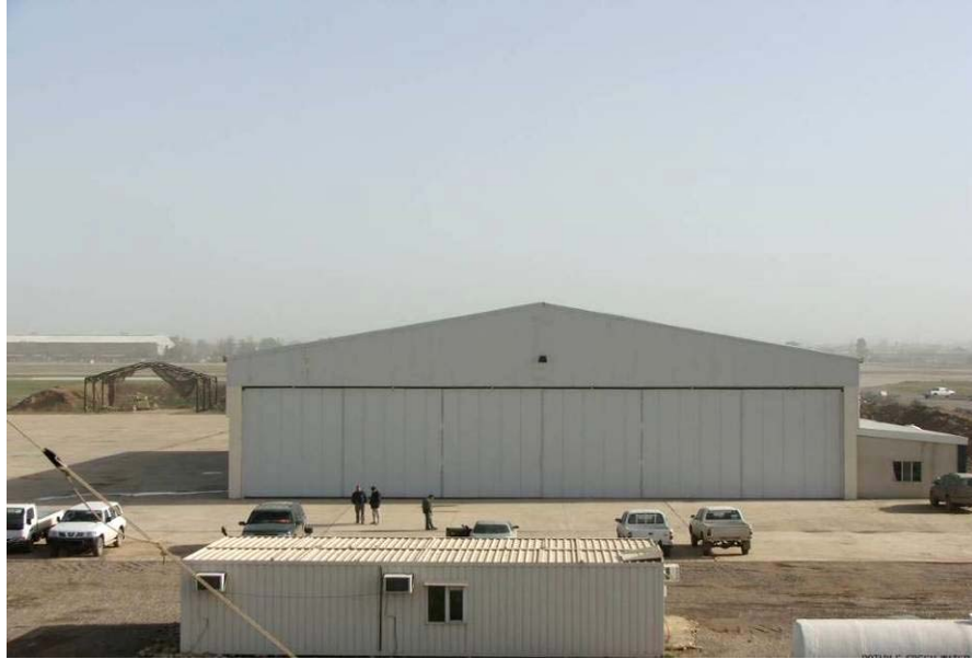
Site Photo 2. Exterior view of the hangar
