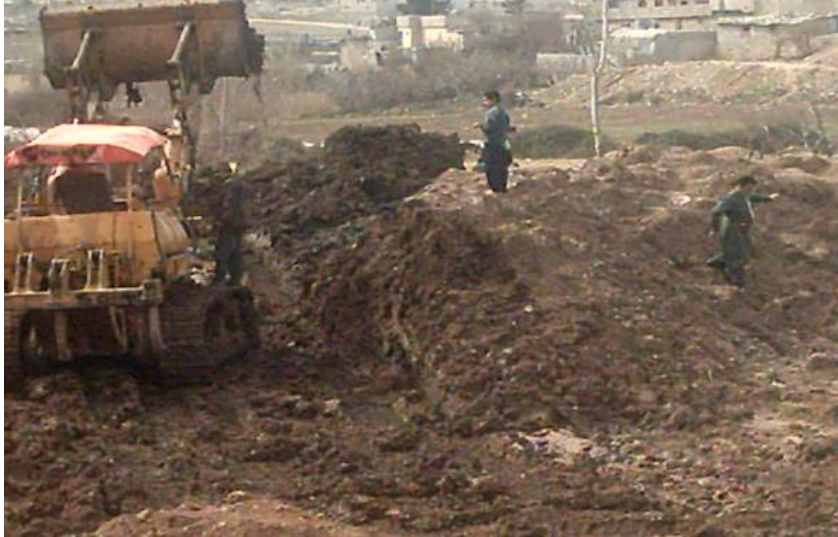
Site Photo 1. Initial site preparation work – Photo provided by USACE
