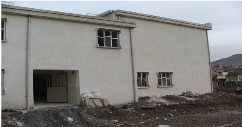
Site Photo 7. Exterior showing painted cement finish
