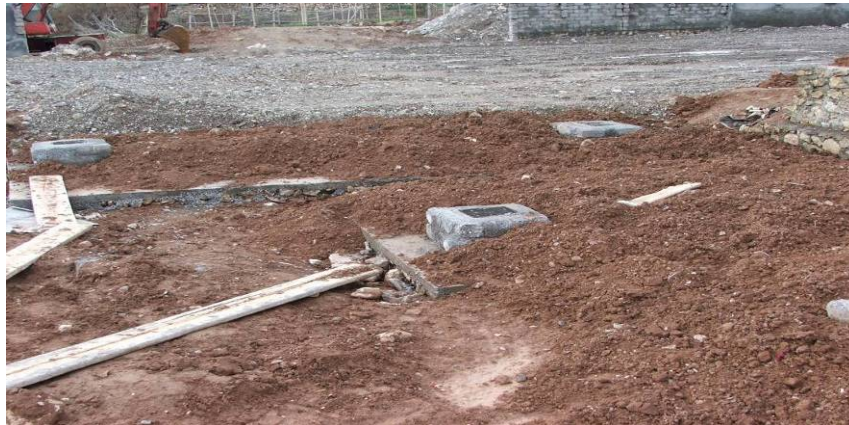
Site Photo 14. Septic tank location and manholes in front of school
