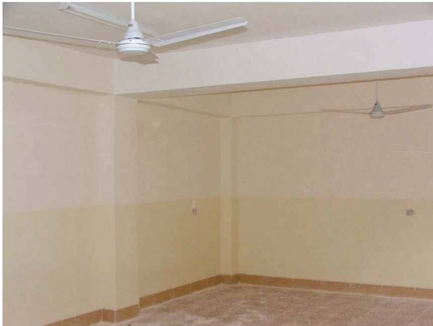
Site Photo 6. Ceiling fan installation
