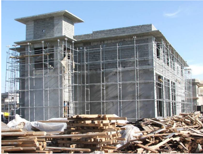
Site Photo 2. Exterior view of the Ainkawa fire station
