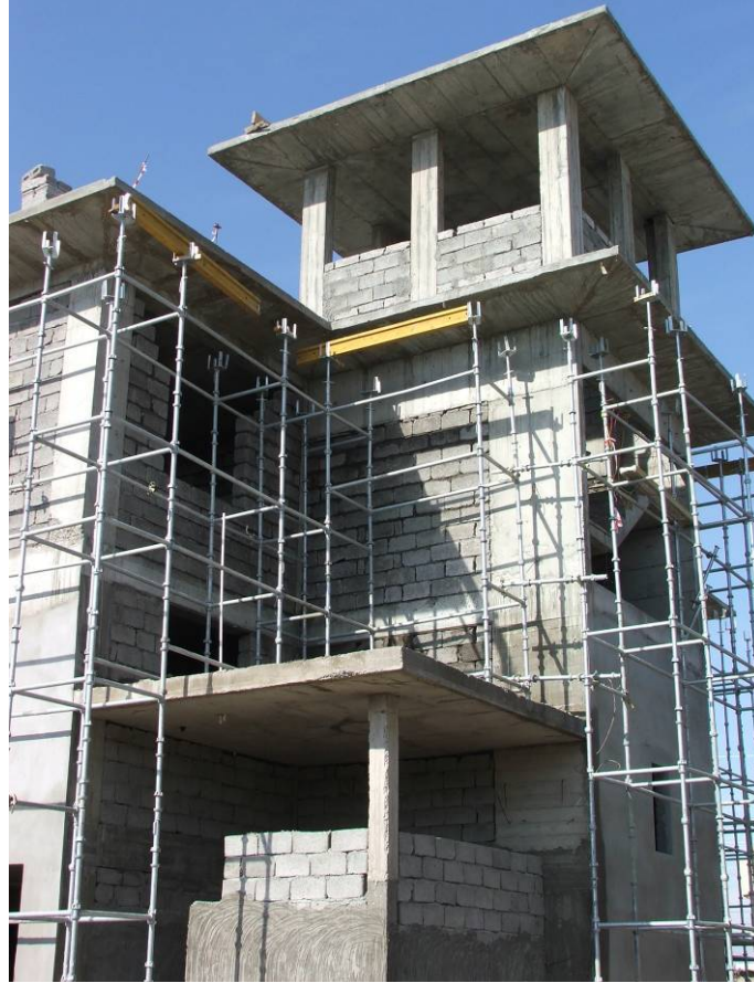
Site Photo 11. Exterior view of staircase # 1
