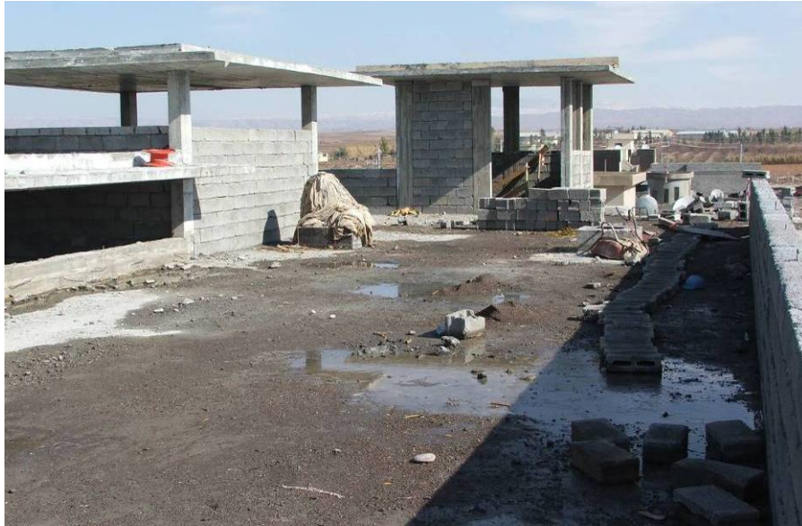
Site Photo 12. Fire station roof construction
