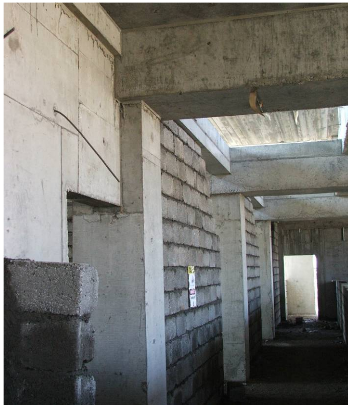
Site Photo 3: Interior structure showing concrete block walls, columns, and beams
