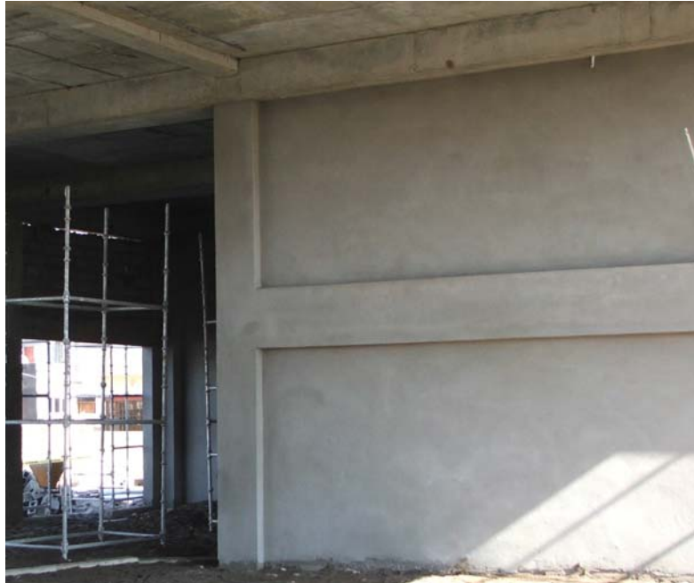
Site Photo 14. Finish coating applied to concrete surfaces on Level 1
