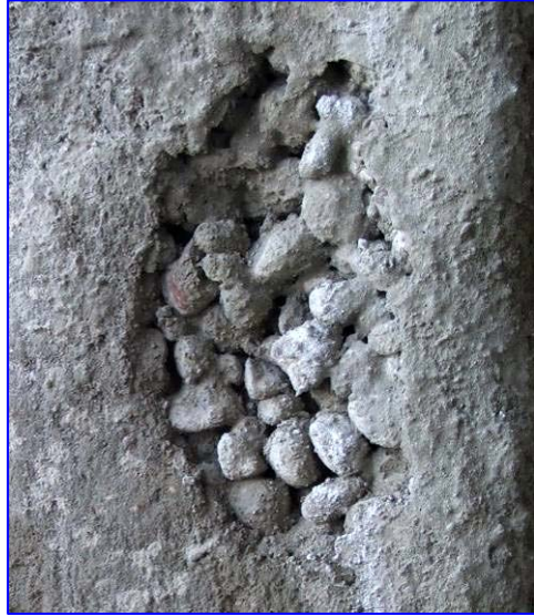
Site Photo 6. Closeup of Site Photo 5
