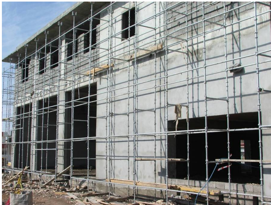
Site Photo 13. External concrete block wall construction on Level 3
