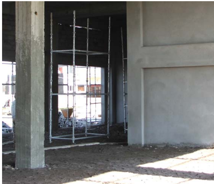
Site Photo 16. Base Preparation in Level 1 prior to floor slab construction
