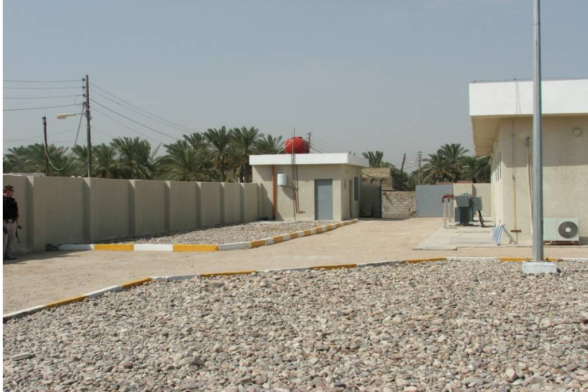
Site Photo 2: Exterior fence, guard house, and gate
