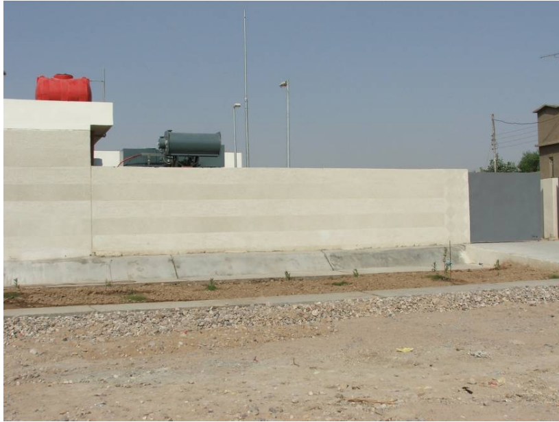
Site Photo 1: Exterior fence and gate (right)
