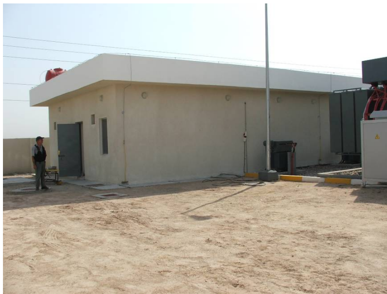
Site Photo 1: Substation building exterior view
