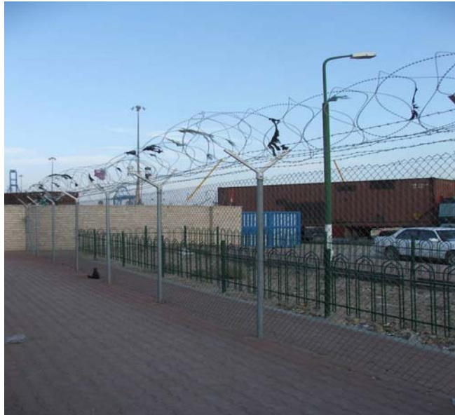
Site Photo 3. Perimeter Fence with Concertina Wire
