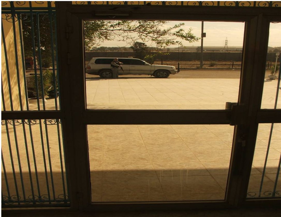
Site Photo 1. Marble Sidewalk at the Building Entrance
