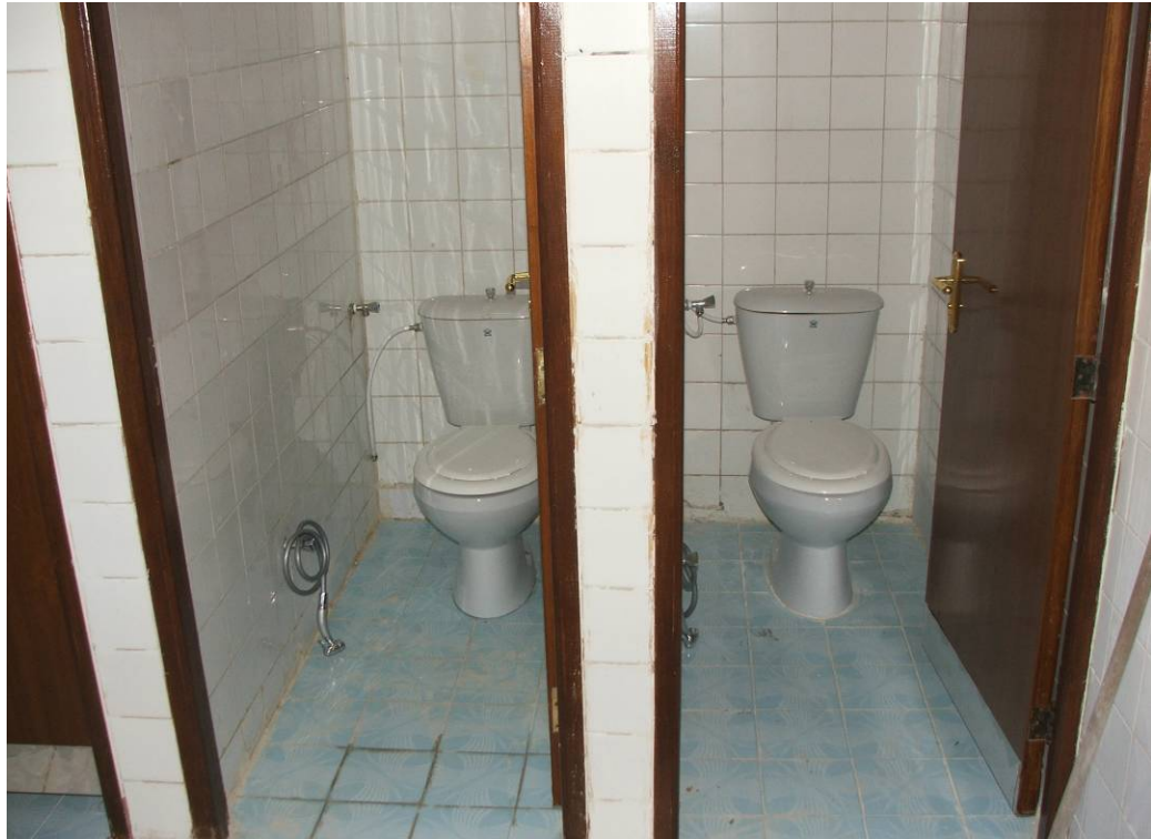
Site Photo 8. New “Western Style” Bathroom Toilets
