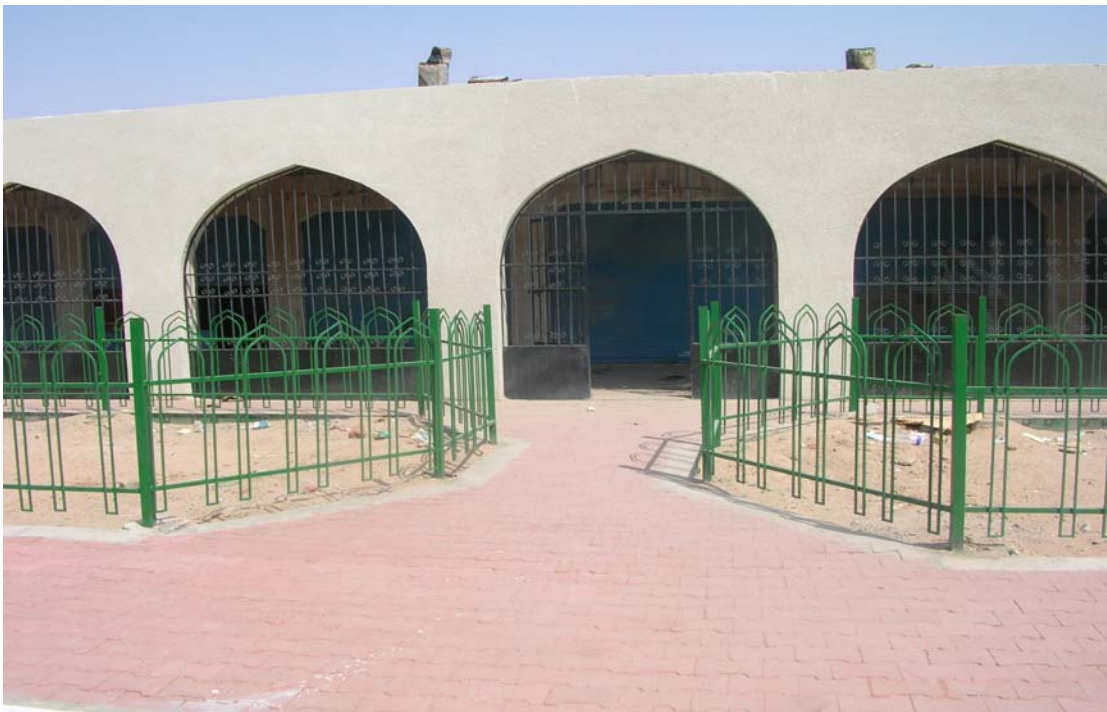
Site Photo 2. Brick Sidewalk in front of Kiosk (Photograph Courtesy of the USACE GRS Resident Engineer)
