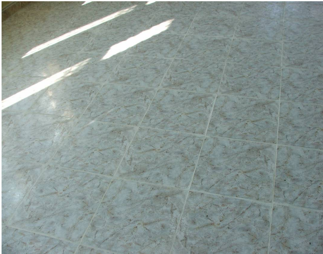
Site Photo 11. New Ceramic Tile throughout the Operations Center Building
