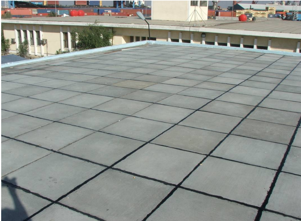
Site Photo 5. Section of the Roof
