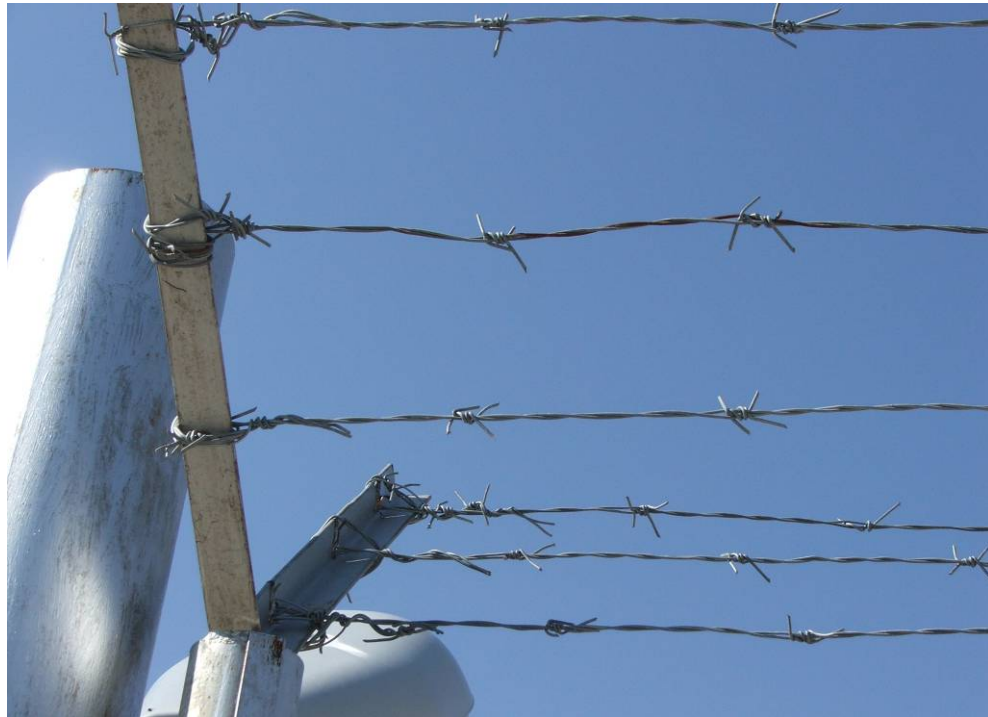
Site Photo 2. Barbed Wire Outriggers on Security Fence
