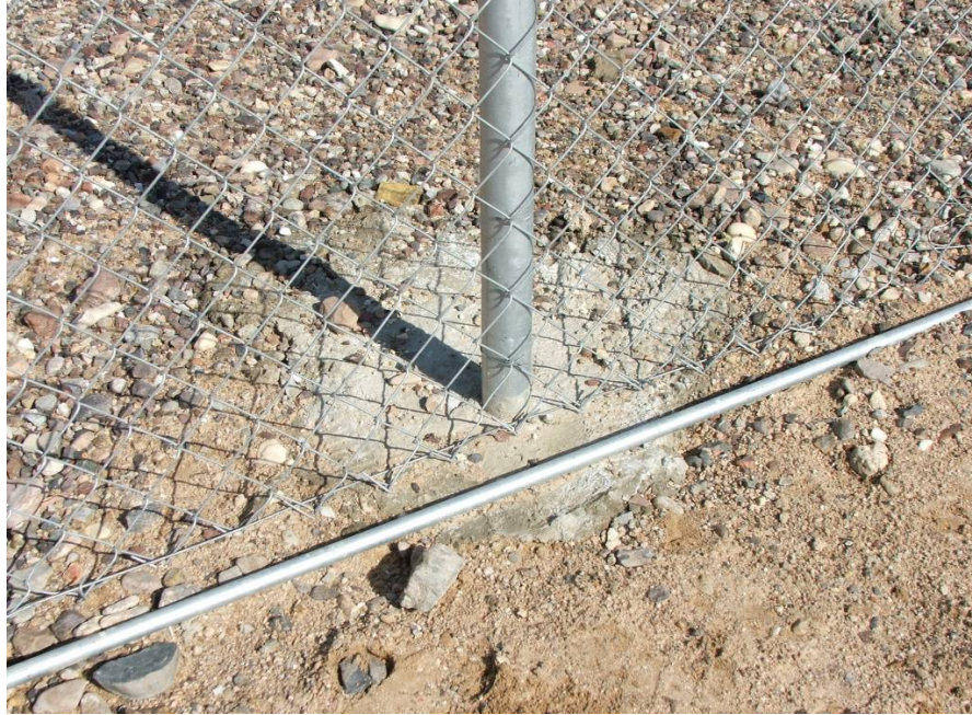
Site Photo 3. Security Fence Pole Anchored into Ground with Concrete
