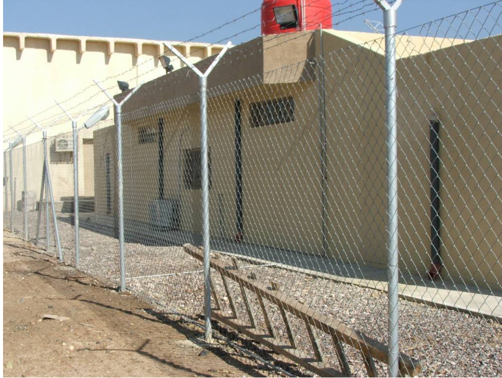
Site Photo 5. Three Roof Mounted Lights on the Rear of the ASP
