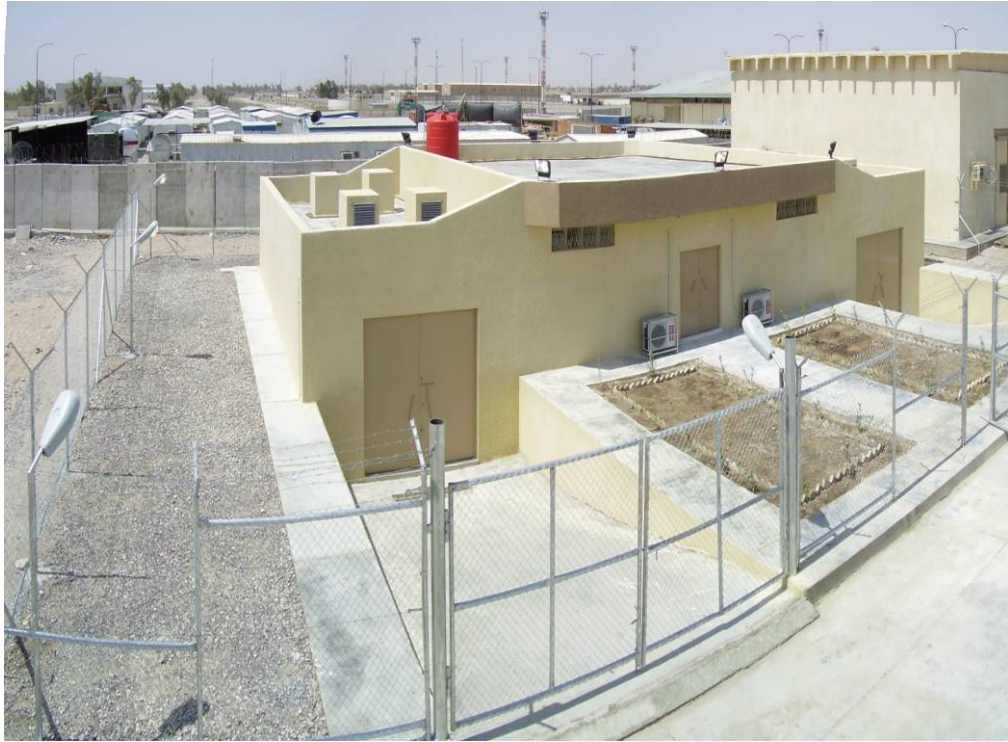
Site Photo 1. View of Security Fence around the ASP (Photograph Courtesy of USACE Resident Engineer)
